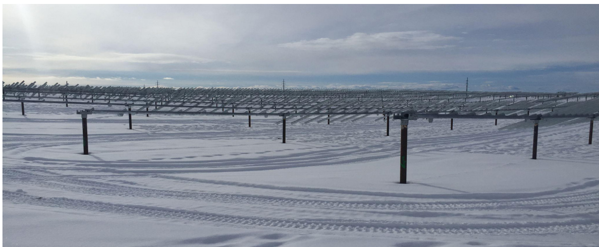
FIGURE 26: Solar framing at another site being installed prior to mounting the panels 48
