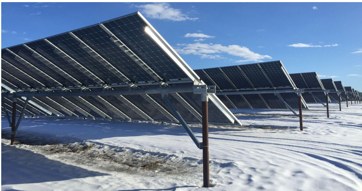
FIGURE 27: An example of fully installed south facing, bi-facial, fixed tilt solar arrays. This view from the back shows the framing typically used for this type of installation 50
