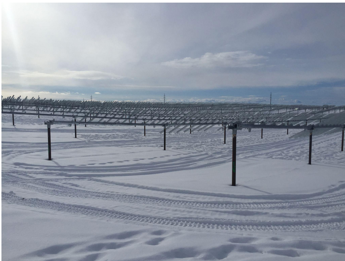
FIGURE 29: Solar framing at another site being installed prior to mounting the panels 43
