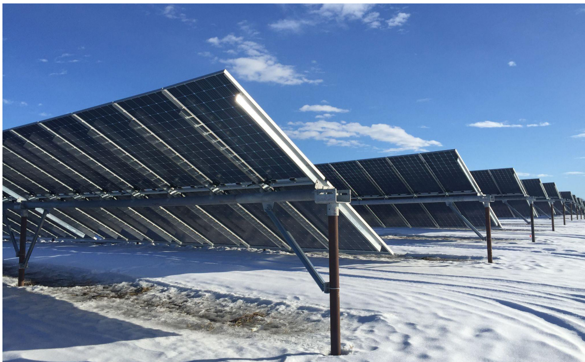
FIGURE 30: An example of fully installed south facing, bi-facial, fixed tilt solar arrays. This view from the back shows the framing typically used for these types of panels 45
