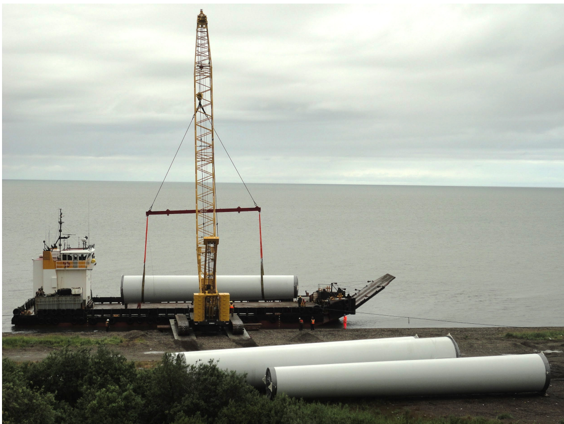
Figure 30: EWT tower sections being lifted from barge to beach using a mobile crane.
