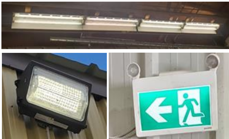
Figure 4: T12 Fluorescent (top), Exterior Wall Pack (left), and Emergency (right)
