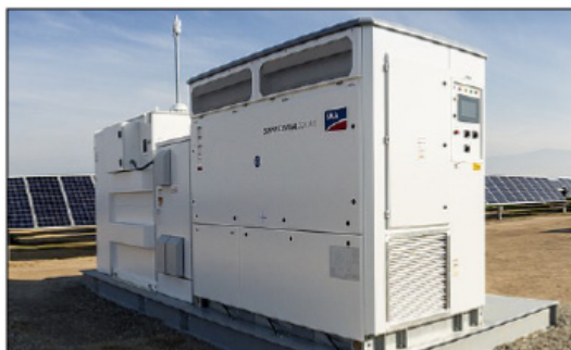
Figure 14: Inverter unit typical of a large ground-mounted solar PV array. 139
