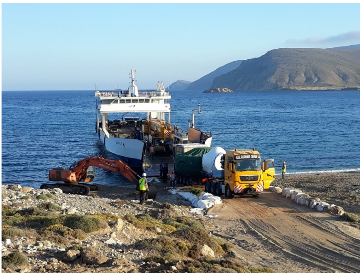
Figure 32: EWT turbine components being transported from barge to beach using a temporary ramp.
