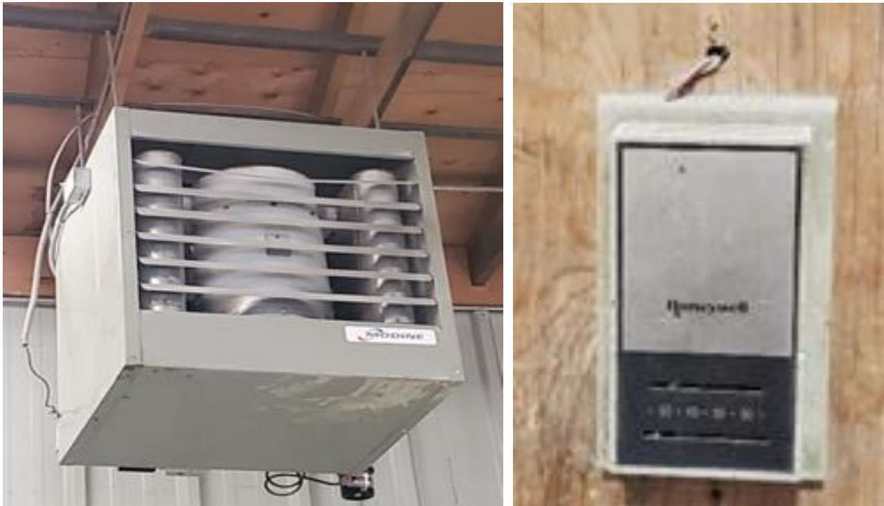
Figure 2: Modine Unit Heater (left), Honeywell Thermostat (right)
