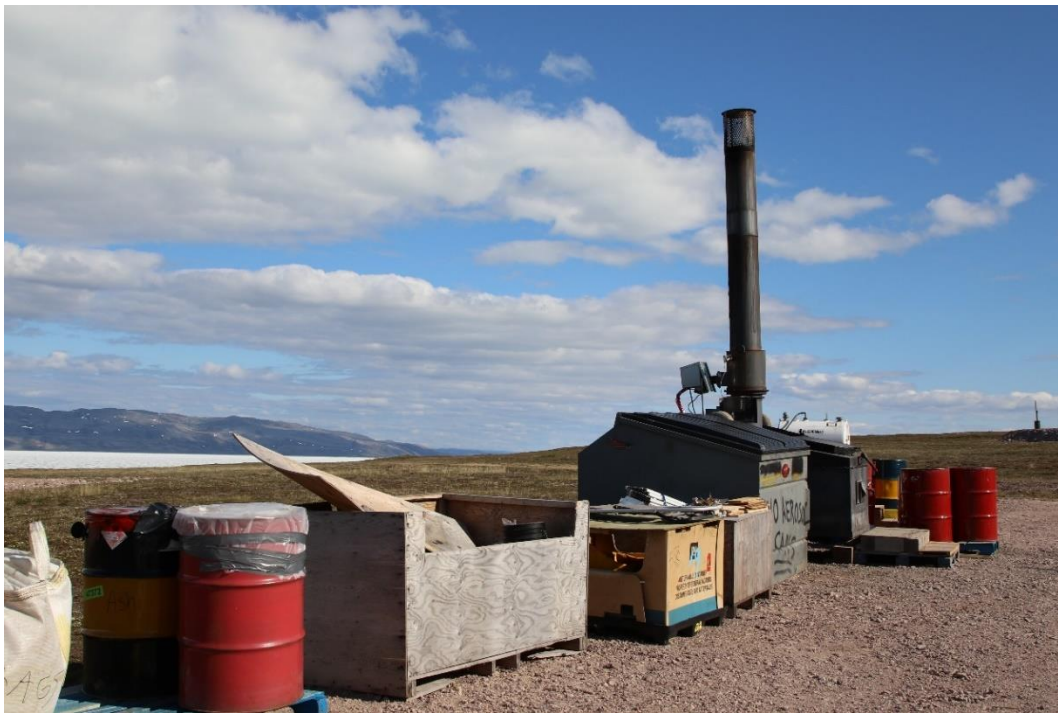
Photo 33: Incinerator with Waste Segregation
