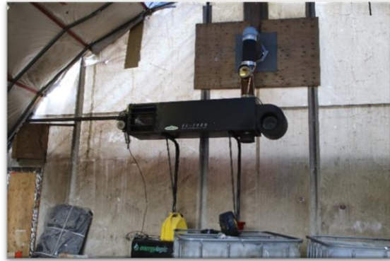
Photo 17: Oil Heater Supplied by Used Oil
