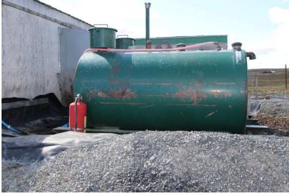
Photo 16: Heating Fuel Tank and Berm
