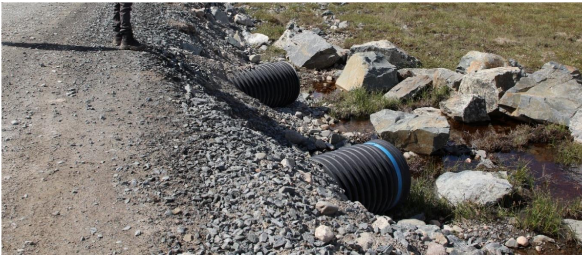
Photo 21: Culvert on the Road Towards the New Goose Camp Pad
