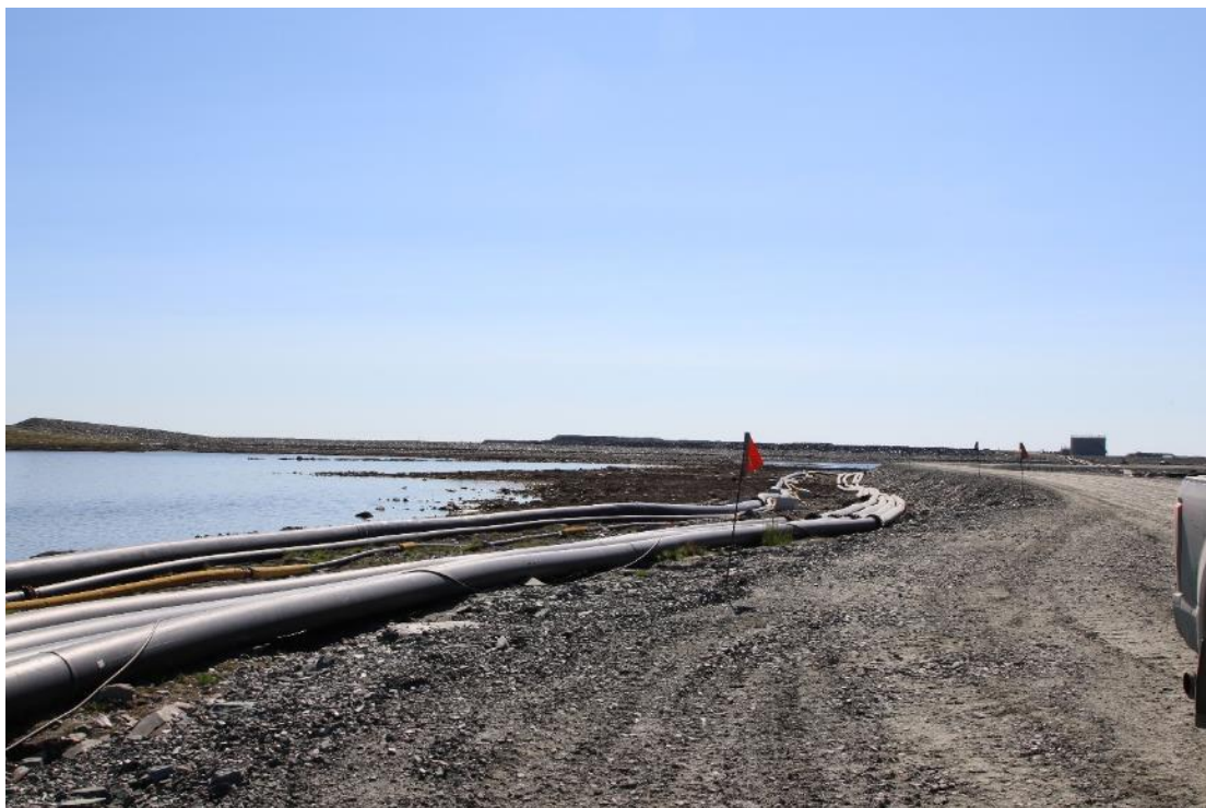
Photo 41: Waterlines for Moving Water to and from Containment Pond 1
