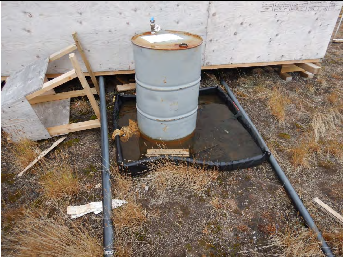
Description: secondary containment full of water.
