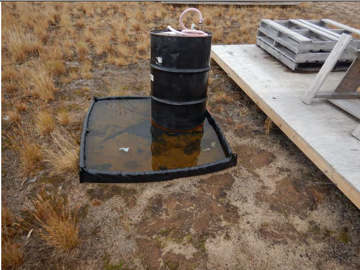
Description: secondary containment full of water.
