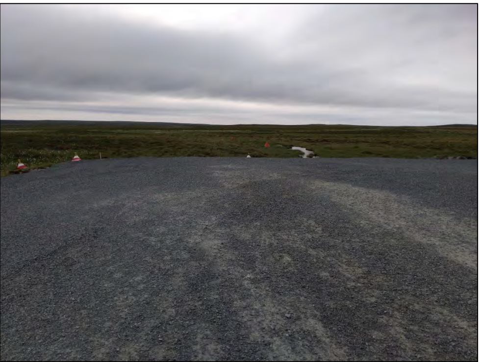
Photo 26 – Southern end of airstrip where think fill note, no cracking or undulation observed
