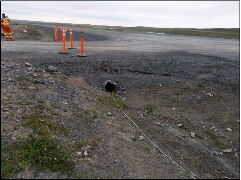
Photo 21 – Culvert along airstrip channel along northern edge
