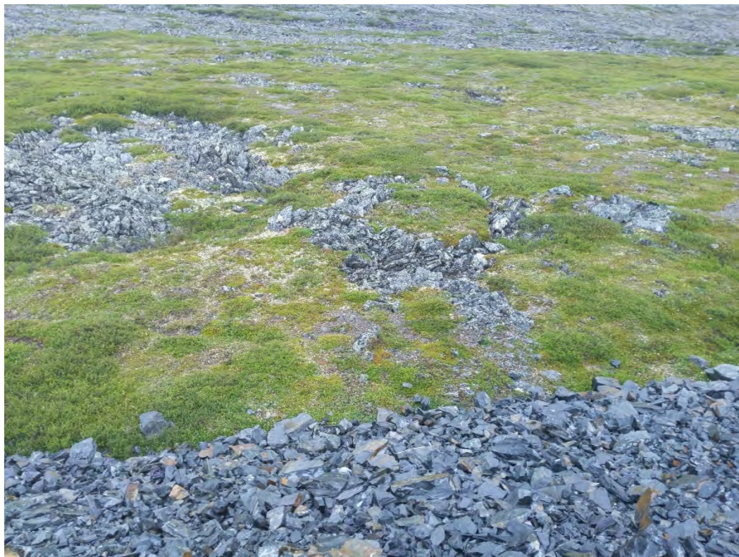
Photo 14 – Fracture rock extending beyond CWP embankment area
