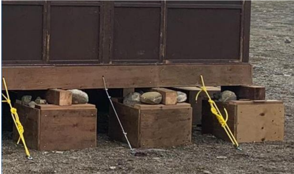
Figure 7. Cribbing placed under cabin and anchors attaching cabin to ground (this photo is from another site but demonstrates the same system that will be used on the cabin at Sinaasiurvik).
