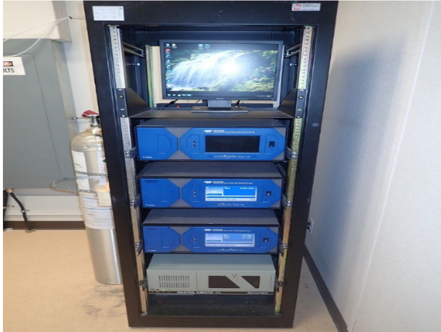
Photo 1.2 The rack-mounted Teledyne T100 (SO 2 ) and T200 (NO x -NO 2 ) continuous gas analyzers at the MSC.
