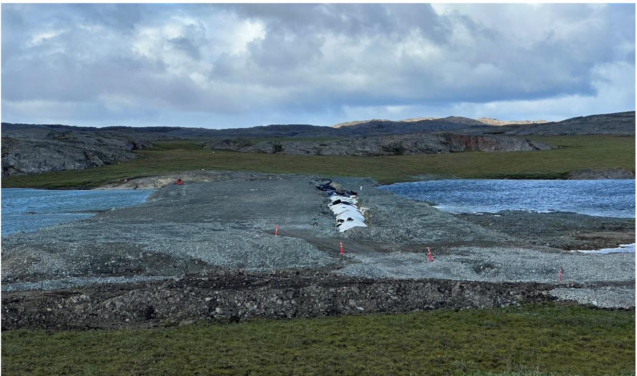
Photo 18: Finished Aqua Dam, measure in place to compliant with the new Metal and Diamond Mining Effluent Discharge Regulations
