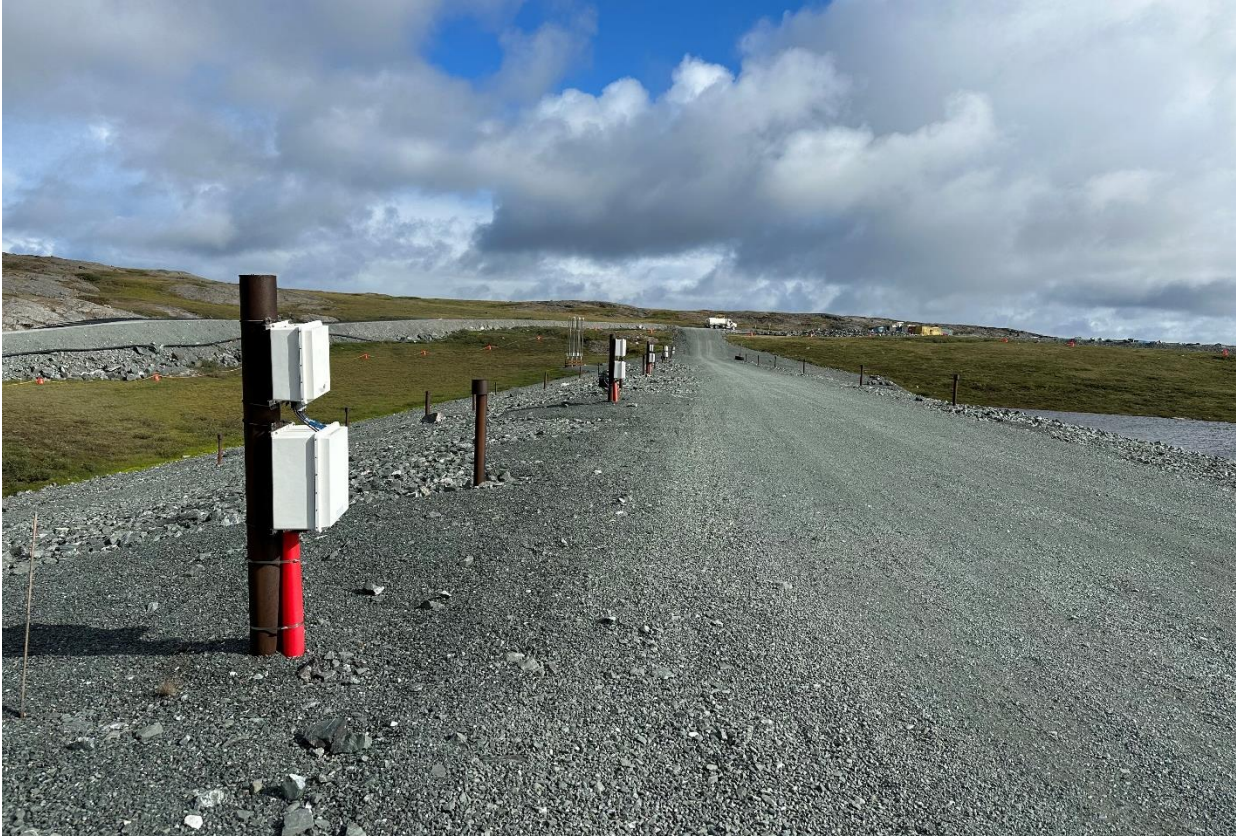
Photo 21: Thermistors at the North Dam
