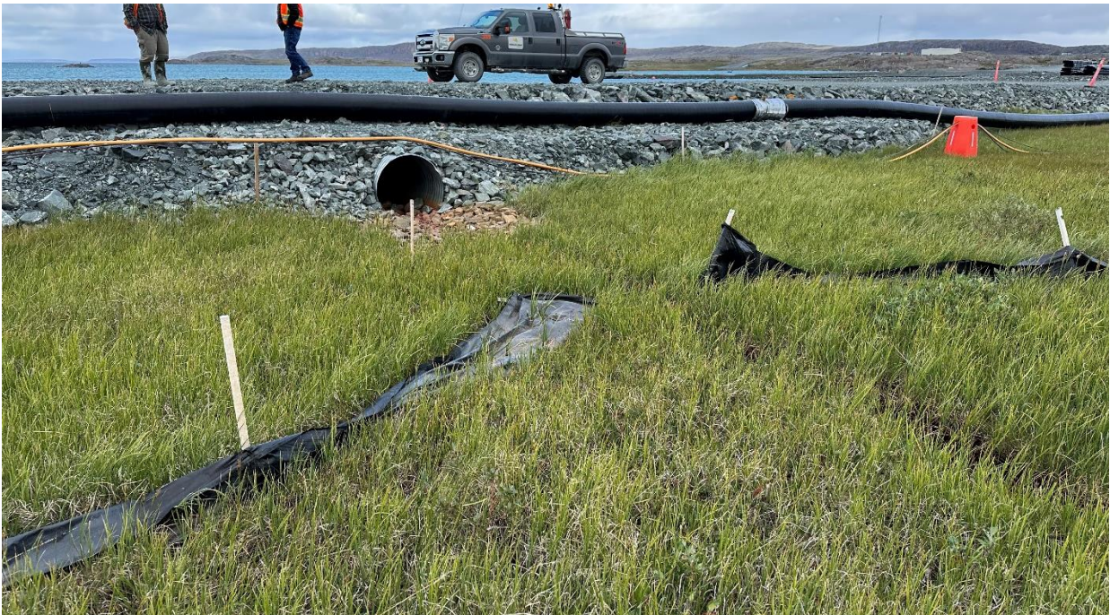
Photo 2: Culvert on the road going to the saline discharge and sedimentation control
