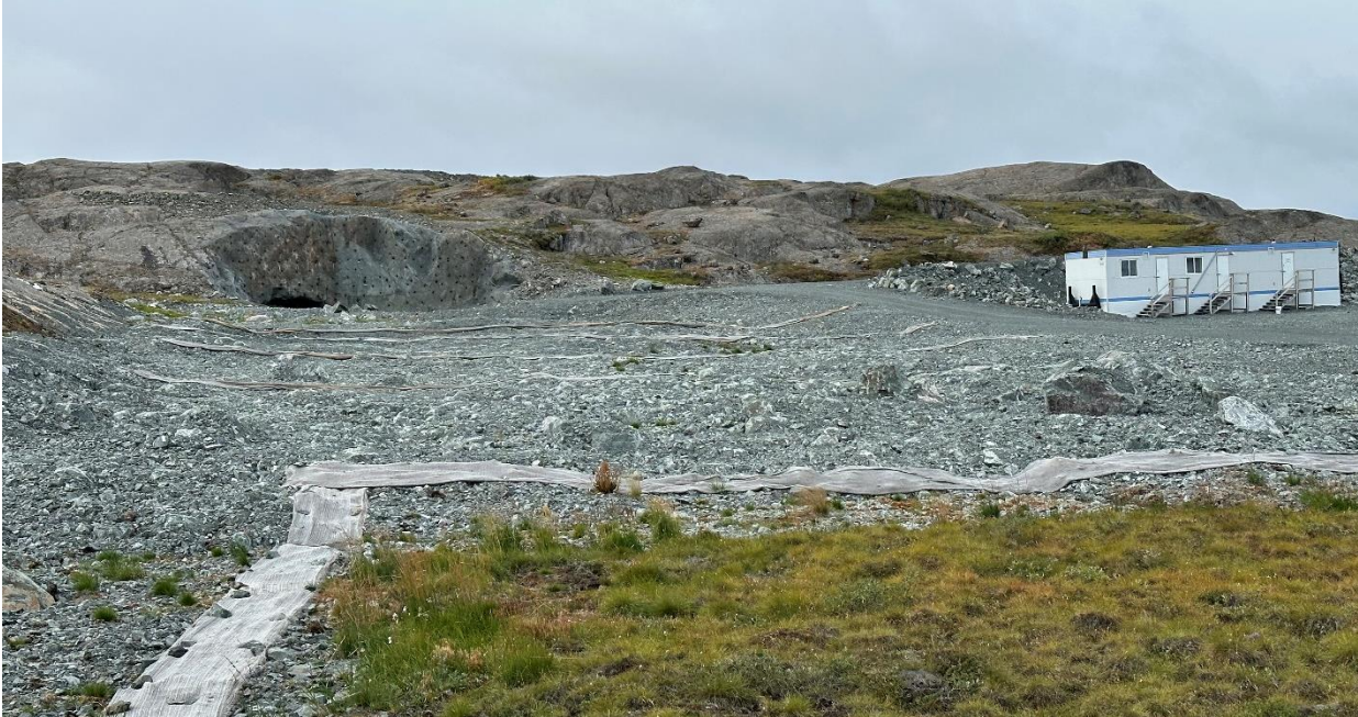
Photo 26: Sedimentation Control at former Madrid Portal
