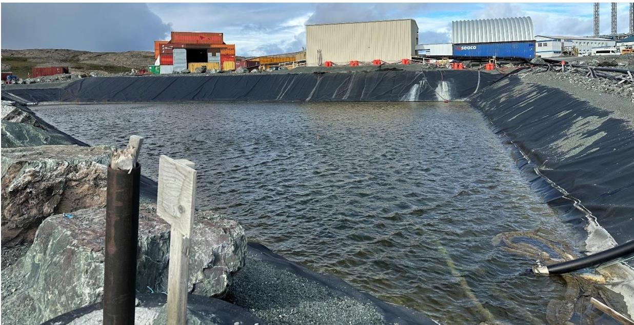
Photo 12: Sedimentation Pond at Doris North which collects Runoff water from Camp site and discharge into Tailings
