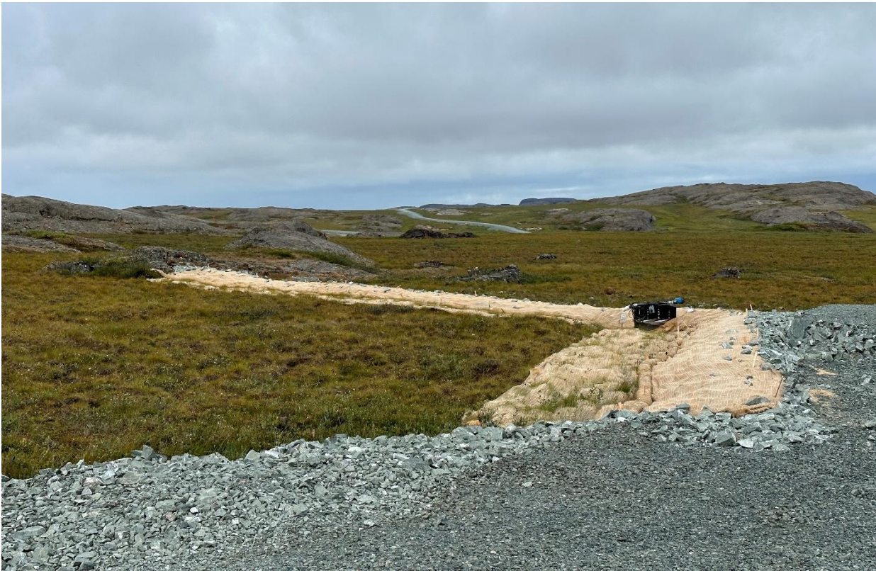
Photo 28: Collection Sump from the PAG Waste Rock Pond leak and new mat to help redirect water
