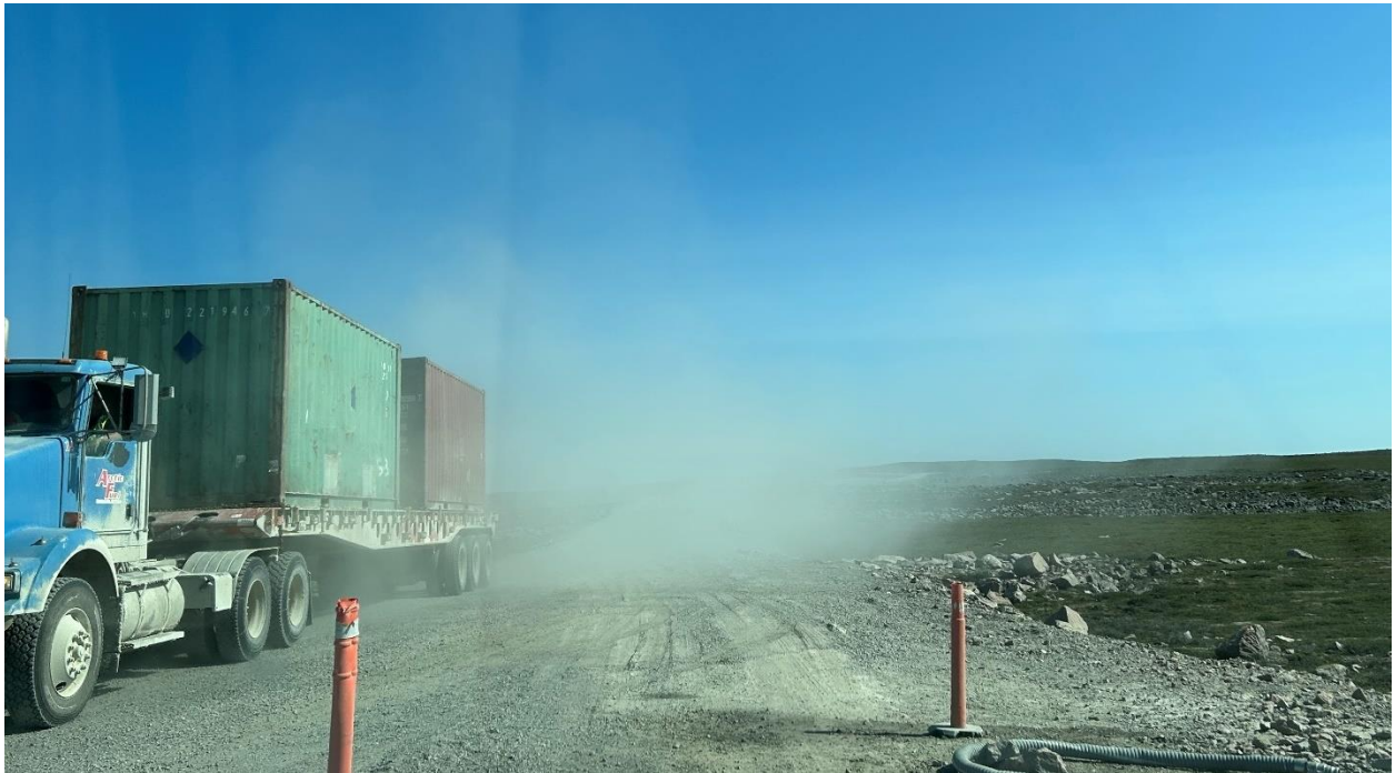
Photo 19: Dusty conditions can be seen on sections of the road that have not received chemical dust suppression treatment.
