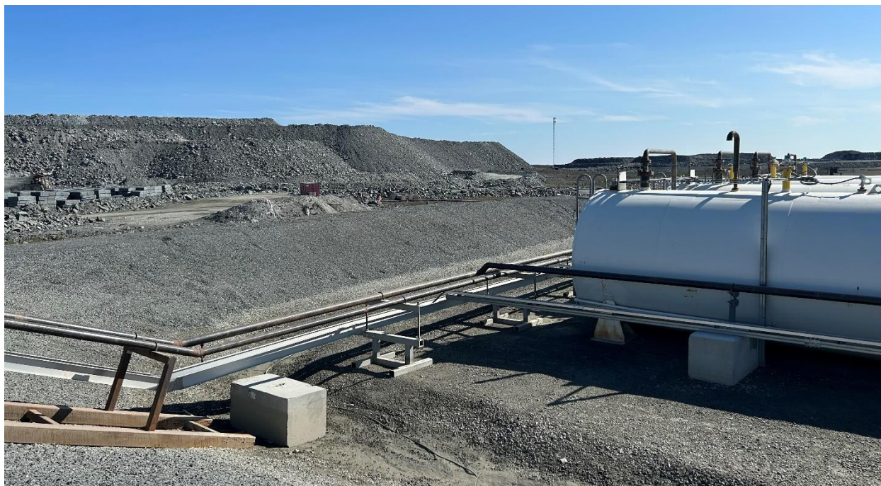
Photo 64: Secondary containment berm around fuel tanks.
