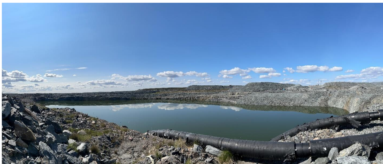
Photo 39: Goose Pit. This pit previously received tailings deposition and is now capped with 35-40 metres of water.
