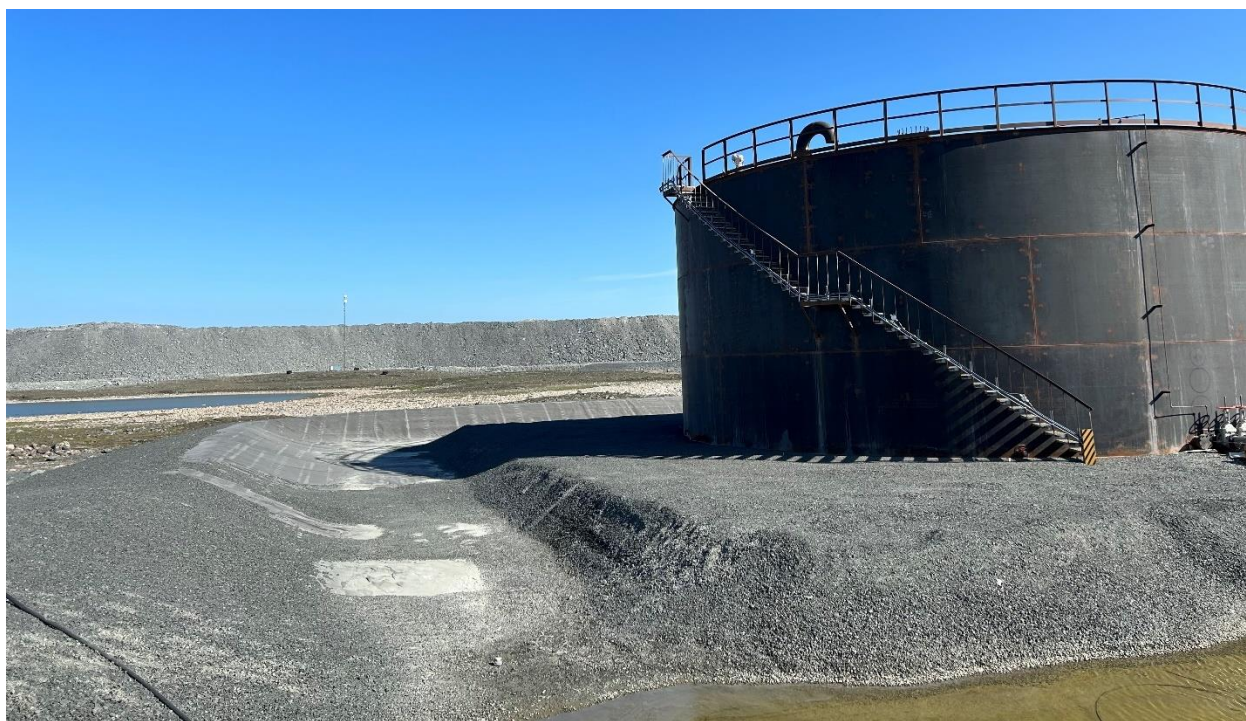
Photo 59: Whale Tail Site tank farm. A large area of exposed liner can be seen in the secondary containment berm.
