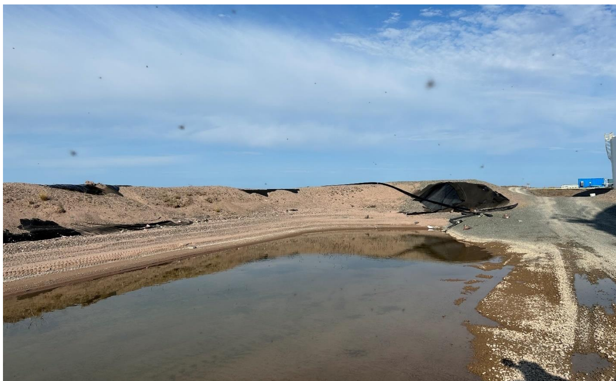
Photo 8: Exposed liner at the Baker Lake Marshalling Facility. Pooled water is being pumped out to be stored in the Stormwater Management Pond at the Meadowbank Site.
