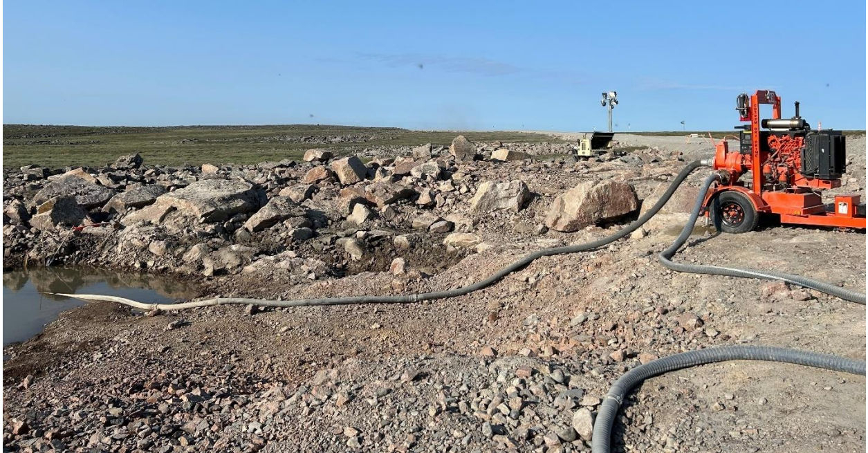
Photo 20: Water pump removing water from a spill cleanup site at kilometer 87 of the AWAR. This was the site of spill in December 2022 and CIRNAC is working with the Proponent on clean-up.
