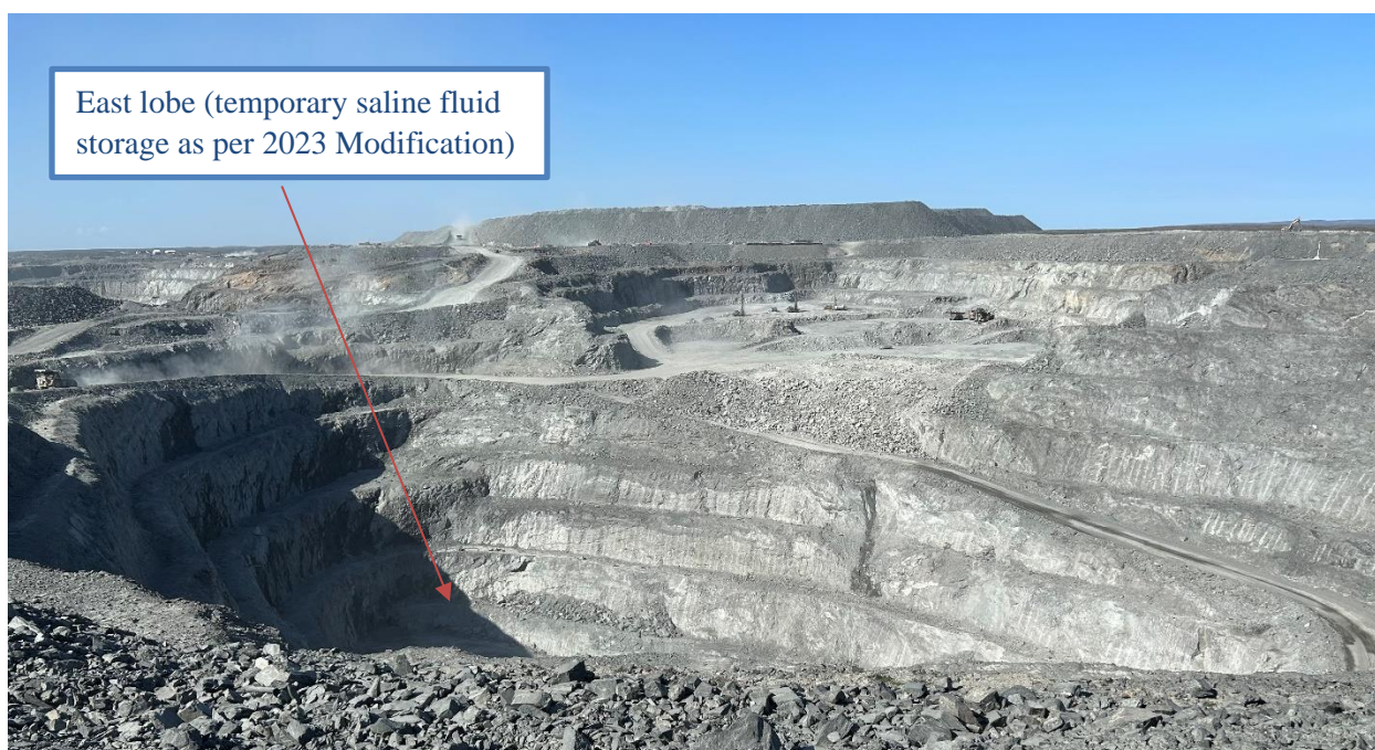
Photo 65: IVR Pit – temporary storage of saline fluid as described in the 2023 modification will occur in the east lobe.
