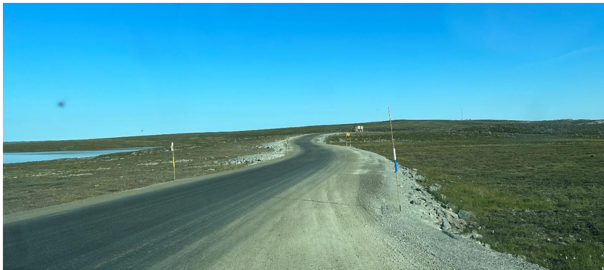
Photo 55: The entirety of the WTHR receives chemical dust suppression treatment.
