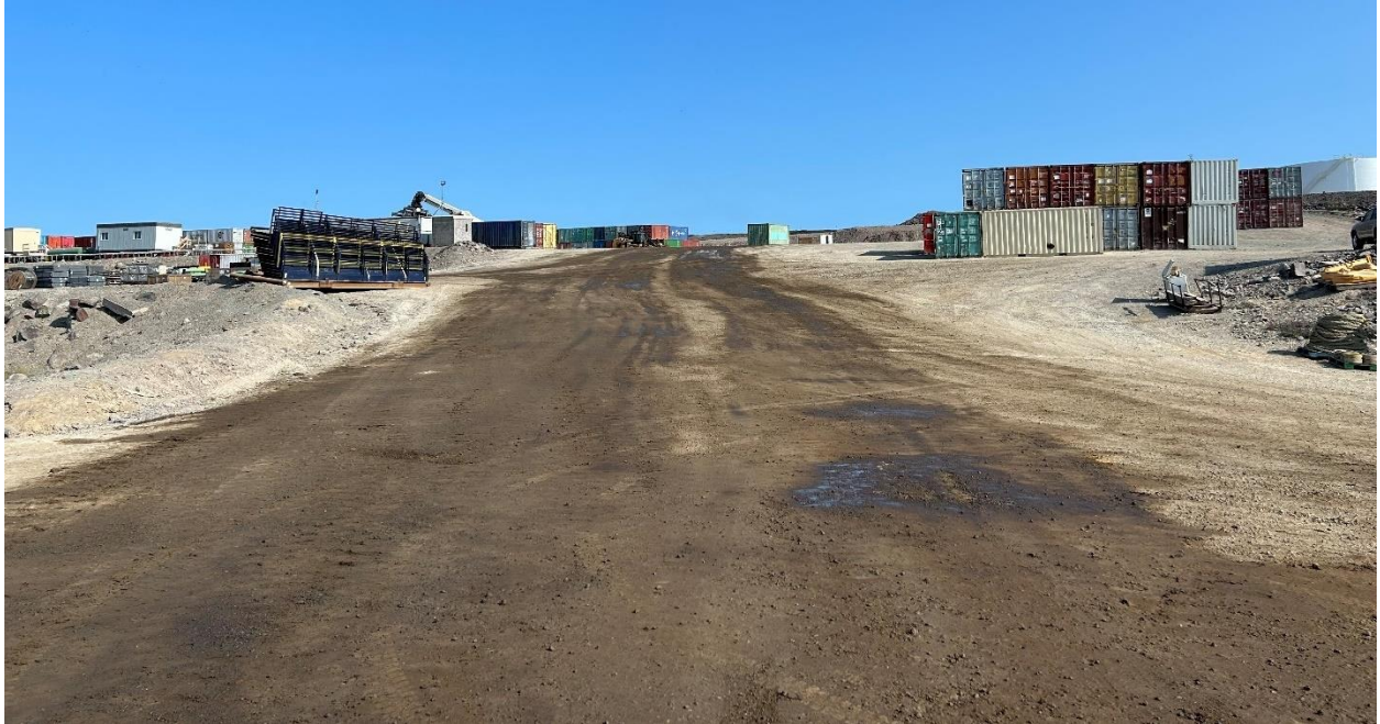
Photo 5: Chemical dust suppression freshly applied to the Baker Lake facilities.
