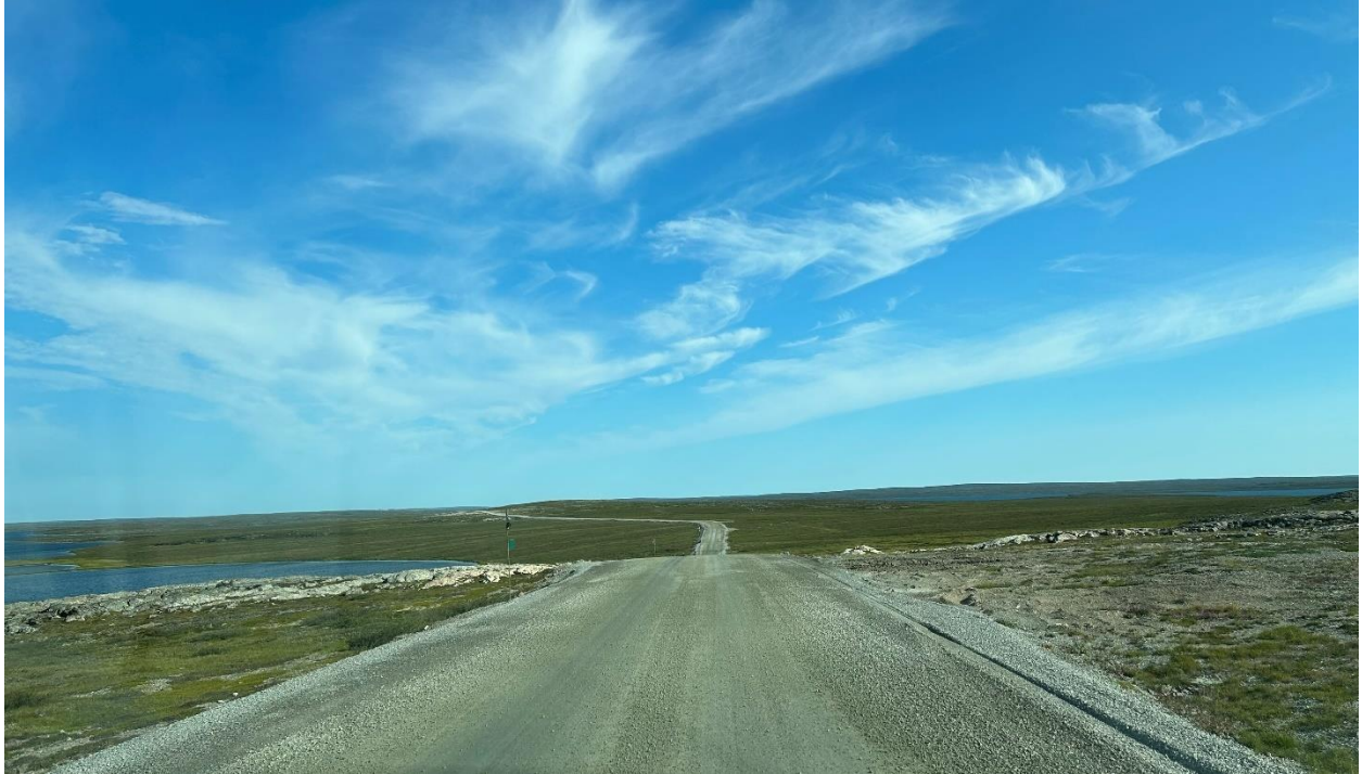
Photo 18: A section of the AWAR that has received chemical dust suppression treatment.
