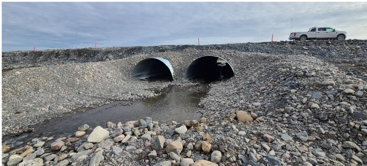
Photo 7: Culverts Installed at Rascal Creek outlet into Goose Lake
