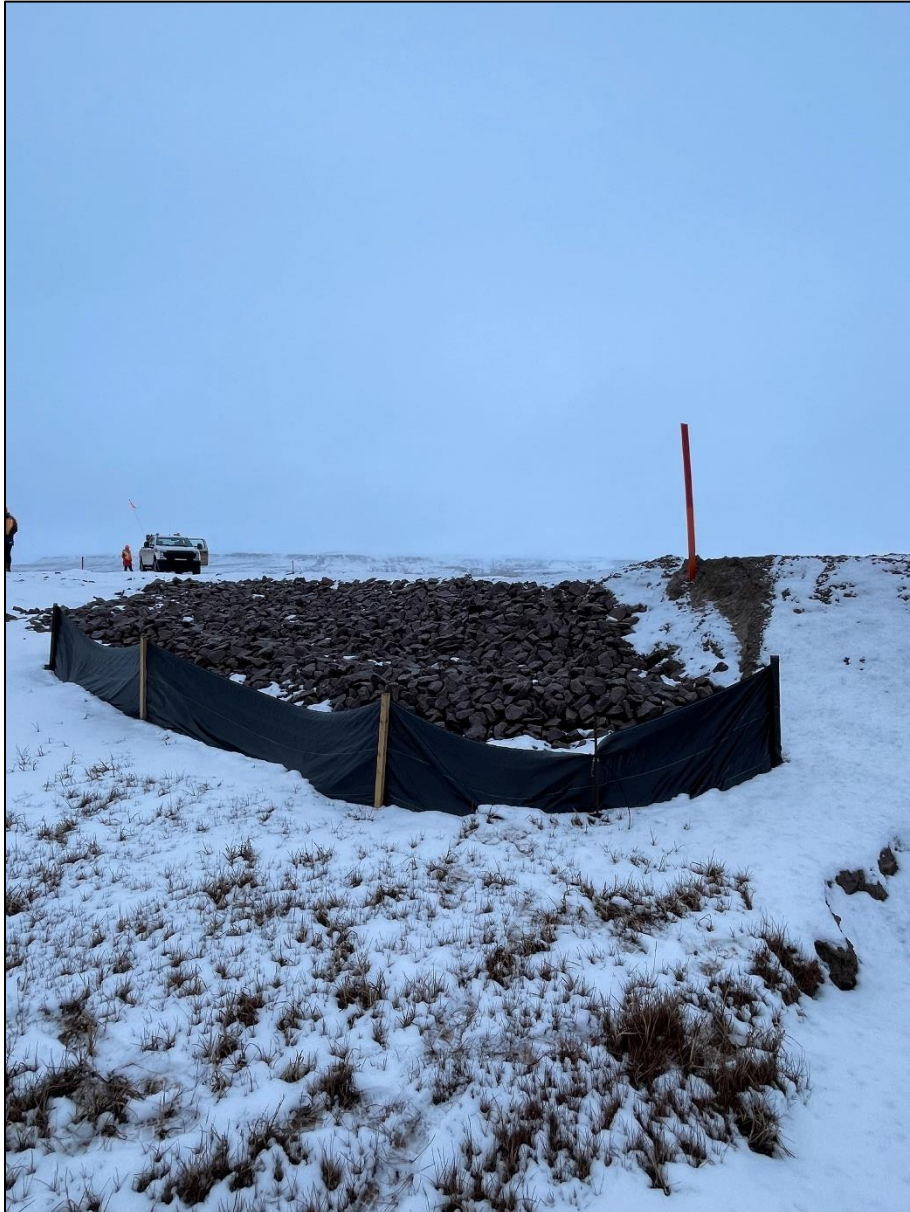
Photo 48: Rip Rap and Check Dam Installed at Culvert CV-215.
