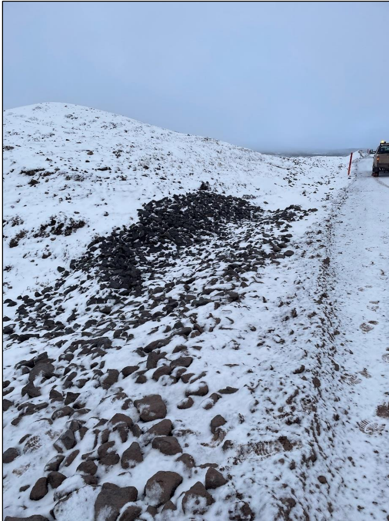
Photo 44: Rip Rap installed to aid in controlling water flow at Culvert CV-079.
