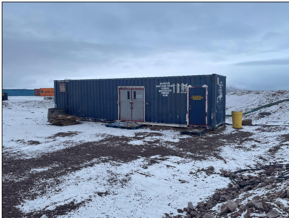
Photo 40: Mobile Oily Water Treatment System located at the Landfarm for Water Treatment.
