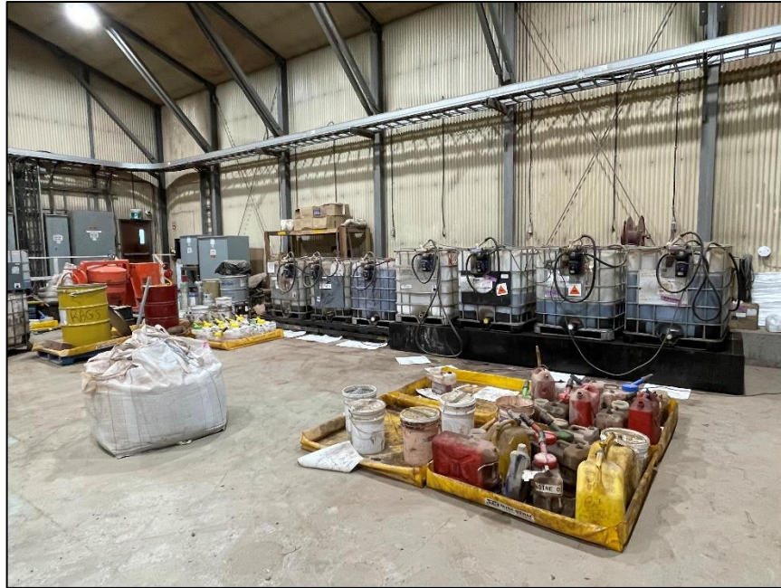
Photo 9: Secondary Containment for Fluid Dispensing Station inside the incinerator facility.
