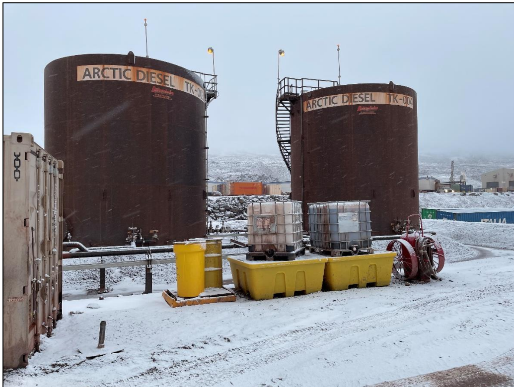
Photo 8: Mine Site Fuel Tank Farm and Secondary Containment.
