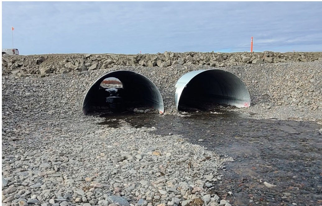
Figure 7. Culvert installation at Gander Outflow
