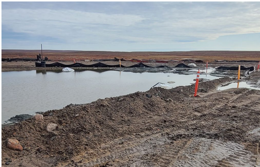
Figure 6. Sedimentation fence installed at exploration cuttings sump
