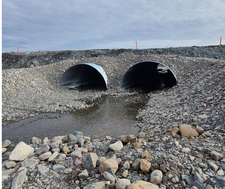
Figure 8. Culvert installation at Gander Outflow
