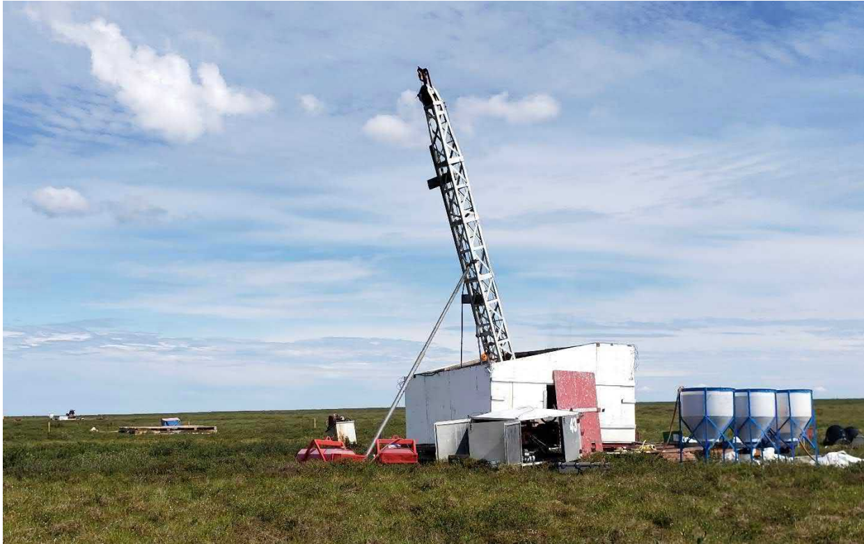
Figure 11: 2022 drilling at Dipole with a Boyles 17 heli-portable rig with cuttings settling tanks.
