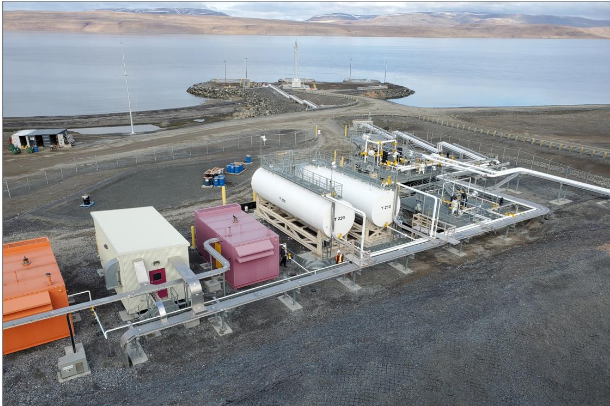
Figure 3. Operational Area (Gensets, POL storage, Diesel tanks, Pump platforms)
