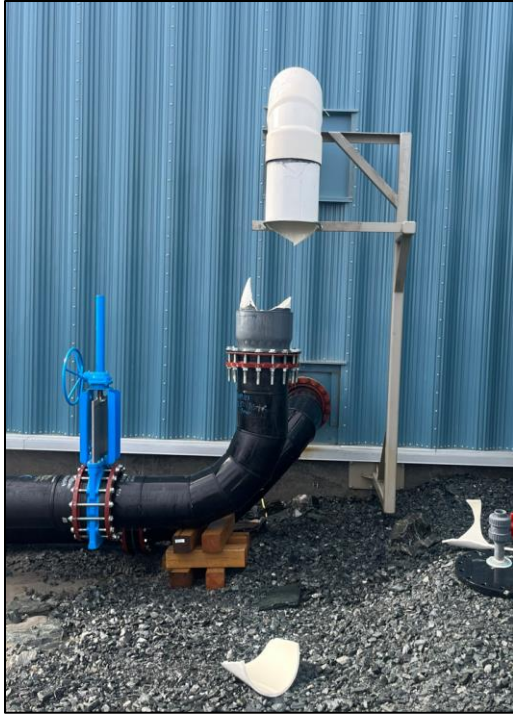
Photo 1: Broken segment of PVC pipe, facing southwest.
