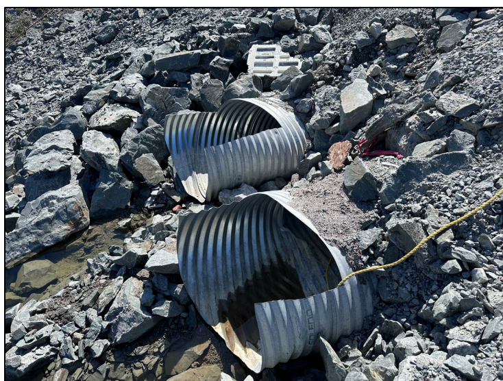
Photo 3 – Temporary repair to the culvert inlets.
