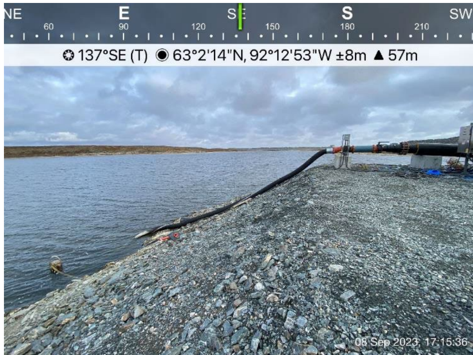
D-CP1 - Photo 18: Dike D-CP1: Jetty 1 water intake - minor erosion, no change from previous years.
