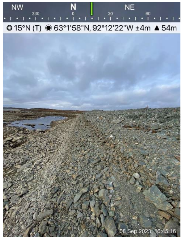
D-CP1 - Photo 2: Dike D-CP1: Upstream face - some wave erosion evident from 2019/2020 high water level event, no change from previous years.
