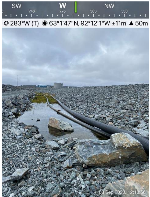
CP6 - Photo 12: CP6 - Ponded water observed between CP6 ramp and CP6 Thermal Berm.
