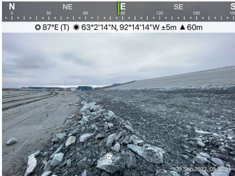
TSF - Photo 2: TSF - Rockfill berm constructed between Cell 1 and Cell 2 tie-in to reduce the surface erosion of north slope of Cell 1.
