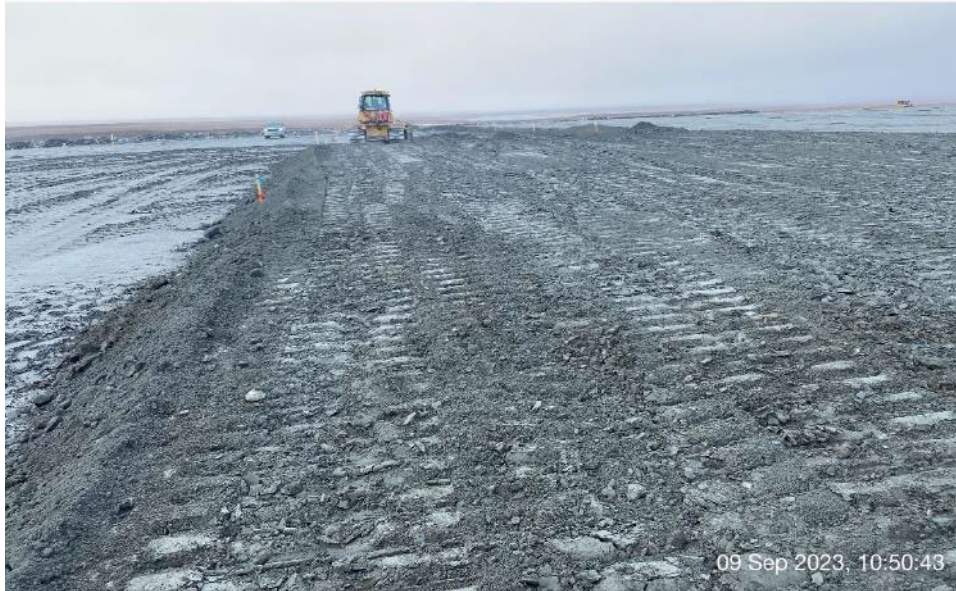
TSF - Photo 9: TSF - Spreading tailings following 0.3 m thick lift control.
