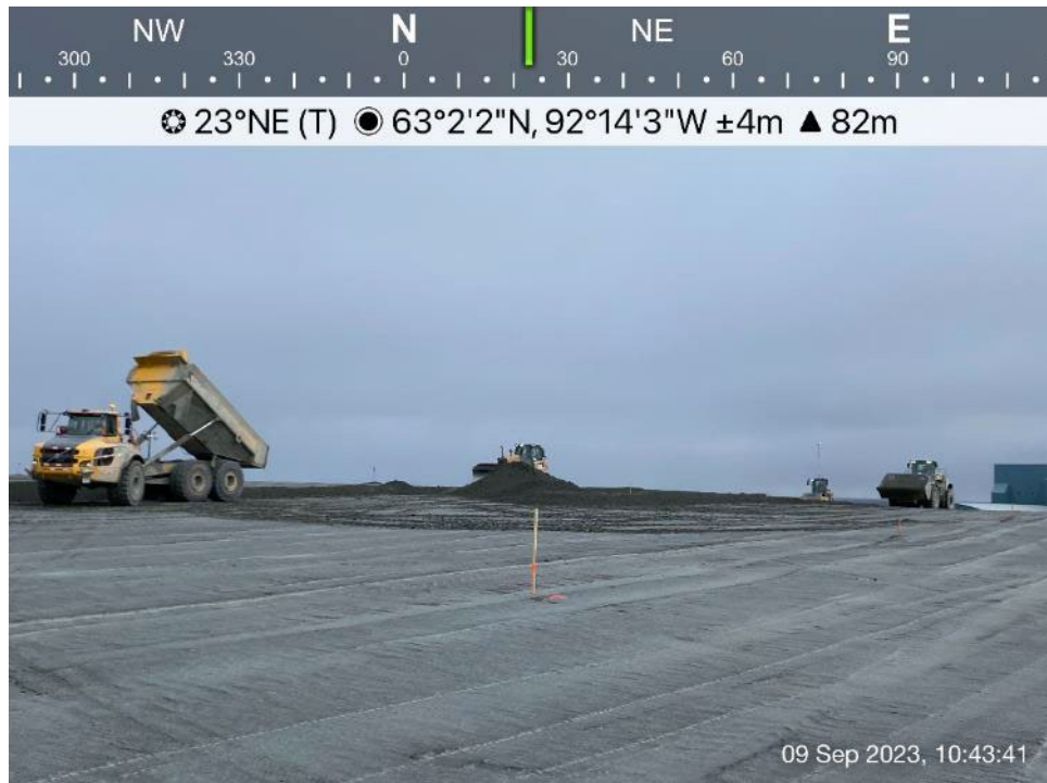
TSF - Photo 6: TSF - dumping, spreading and compacting of the tailings in Cell 1.
