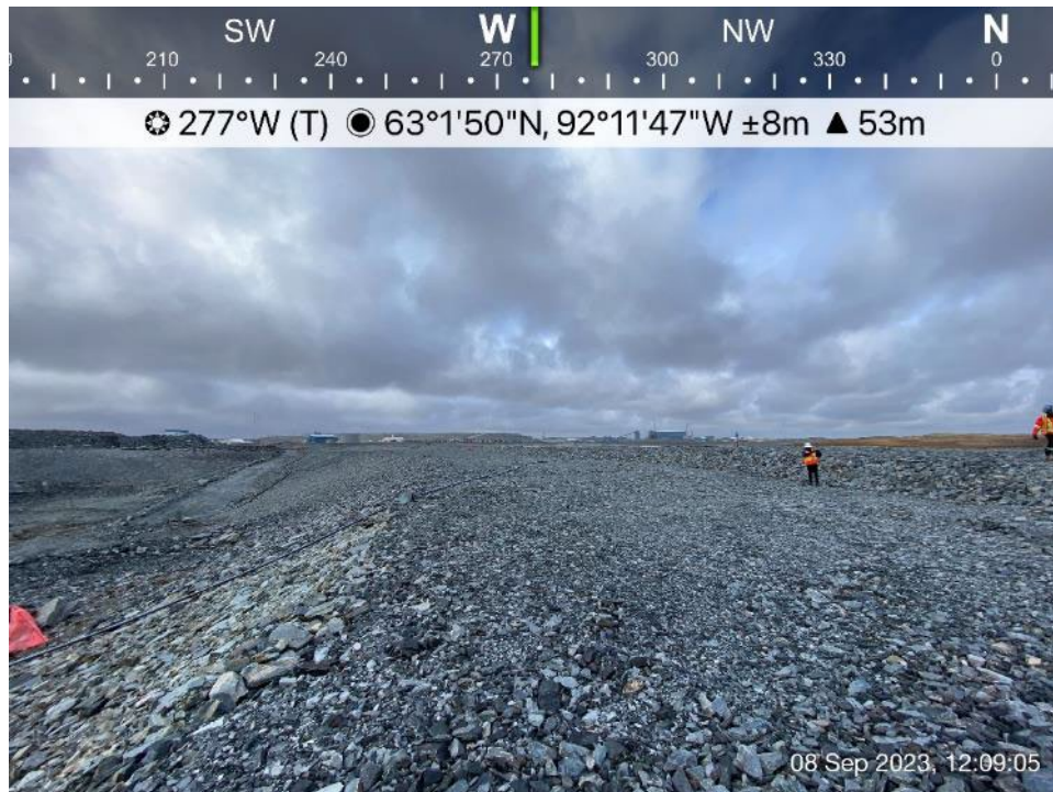
CP6 - Photo 8: CP6 Thermal Berm, looking west, berm crest and upstream slope, CP6 on the left.
