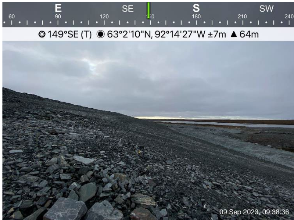
TSF - Photo 5: TSF - Rockfill cover slope along west side of Cell 1, looking southeast.
