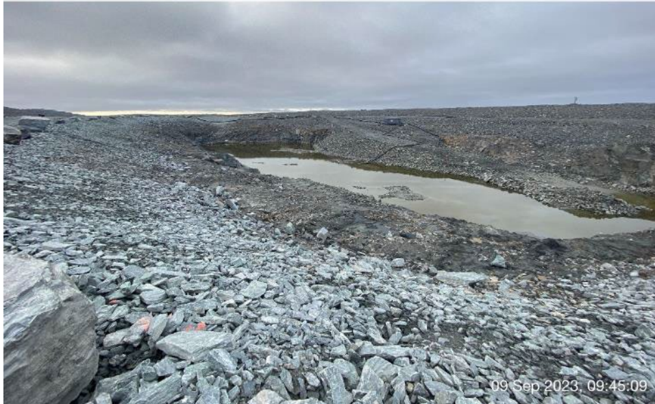
CP3 - Photo 1: CP3 - Small amount of water stored in CP3, bedrock slopes with fractured rock, no stability concern.
