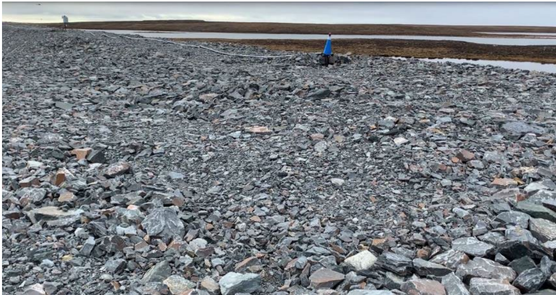
CP3 - Photo 5: CP3 Thermal Berm - Settlement observed on the crest of CP3 Thermal Berm due to thaw settlement.
