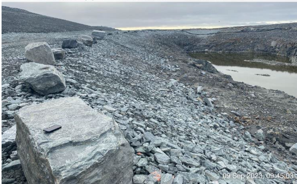
CP3 - Photo 2: CP3- waste rock cover placed between TSF toe and CP3 as thermal protection.
