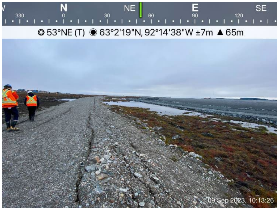
Berm 2 - Photo 13: Berm 2 - ponded water on both sides, cracking observed on slope and crest.
