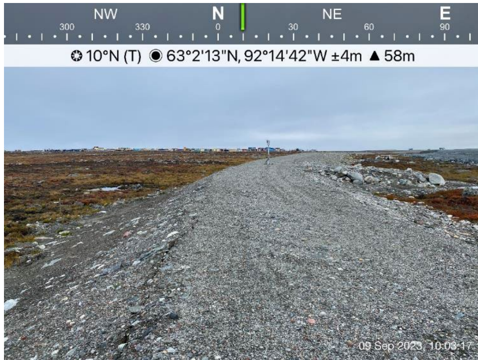
Berm 2 - Photo 10: Berm 2 - Berm 2 south portion, slope and crest, cracking observed on downstream slope.
