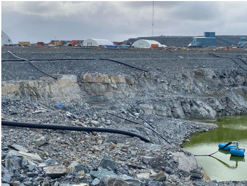
SP1 - Photo 3: SP1 Saline Pond - Perimeter berm side slope and bedrock side wall.
