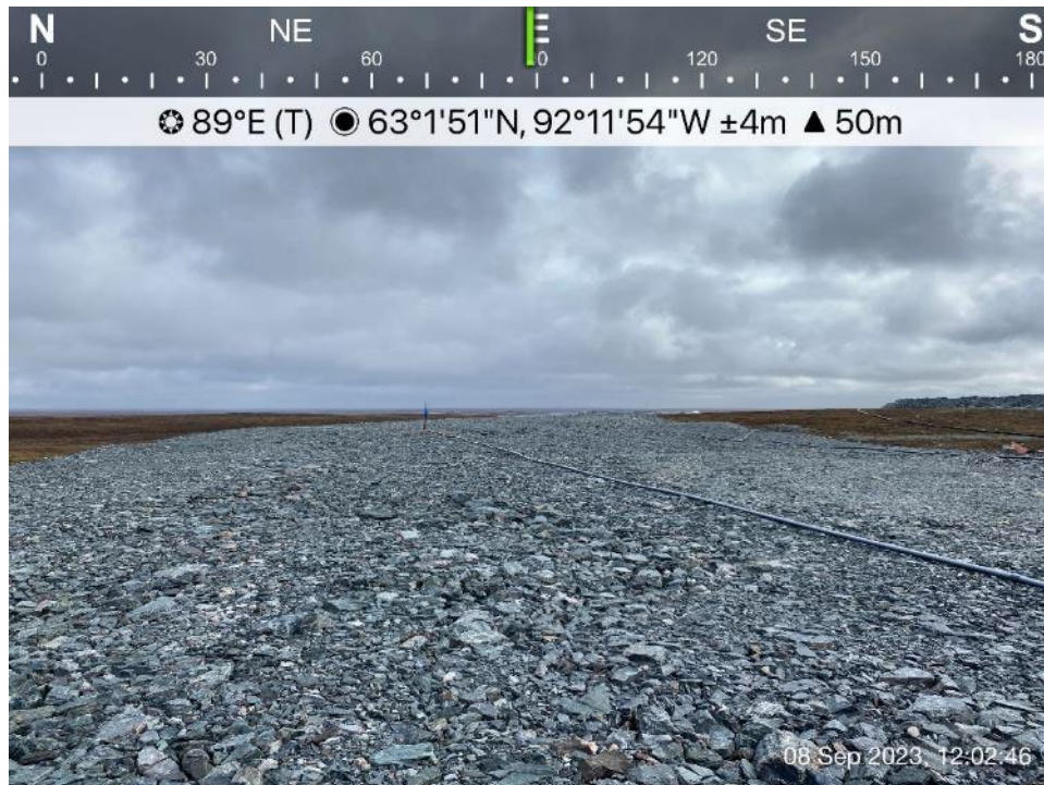
CP6 - Photo 7: CP6 Thermal Berm, looking east, crest, thaw settlement observed at various areas.
