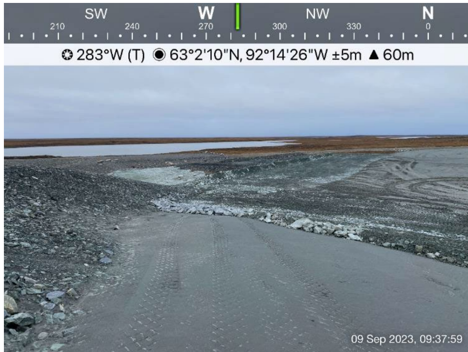
TSF - Photo 4: TSF - Rockfill cover of tailings along west side of Cell 2, looking west.
