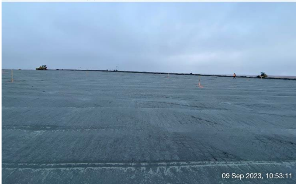
TSF - Photo 10: TSF - Compacted tailings surface.
