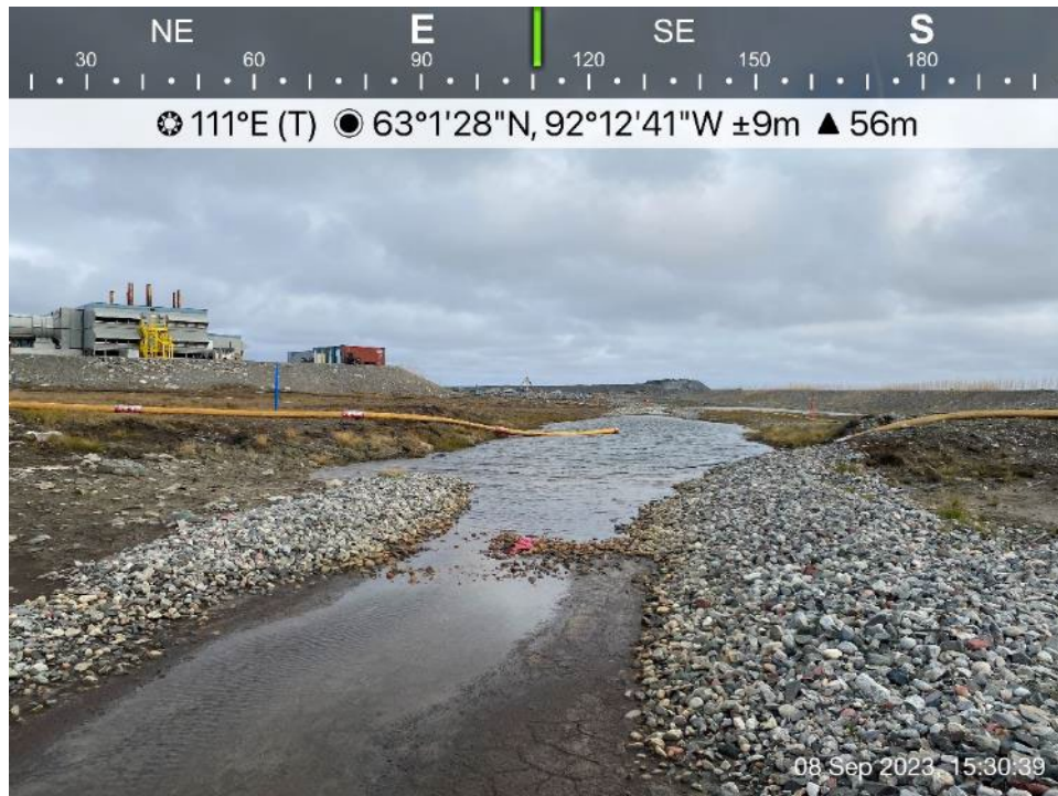
Channel 5 - Photo 14: Channel 5 - Upper section of Channel 5, significant subsidence and cracking along slopes with riprap settled below water level in channel, filled with sedimentation from surface erosion.
