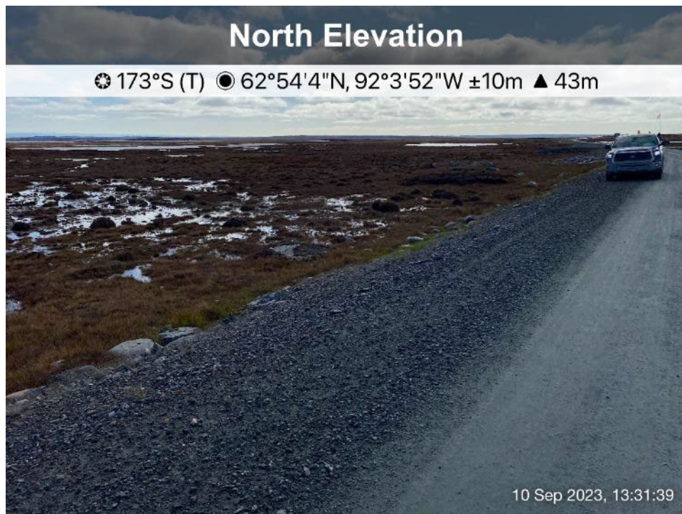
AWAR Road/Culvert - Photo 34: KM 12.6 - No culvert installed, poor drainage condition, no sign of water flow.
