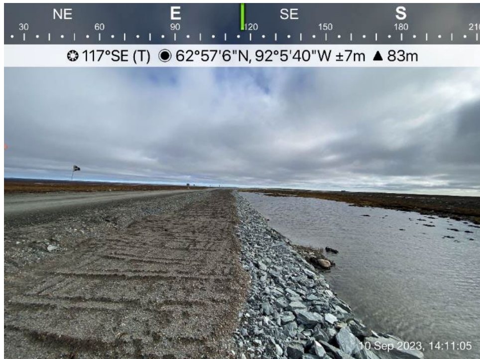
AWAR Road/Culvert - Photo 48: KM 19 - No culvert installed, ponded water upstream, no sign of overflow.
