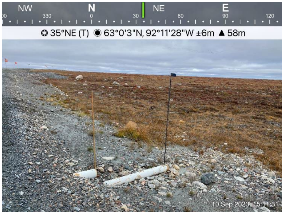
AWAR Road/Culvert - Photo 63: Culvert KM 26.8 - steel pipe as culvert, inlet is above water level.
