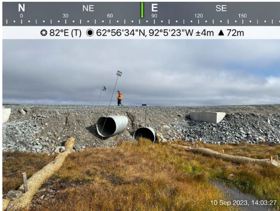
AWAR Road/Culvert - Photo 45: Culvert KM 18.1- outlet.
