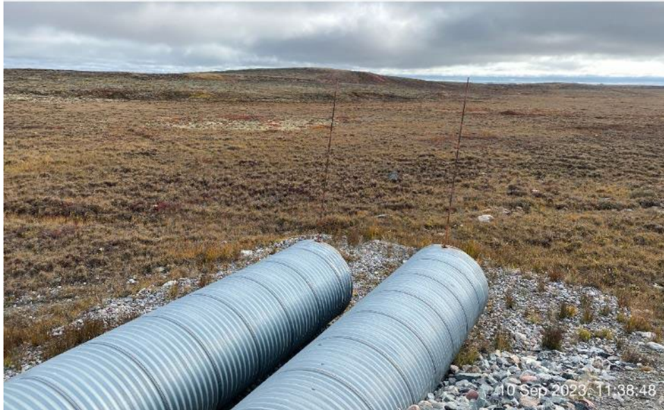
Itivia Bypass Road/Culvert - Photo 47: Culvert C17 inlet.
