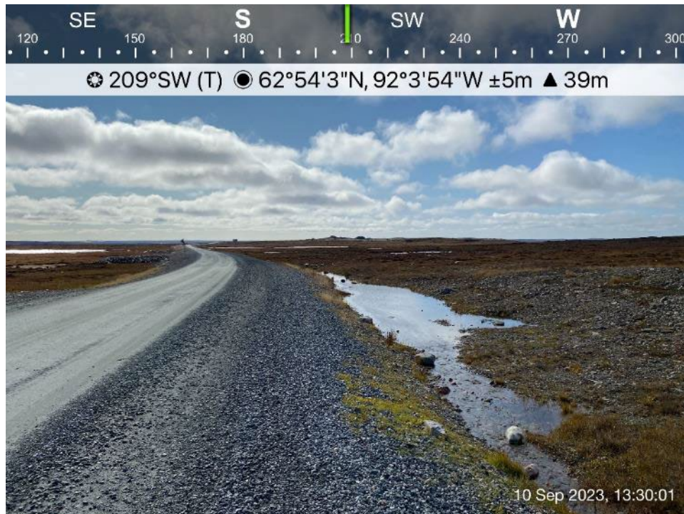
AWAR Road/Culvert - Photo 33: KM 12.6 - No culvert installed, poor drainage condition, no sign of water flow.
