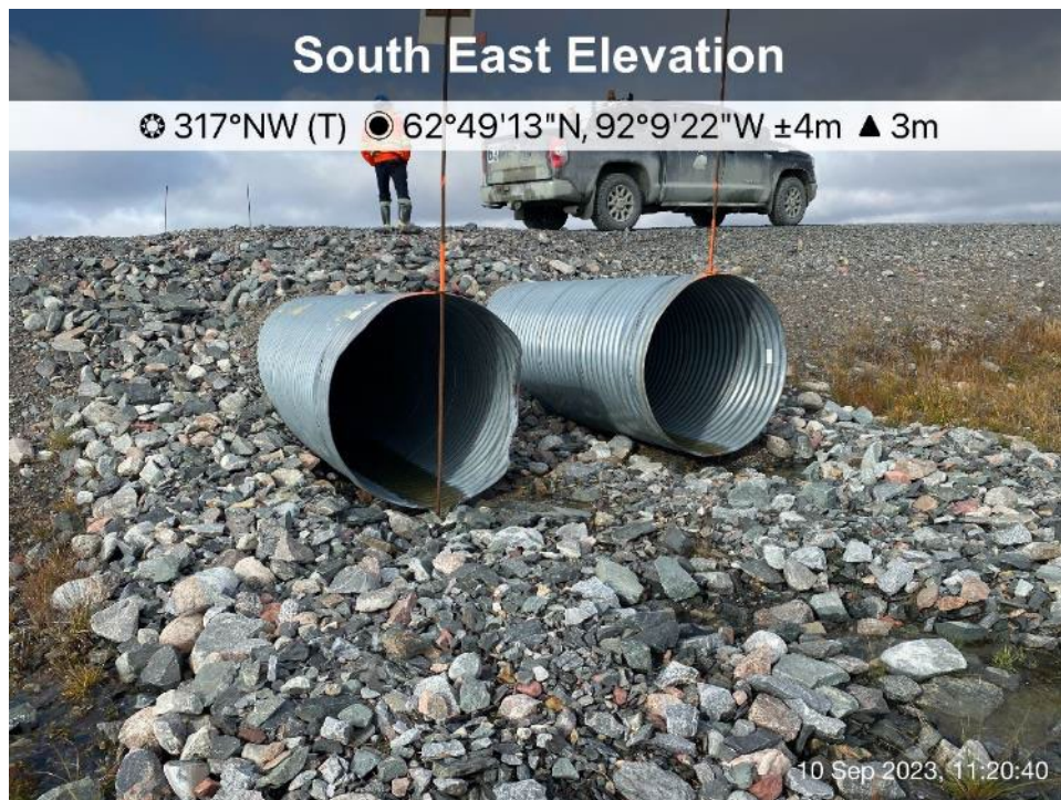
Itivia Bypass Road/Culvert - Photo 34: Culvert C12 inlet.
