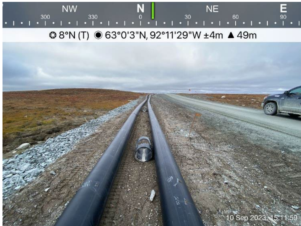
AWAR Road/Culvert - Photo 64: Culvert KM 26.8 - steel pipe as culvert, outlet was buried during the waterline project construction.
