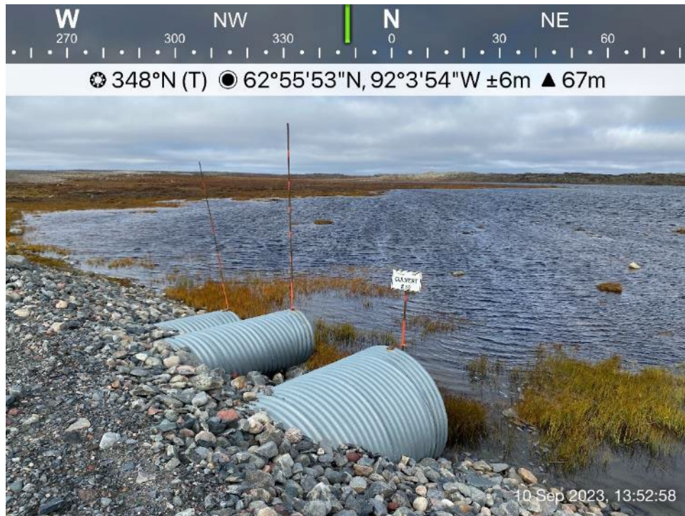
AWAR Road/Culvert - Photo 40: Culvert KM 16.3 – inlet.
