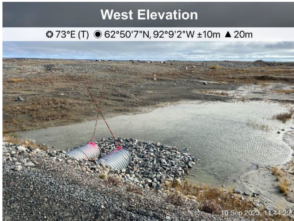
Itivia Bypass Road/Culvert - Photo 50: Culvert C18 inlet.
