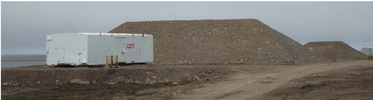
Figure 3-4 Surface Explosive Magazines and Berms
