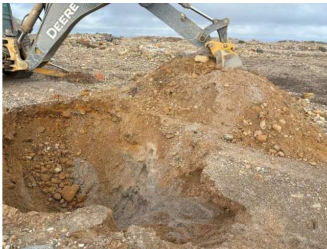
Photograph 13: Test Pit 13, Site 3, excavation in progress
