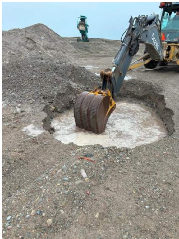
Photograph 17: Test Pit 2, Site 4, test pit excavation in progress. Note high groundwater table.
