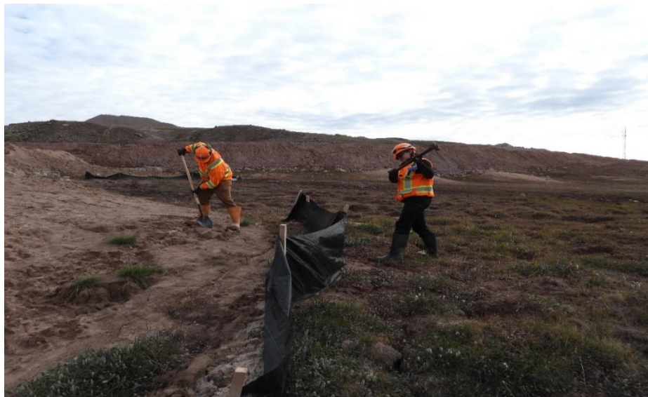
Photo 14: Silt Fence Installation along the Tote Road – August 2024
