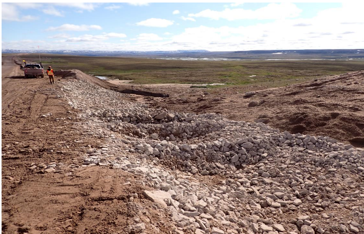
Photo 8: Check Dams Constructed and Silt Fencing Installed along the Tote Road – July 2024
