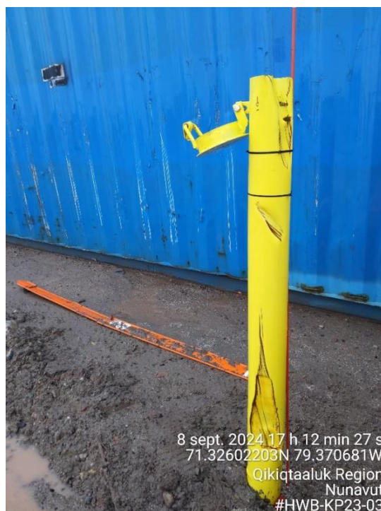
Photo A-32: Standpipe well HWB-KP23-03 (8 September 2024) – Metal casing is damaged.
