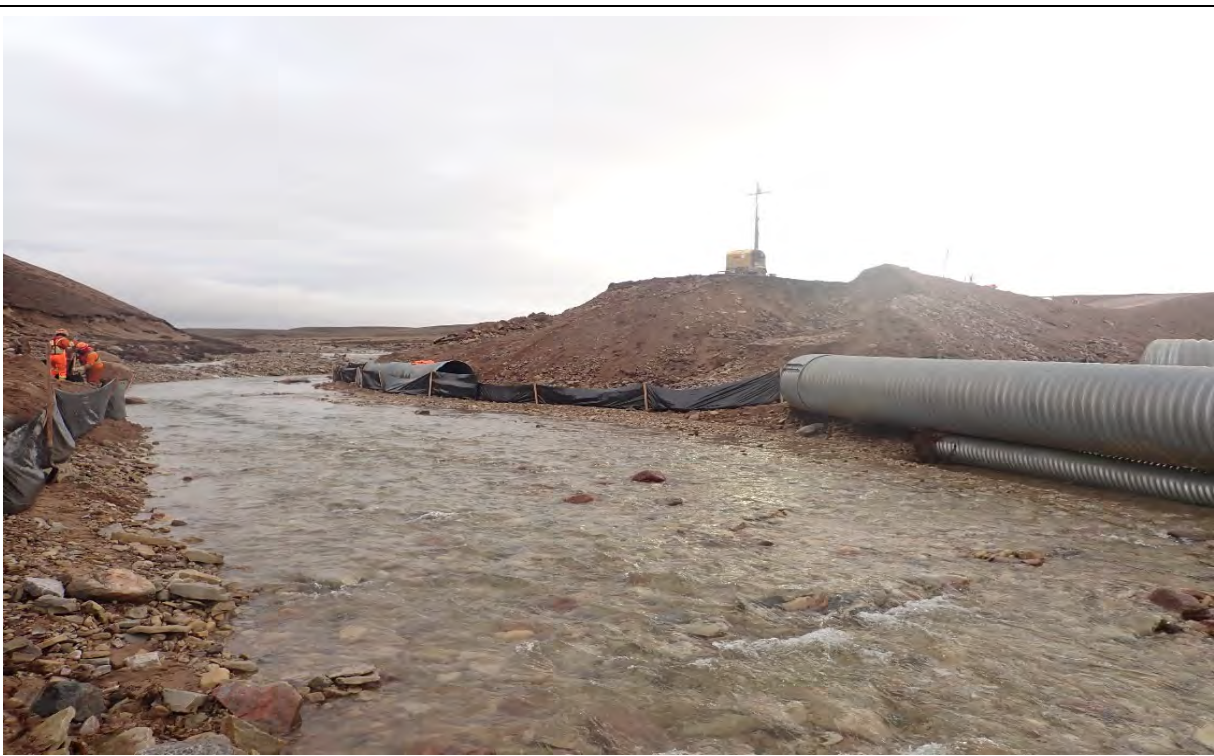
Photo 24. CV-049 looking upstream, silte fence installed to prevent sediment deposition into watercourse during to re-construction of the washed out crossing.
