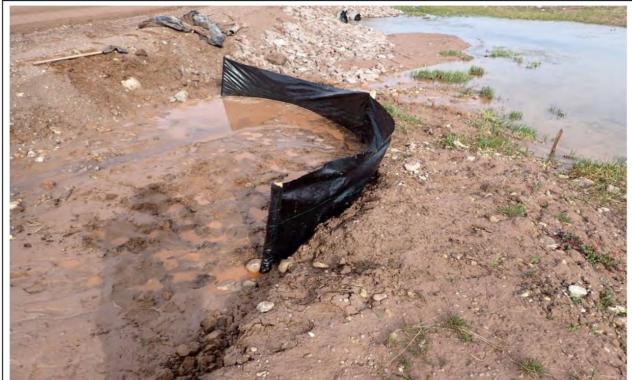
Photo 15. CV-060 downstream, silt fence replaced.
