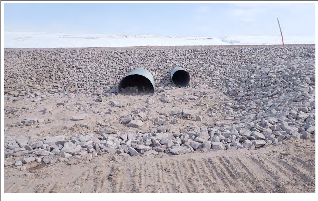
Photo 5. CV-106 downstream, culvert outlet after remedial construction.
