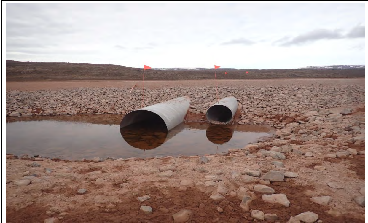
Photo 37. CV-001 downstream, culvert outlet after remedial construction.
