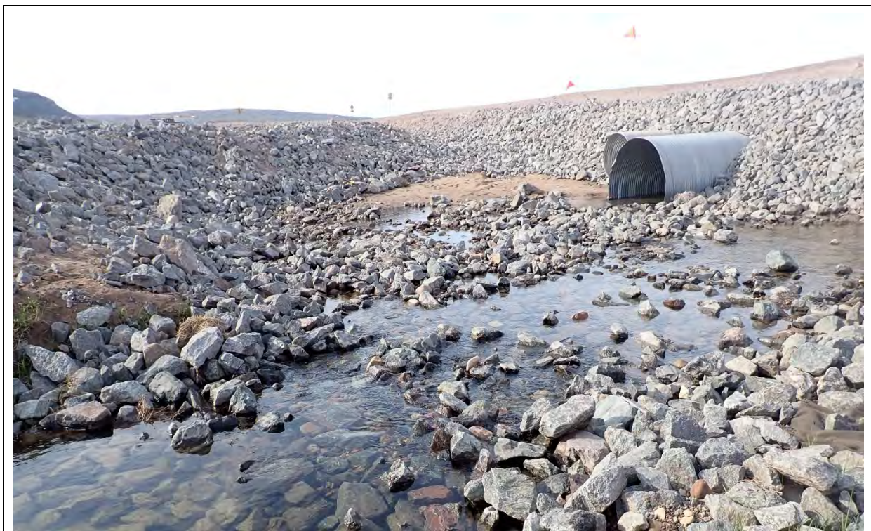
Photo 16. CV-059 upstream culvert inlet after remedial construction.
