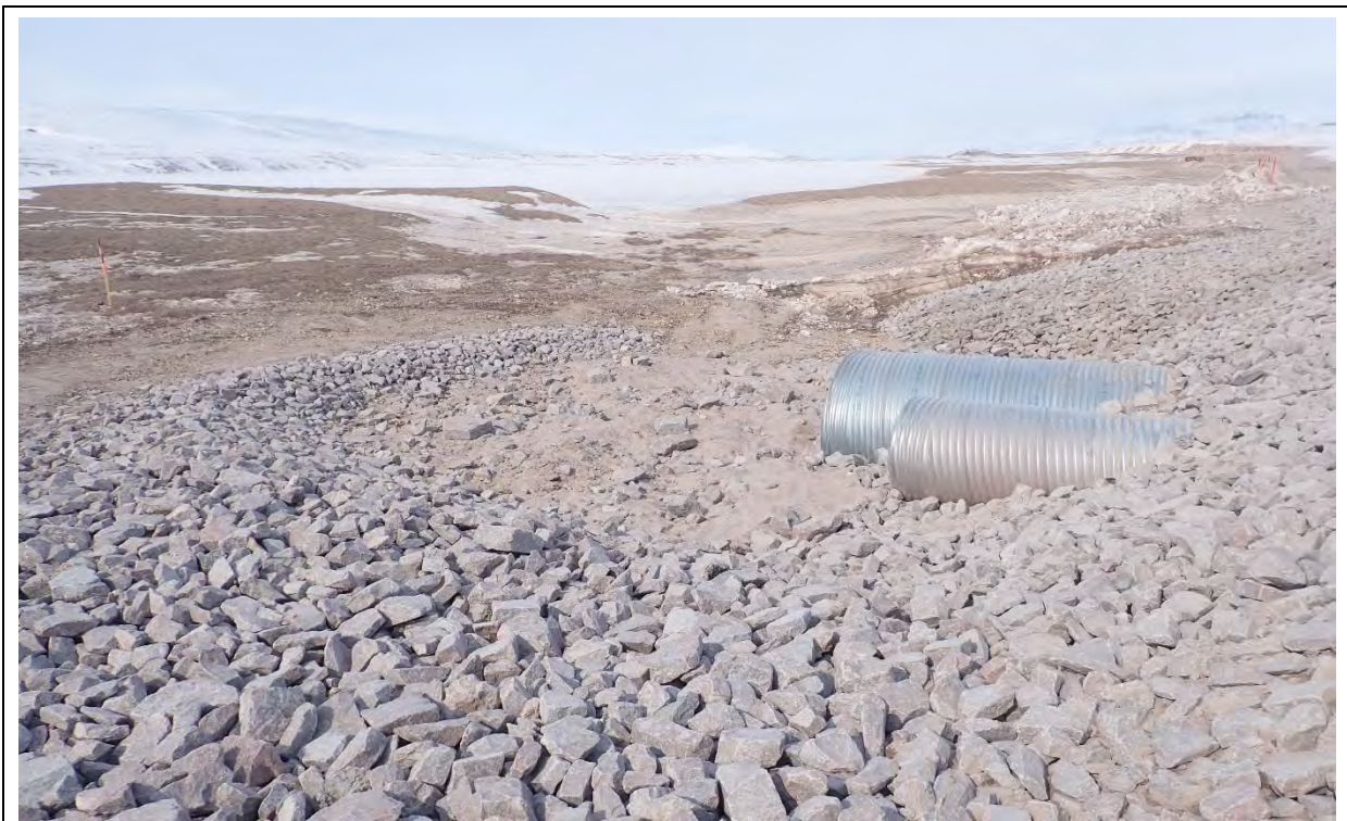
Photo 6. CV-106 downstream, culvert outlet apron after remedial construction.
