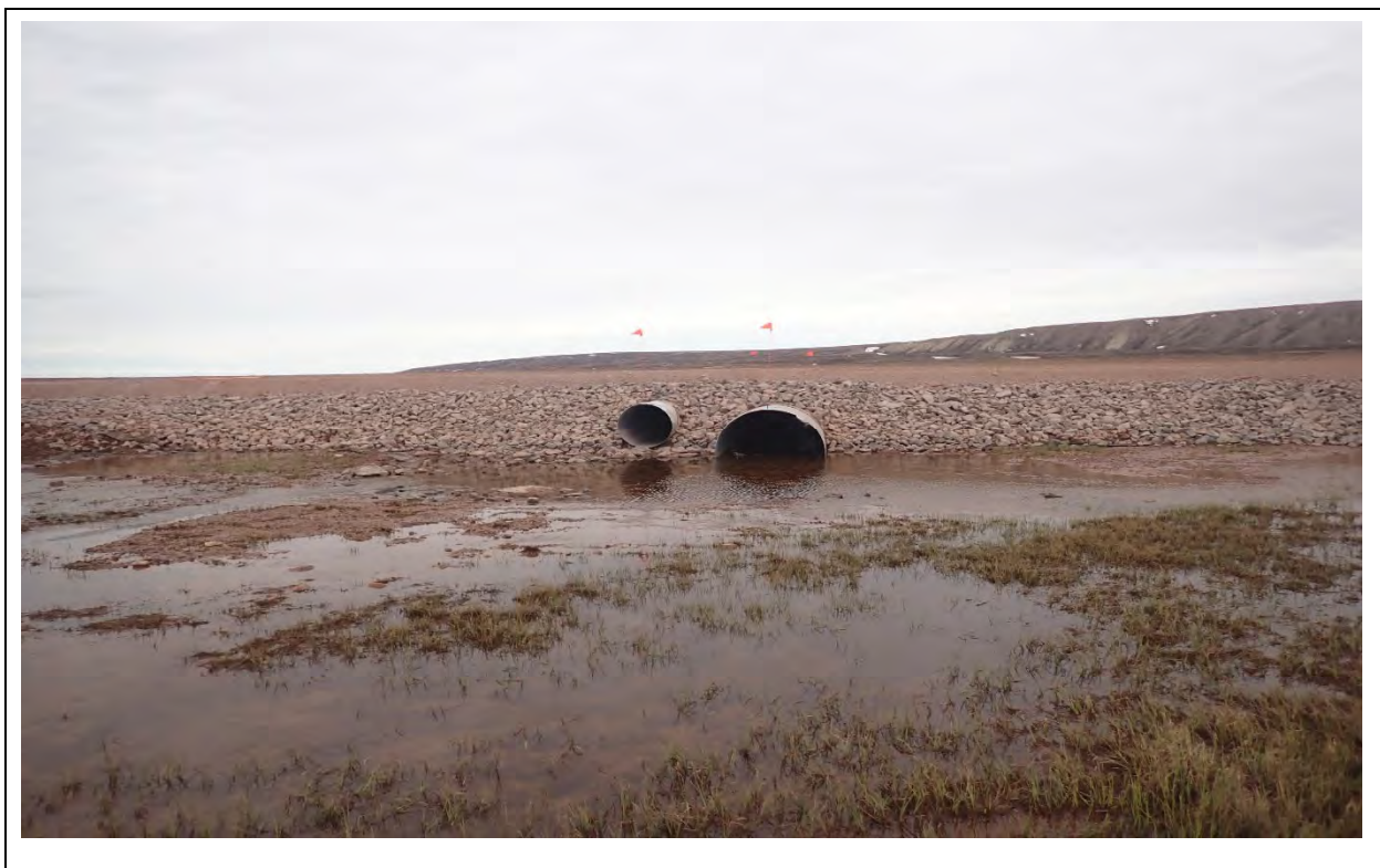
Photo 36. CV-001 upstream, culvert inlet after remedial construction.
