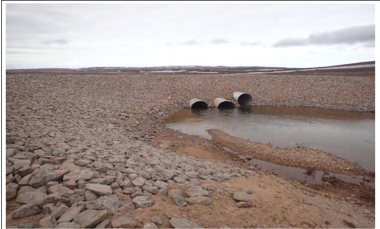
Photo 35. BG-04 downstream, culvert outlet apron after remedial construction.
