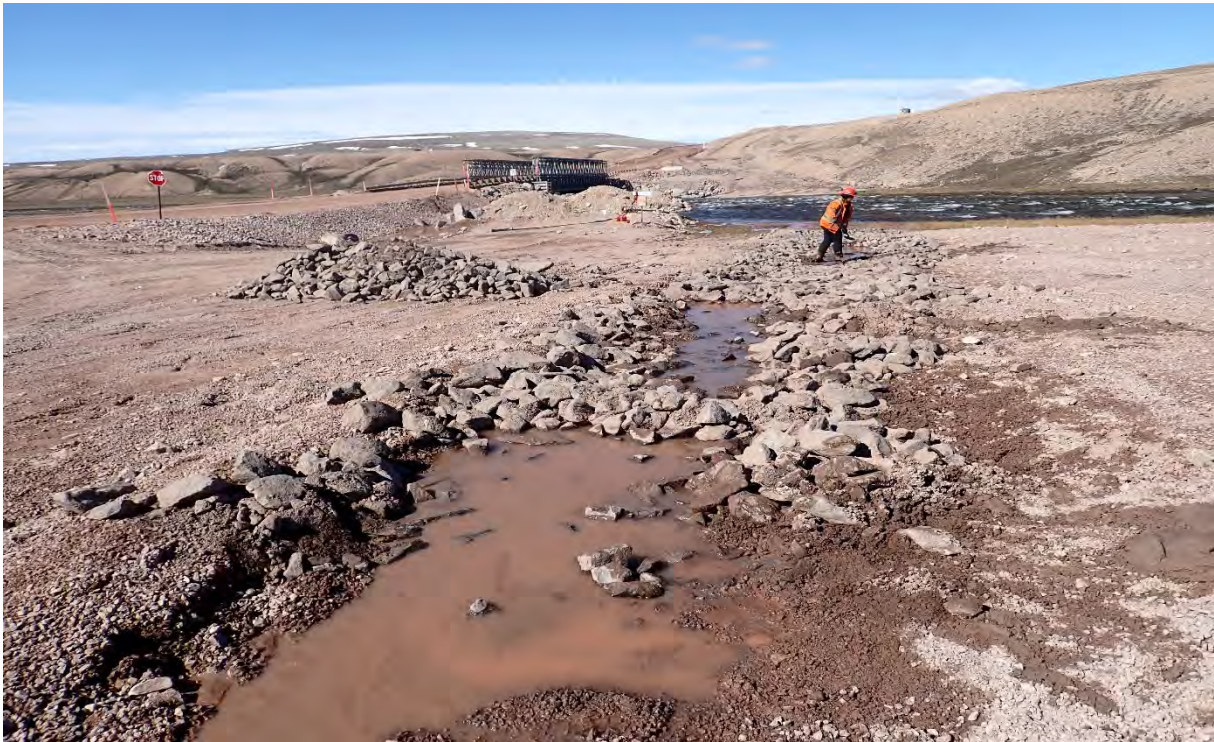
Photo 23. BG-50 sediment removal from snow stockpile check dams.
