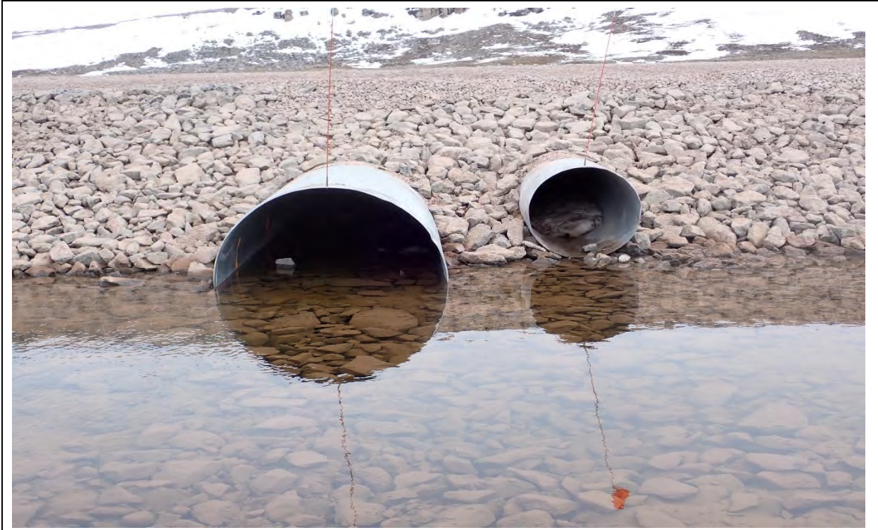
Photo 21. CV-057 downstream culvert outlet after remedial construction.
