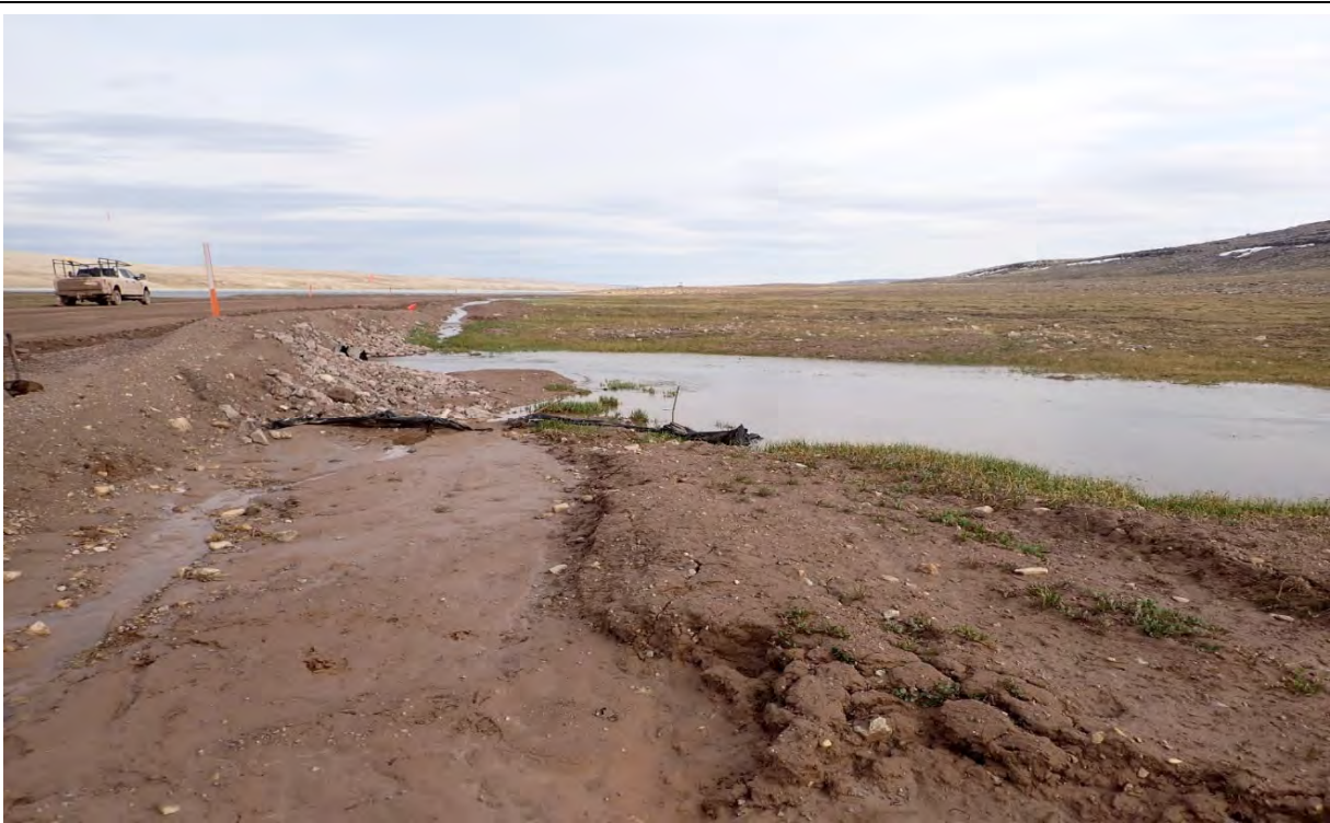
Photo 14. CV-060 downstream, silt fence in disrepair.
