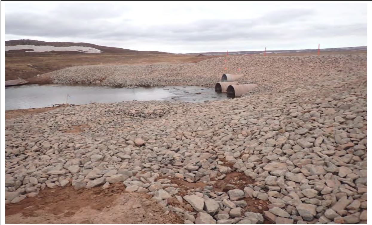
Photo 33. BG-04 upstream, culvert inlet and apron after remedial construction.
