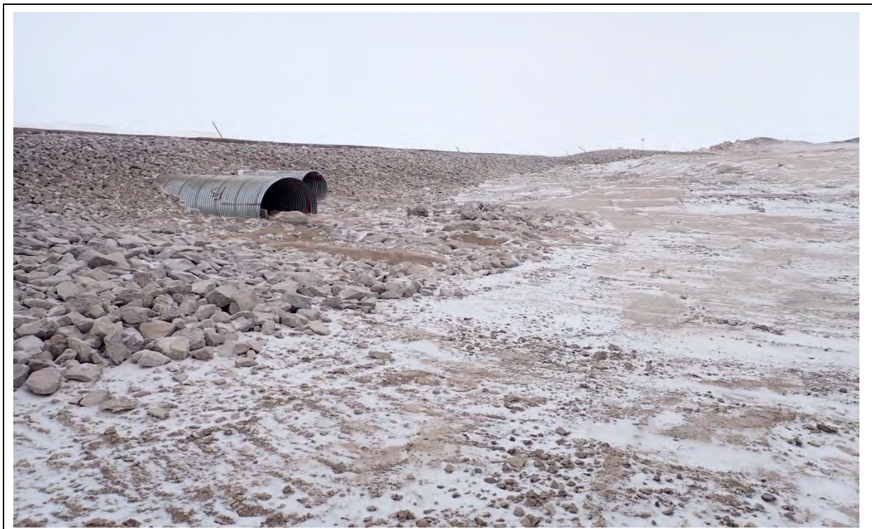
Photo 10. CV-102 downstream, culvert outlet apron after remedial construction.
