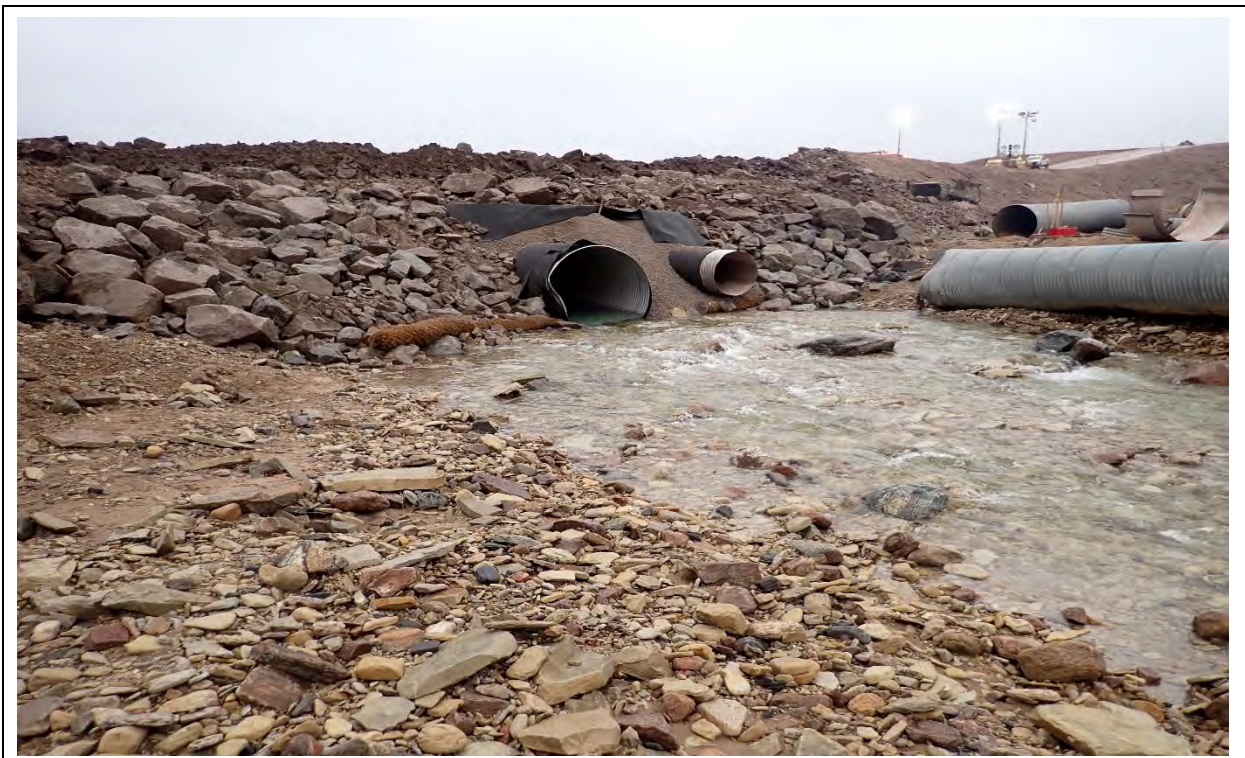
Photo 28. CV-049 downstream, culvert outlet completed with rock armouring of embankment
