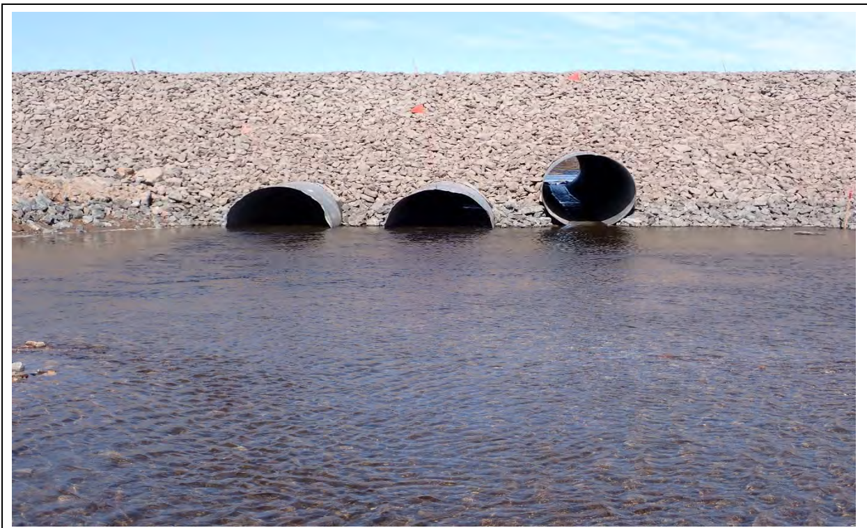
Photo 34. BG-04 downstream, culvert outlet after remedial construction.
