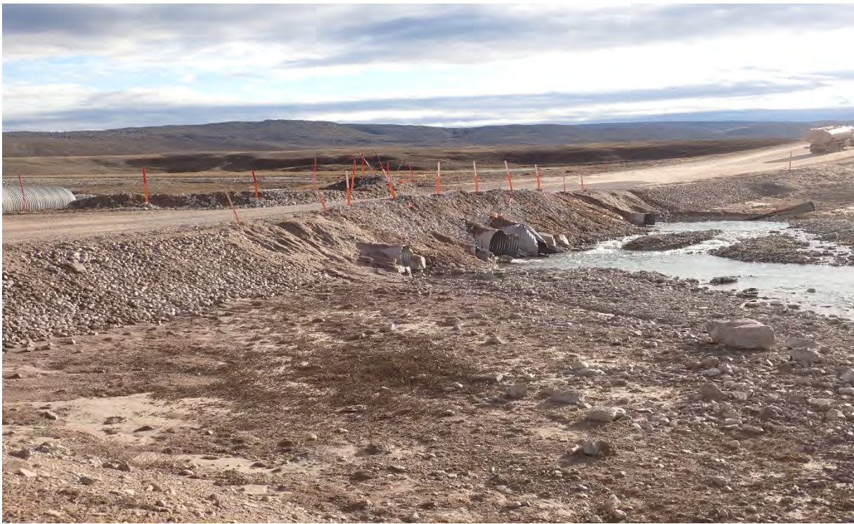
Photo 13. CV-078 downstream, re-established safe travel on the downstream lane of the road and re-armoured the embankment.
