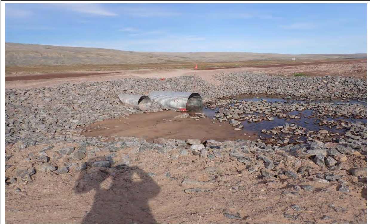
Photo 17. CV-059 upstream, culvert inlet apron after remedial construction.
