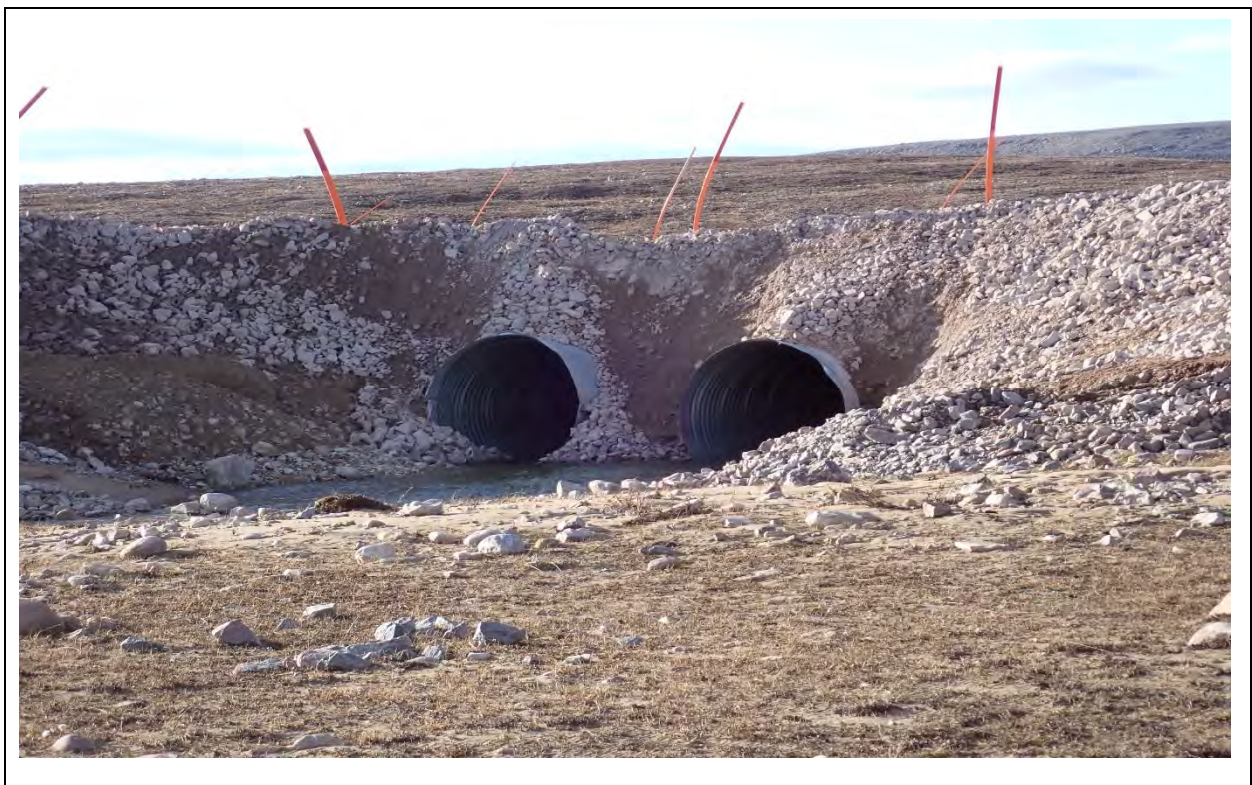
Photo 12. CV-078 upstream, culvert inlets detached and road embankment eroded during September rain event, repaired yet to be completed.
