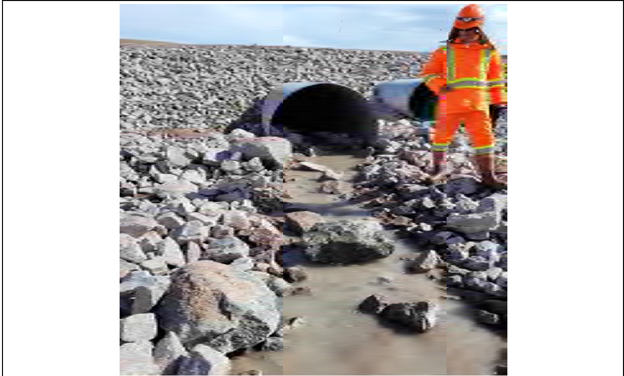
Photo 11. CV-102 downstream, culvert outlet apron rip rap thinned out to improve fish passage.
