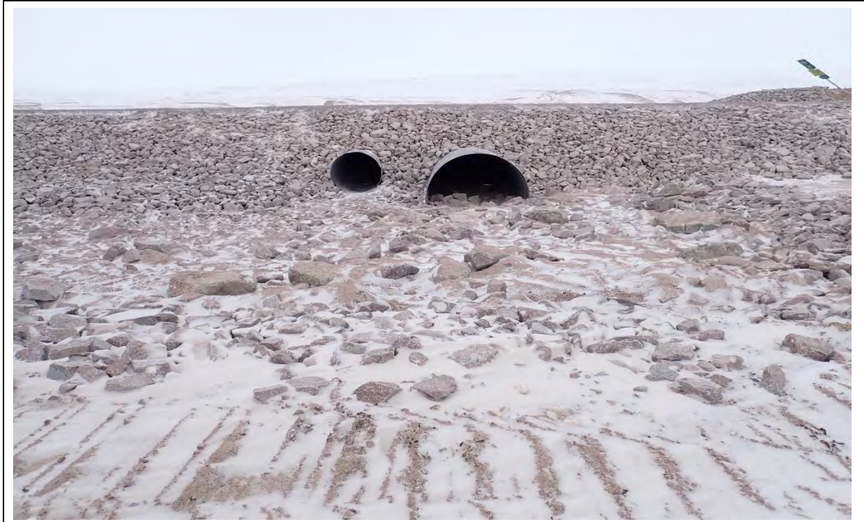
Photo 7. CV-102 upstream, culvert inlet after remedial construction.
