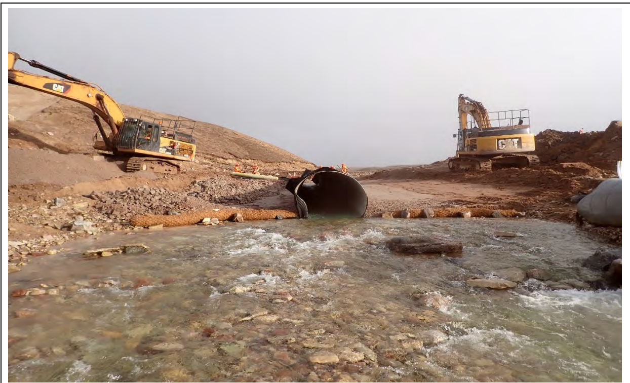
Photo 26. CV-049 downstream, coir logs placed during to protect culvert bedding material from erosion due to back eddy flow at culvert outlet.
