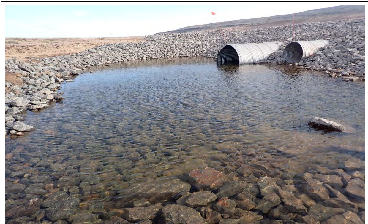
Photo 18. CV-059 downstream culvert outlet apron after remedial construction.
