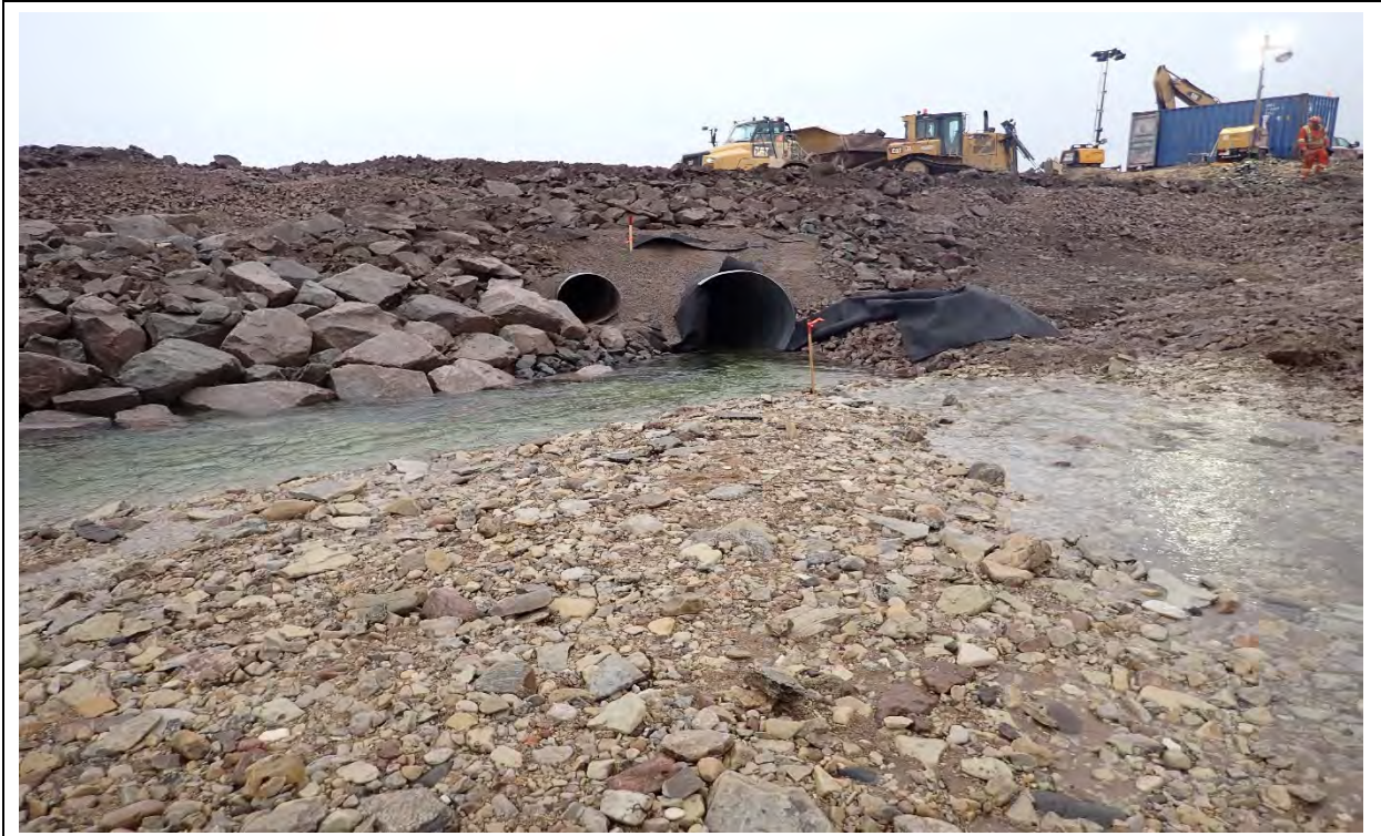
Photo 27. CV-049 upstream, culvert inlet completed with rock armouring of embankment
