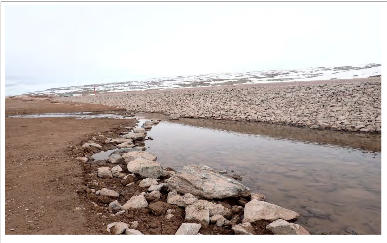
Photo 22. CV-057 downstream culvert outlet apron after remedial construction.
