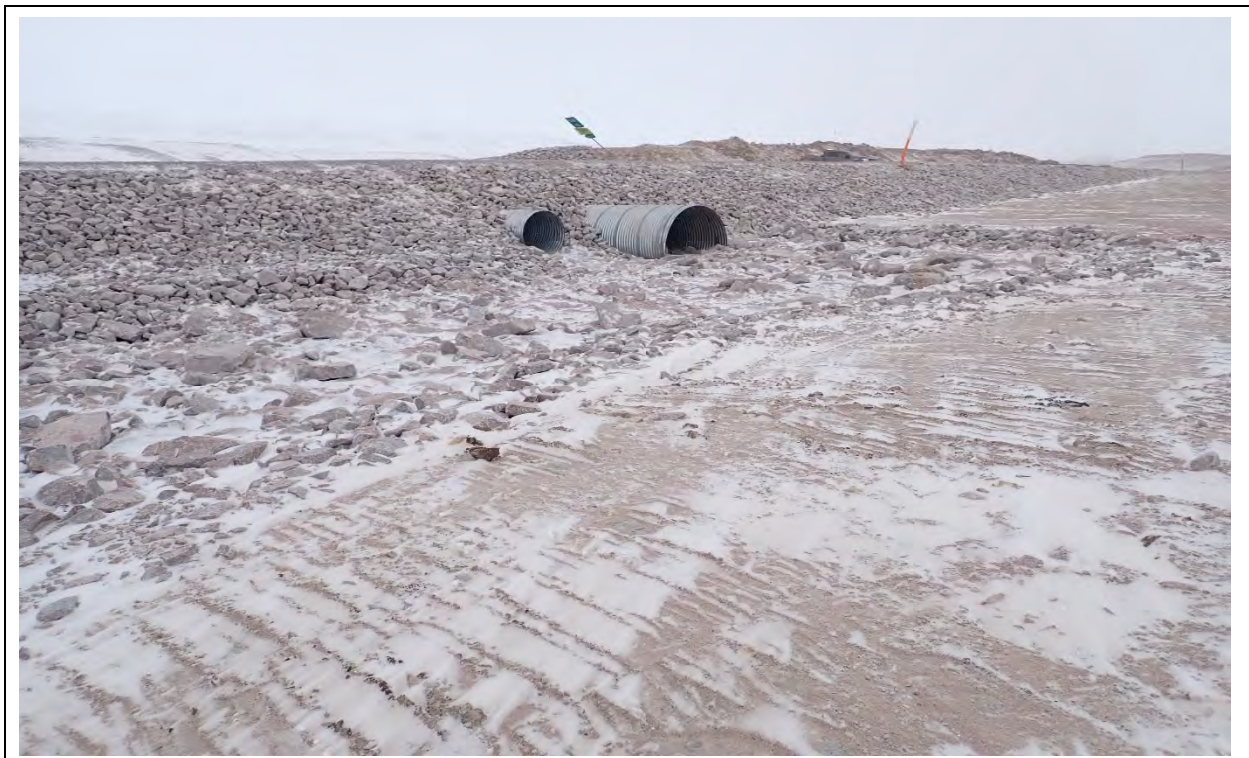
Photo 8. CV-102 upstream, culvert inlet apron after remedial construction.
