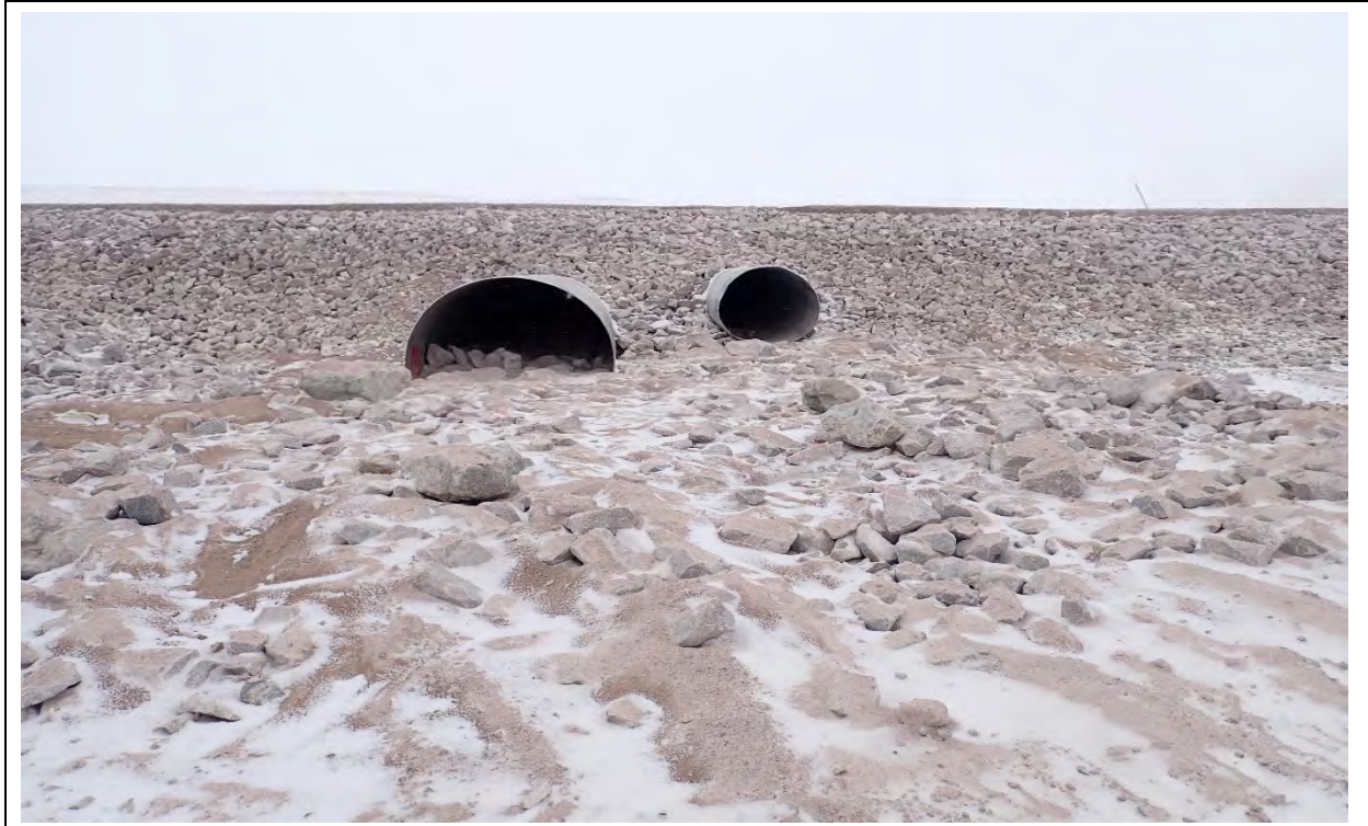
Photo 9. CV-102 downstream, culvert outlet after remedial construction.
