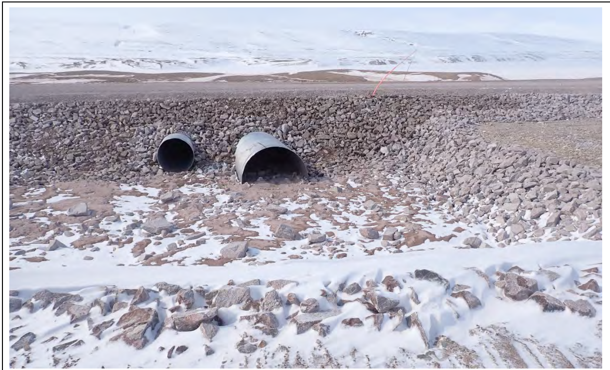
Photo 3. CV-106 upstream, culvert inlet after remedial construction.
