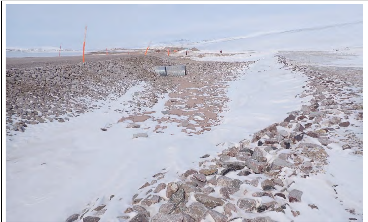
Photo 4. CV-106 upstream, culvert inlet apron after remedial construction.
