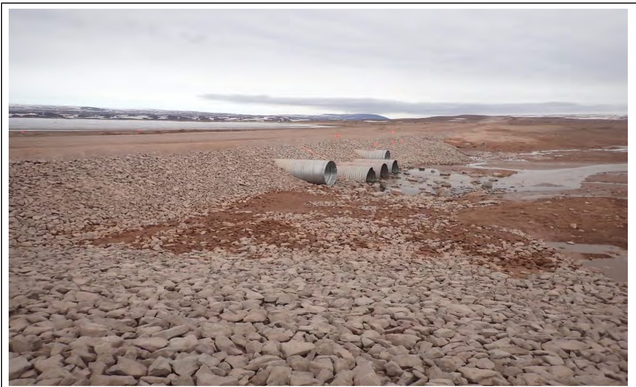
Photo 30. CV-216 upstream, culvert inlet apron after remedial construction.
