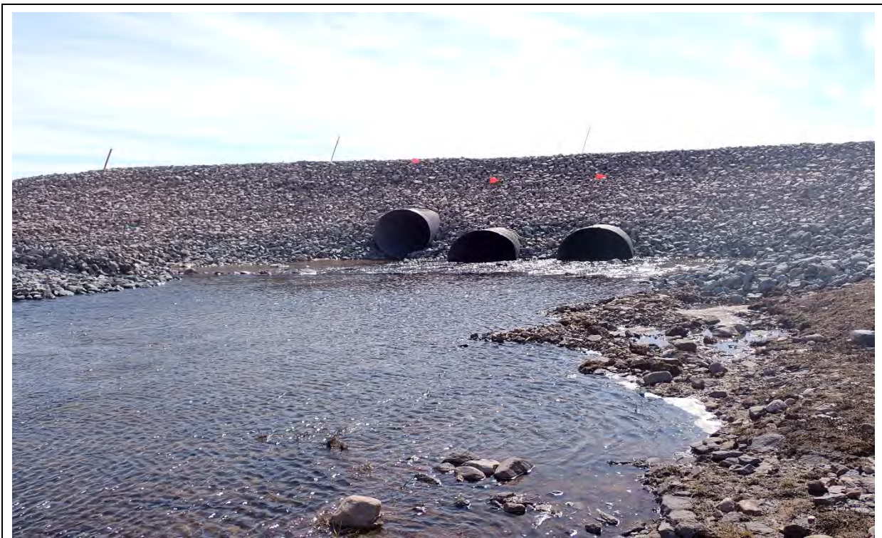
Photo 32. BG-04 upstream, culvert inlets after remedial construction.
