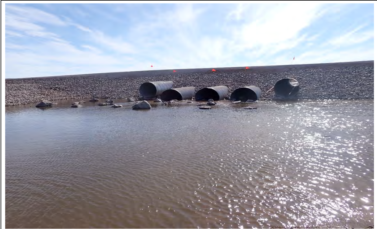
Photo 31. CV-216 downstream, culvert outletapron after remedial construction.
