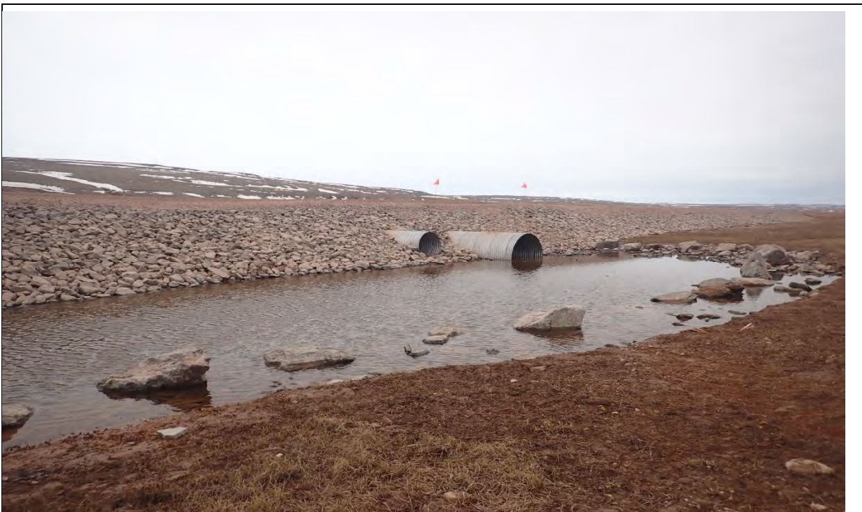
Photo 20. CV-057 upstream culvert inlet apron after remedial construction.
