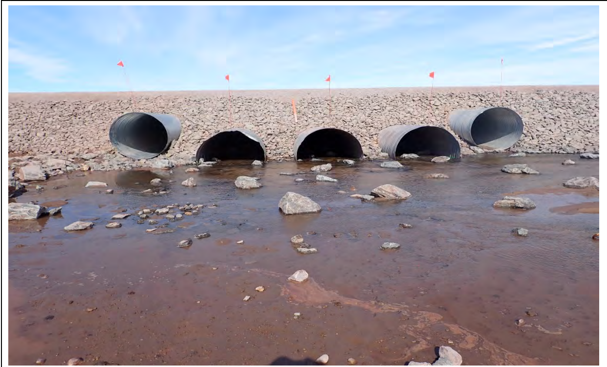
Photo 29. CV-216 upstream, culvert inlets after remedial construction.
