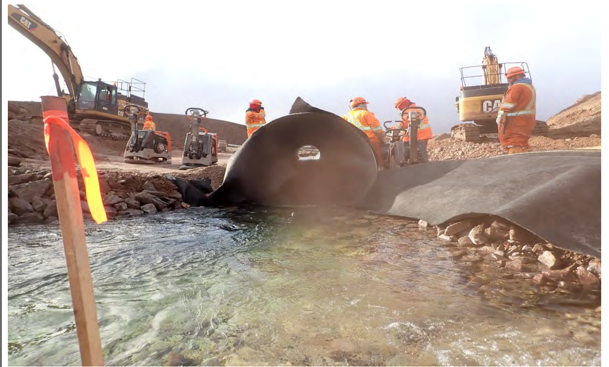
Photo 25. CV-049 upstream, geotextile placed behind rock armouring to prevent culvert bedding material from entering watercourse during re-construction
