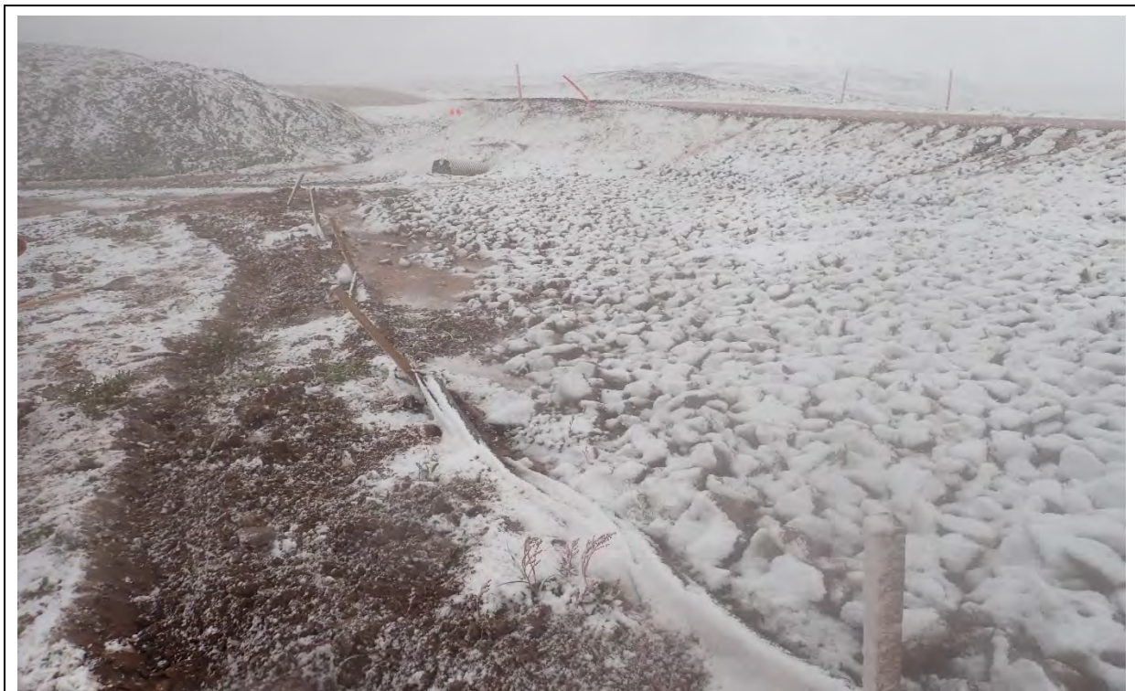
Photo 38. CV-224 downstream, silt fence in disrepair.
