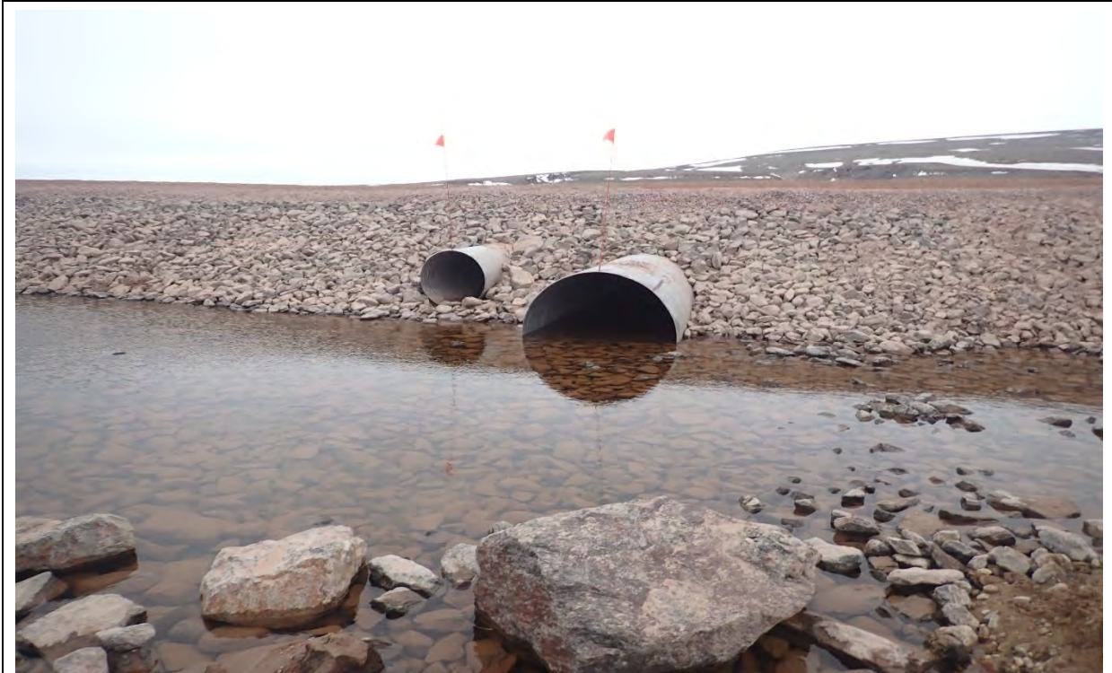
Photo 19. CV-057 upstream culvert inlet after remedial construction.
