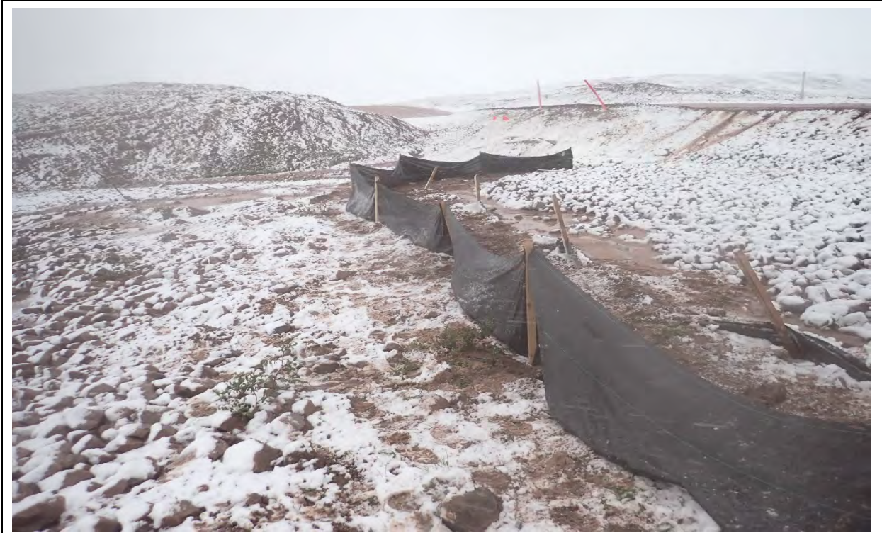
Photo 39. CV-224 downstream, silt fence replaced.
