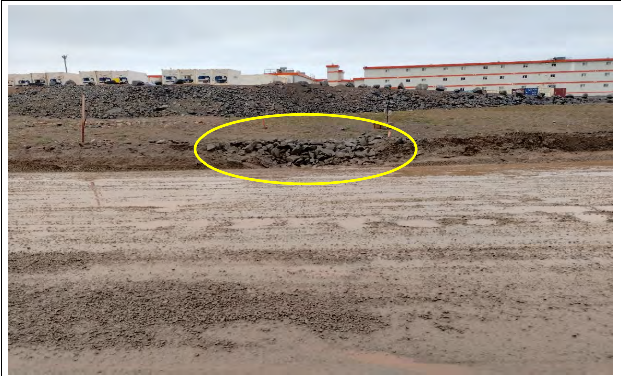
Photo 45. CV-186 downstream, rock armouring of roadside berm.
