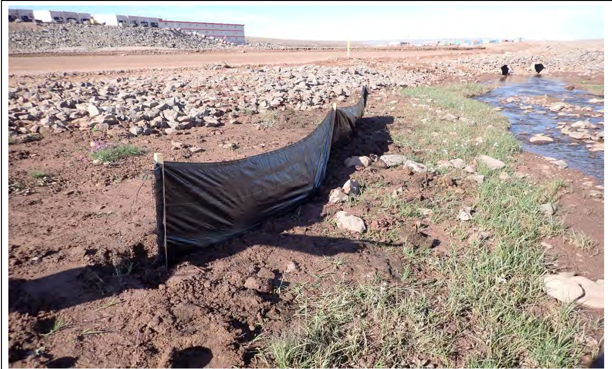
Photo 43. CV-186 upstream, silt fence along south bank replaced.
