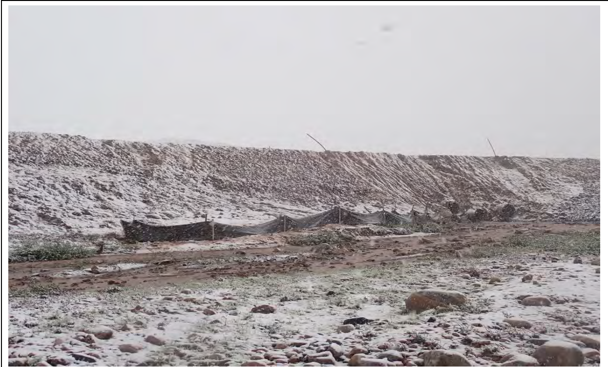
Photo 41. BG-01 upstream, silt fence replaced.
