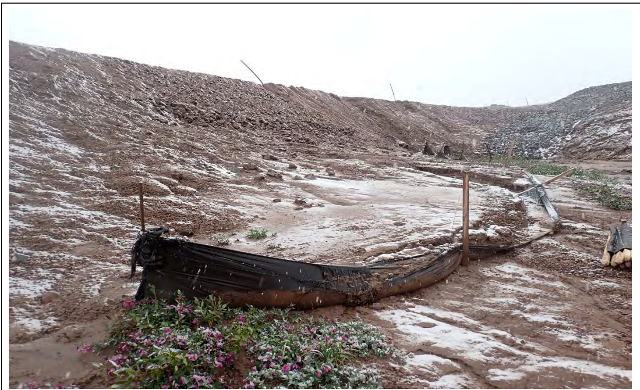
Photo 40. BG-01 upstream, silt fence in disrepair.
