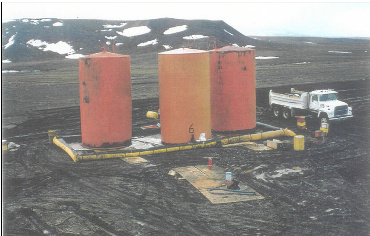
Figure 4-3-2 Original Berm around the Runway Tanks in 1996
