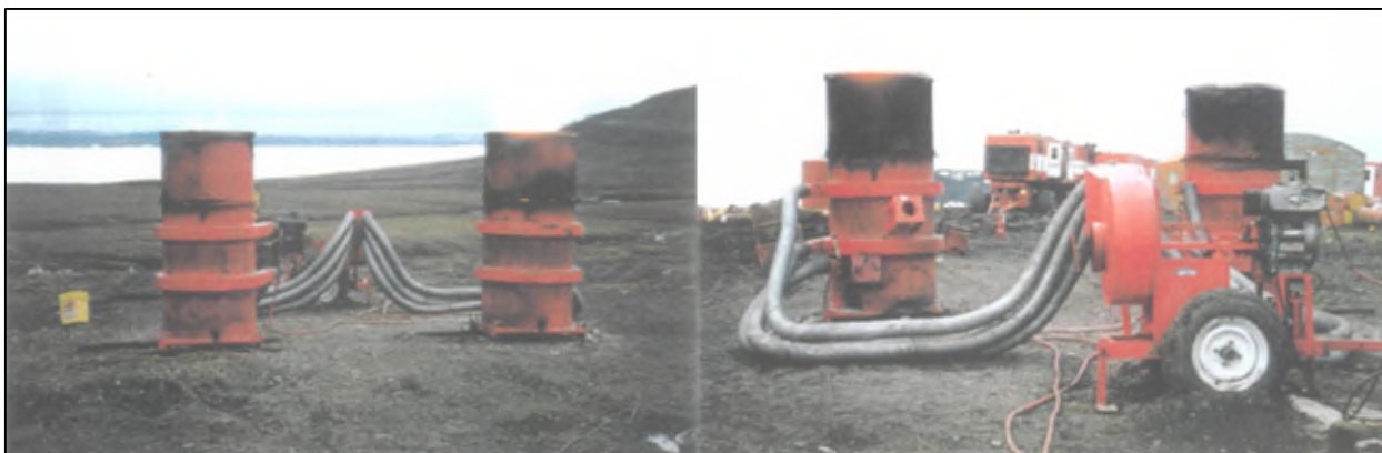
Figure 4-1: Previous Fuel Incineration System in Operation (1996).
