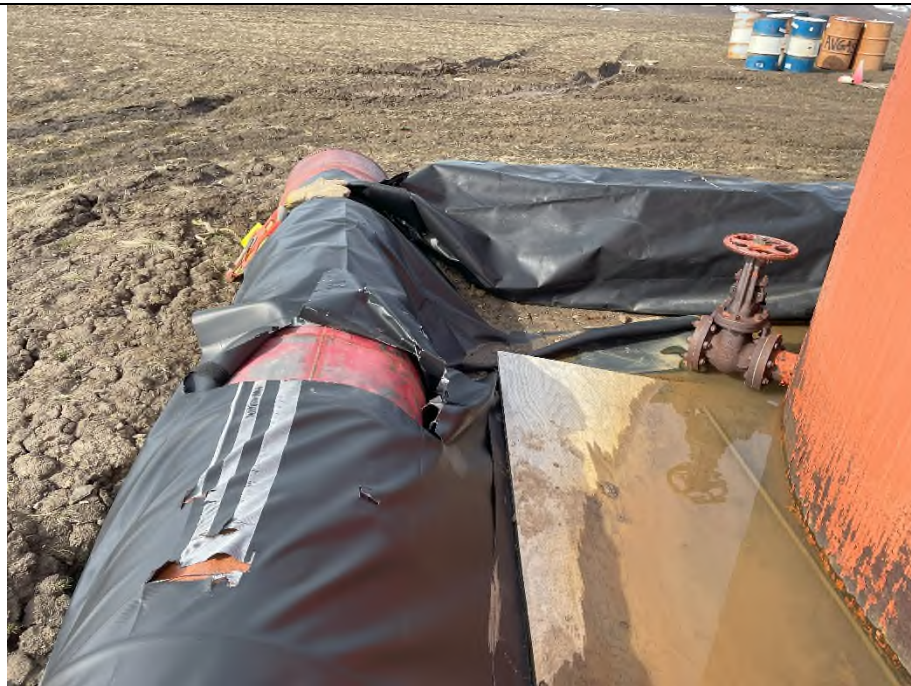
Photo 4: Condition of the berm liner, note rips and tears in corner, view Northwest. (July 6, 2024)
