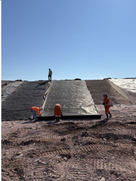
Photo 4 Replacing Geotextile
