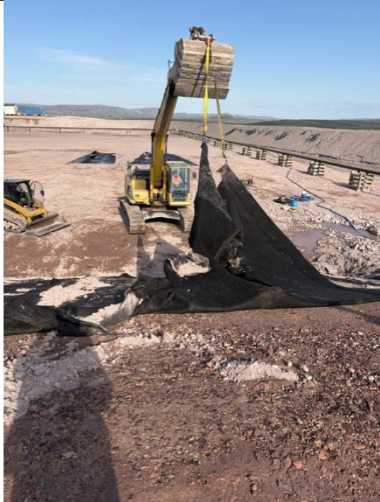
Photo 3: Removing Damaged Liner
