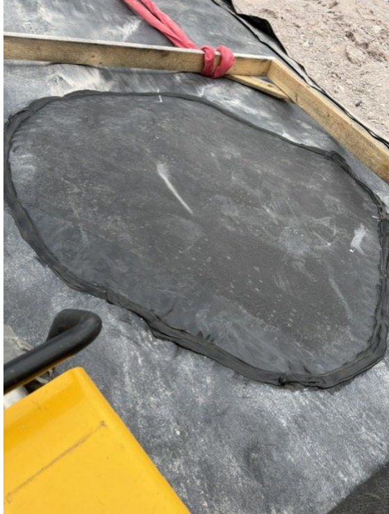
Photo 2: Exposed HDP Liner NW Corner was fixed and tested
