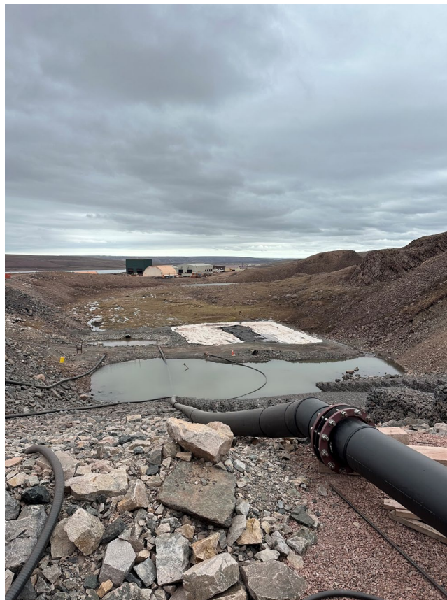
Photo 10 – Tundra below KM105 Dam (June 18 th , 2025).
