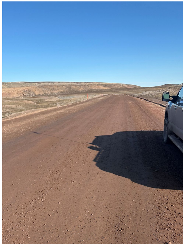
Photo 20 – Tote Road after application of calcium chloride and water (June 19 th , 2025).
