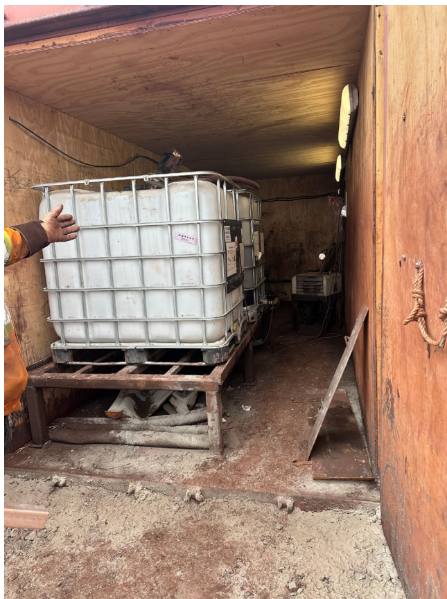
Photo 12 – Crusher Pond Totes for dust suppression (June 18 th , 2025).
