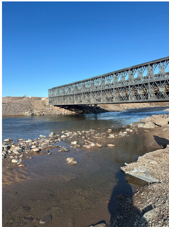
Photo 18 – KM97 Bridge crossing (June 19 th , 2025).
