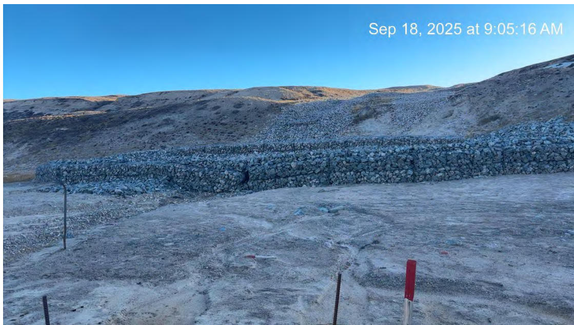
Photo 22 – Gabion wall at Camp Lake (September 18, 2025).
