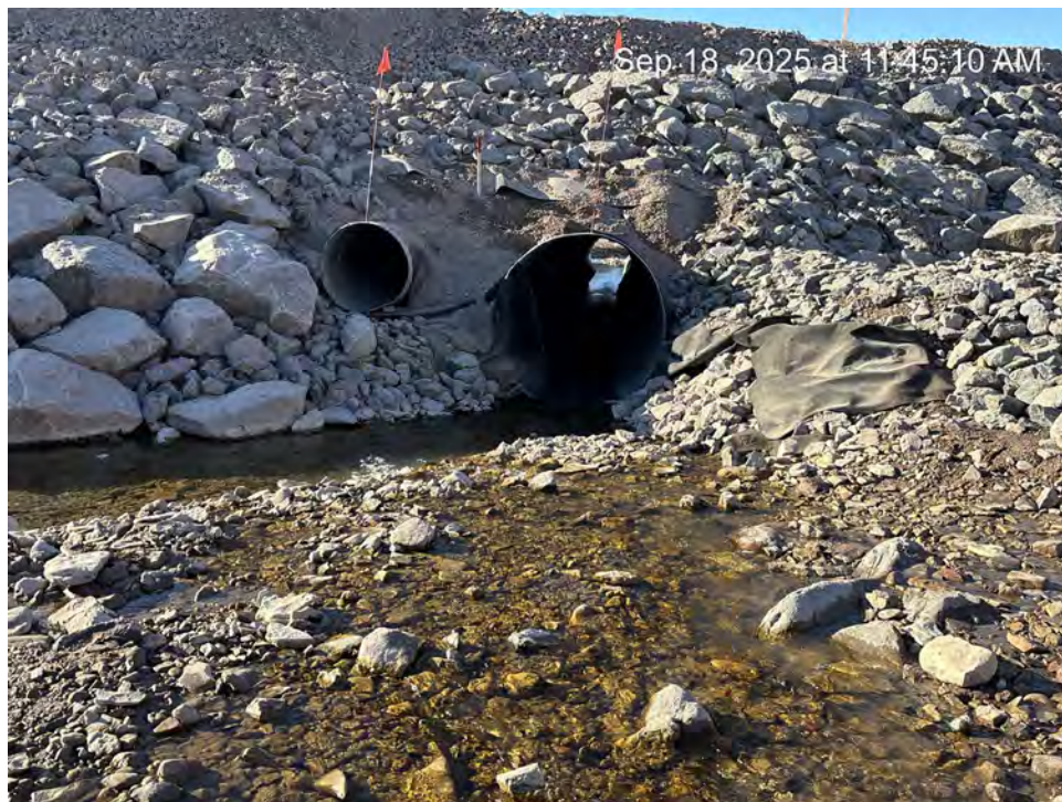
Photo 42 – Culverts at KM64 (September 18, 2025).
