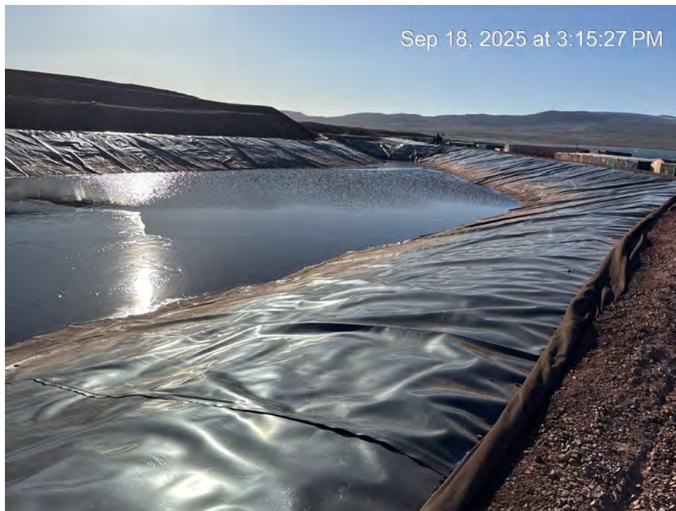
Photo 52 – West stockpile discharge pond (September 18, 2025).
