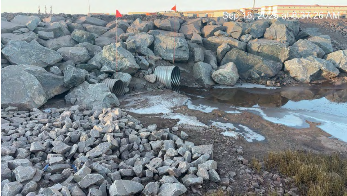
Photo 19 – CV187 replaced in June 2025 (September 18, 2025).
