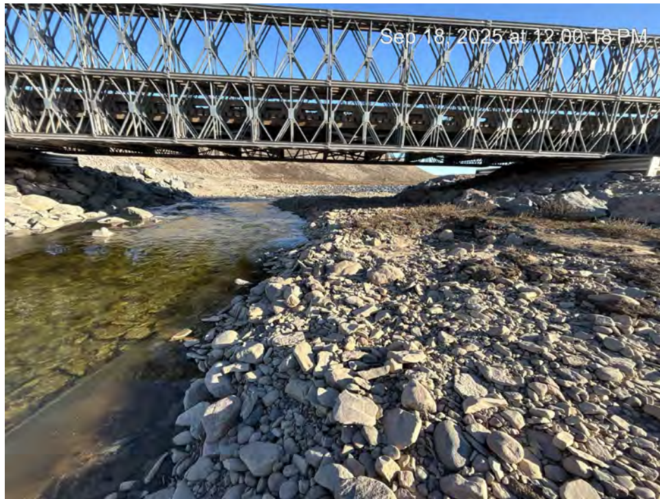
Photo 46 – Clear, flowing water at KM63 bridge (September 18, 2025).
