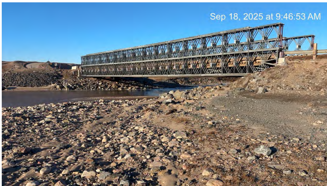
Photo 28 – Reinforced bridge at KM97 (September 18, 2025).
