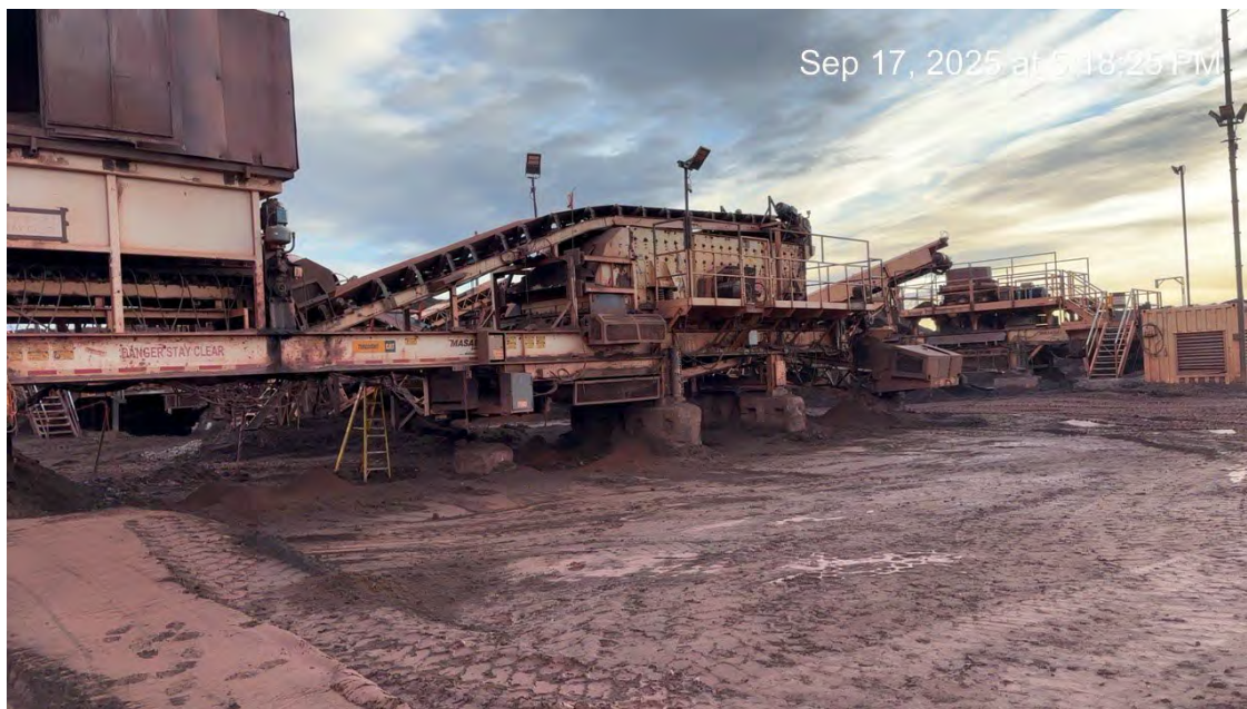
Photo 18 – Crusher at the crusher pad (September 17, 2025).
