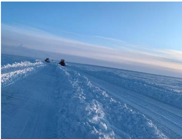
Figure 8-3: Establishing Ice Road Alignment after Profiling
