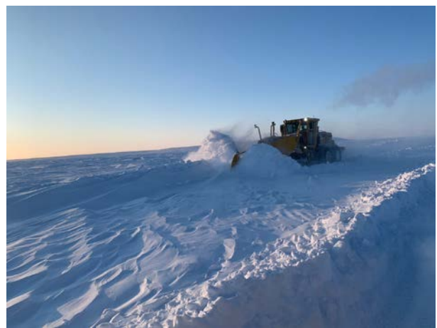
Figure 8-4: 160M Grader Plowing Ice Road Alignment
