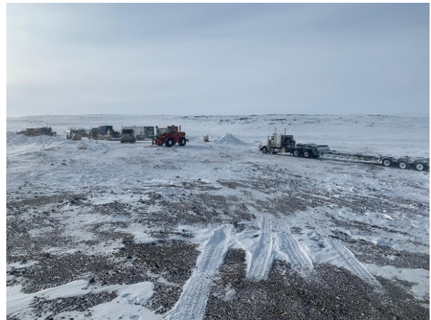
Figure 8-22: Portage 55 Demobilization Activities
