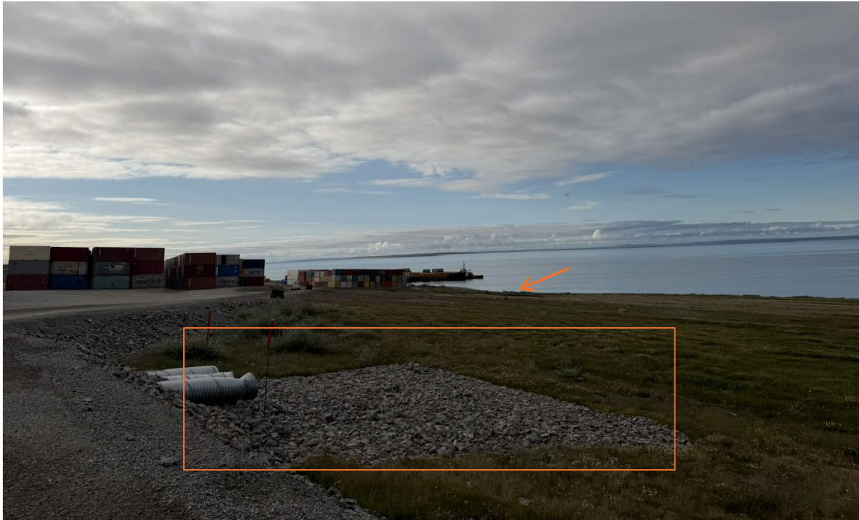
Photo 4: Riprap and silt fences implemented to mitigate erosion and control sediment runoff
