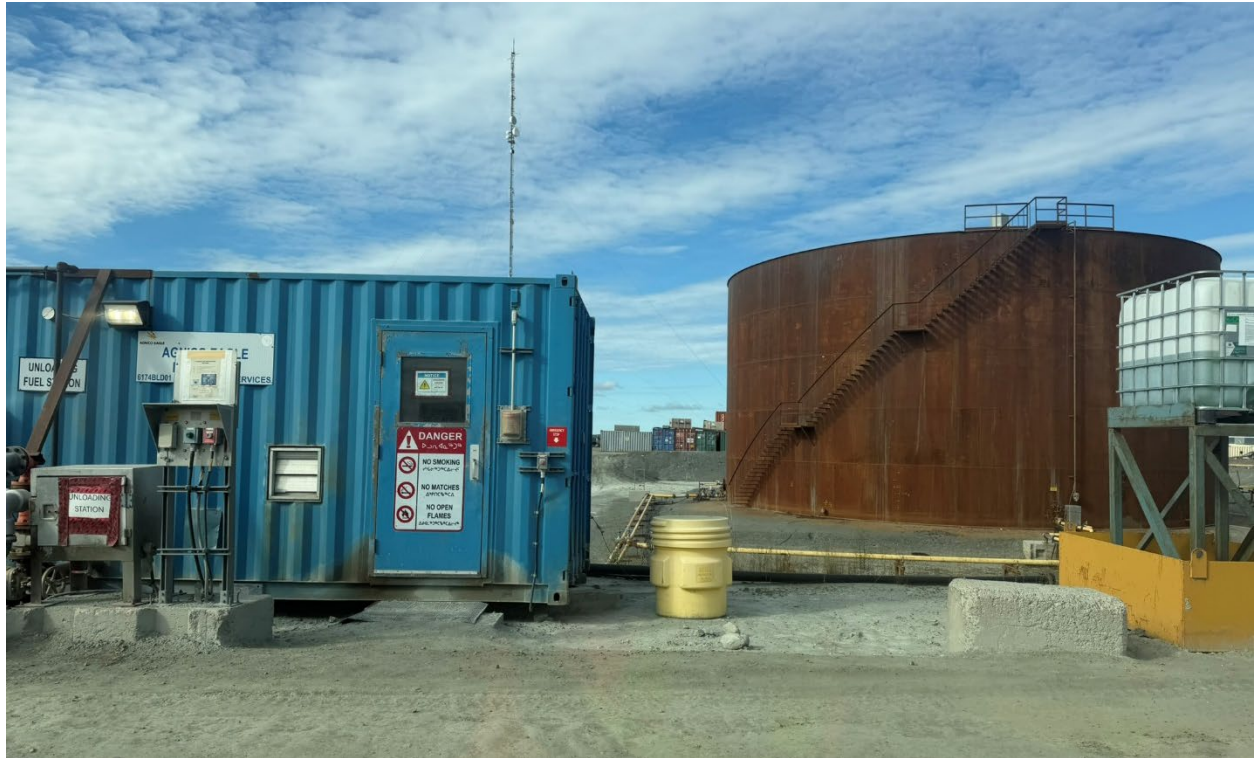
Photo 56: On site tank farm, and fueling station
