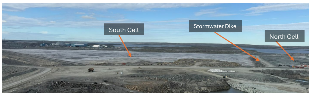
Photo 48: Tailings Storage Facility - South Cell 8
