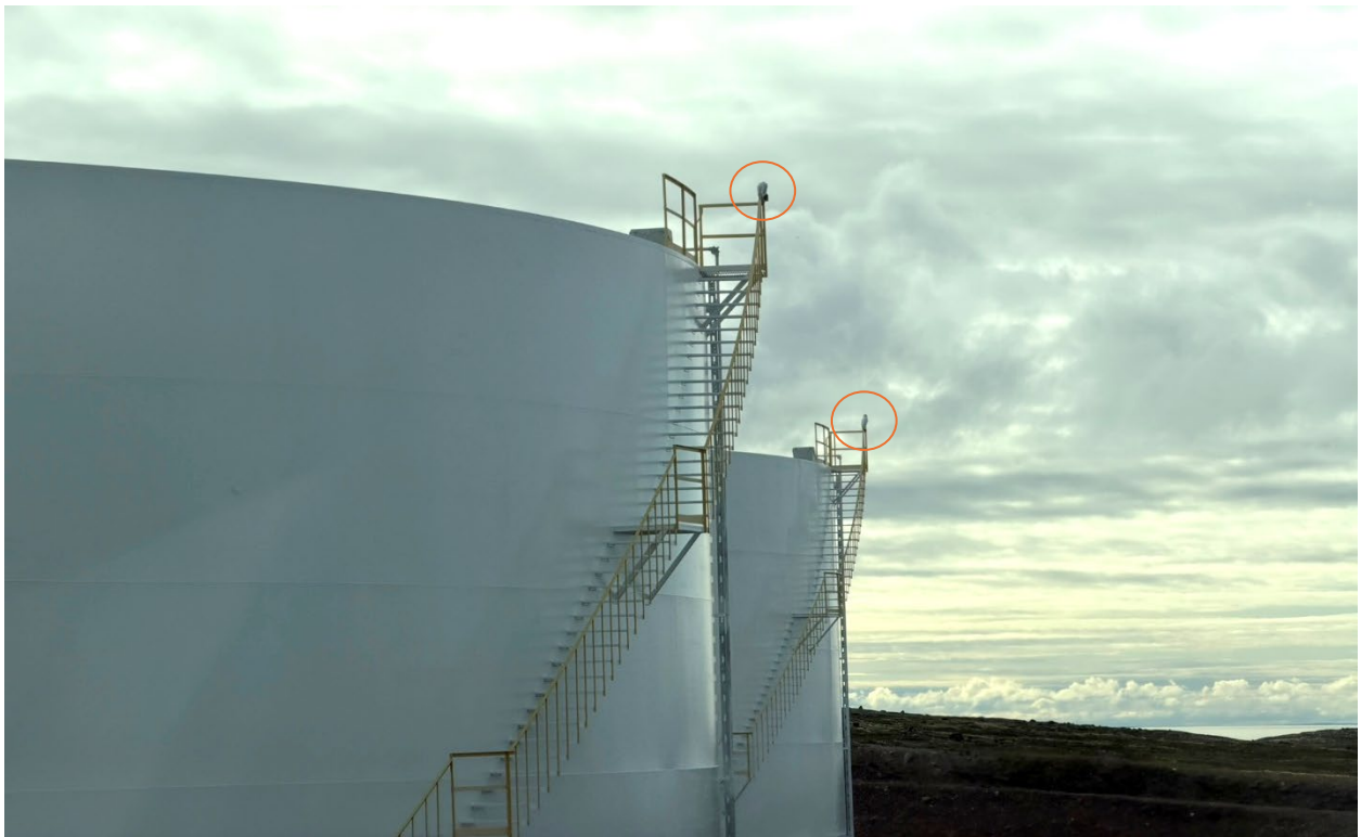
Photo 13: Bird/raptor deterrent on fuel tanks
