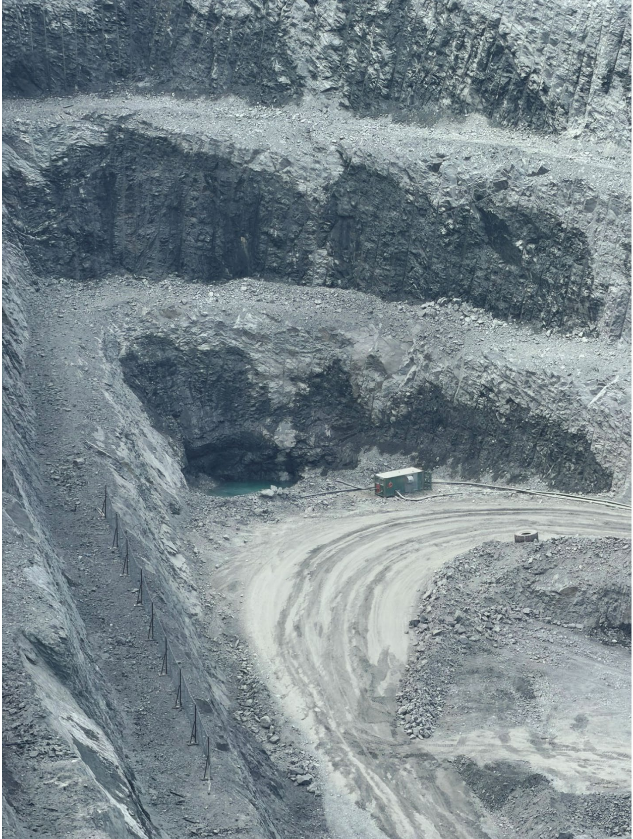
Photo 83: Pool of water at the base of the WT Pit
