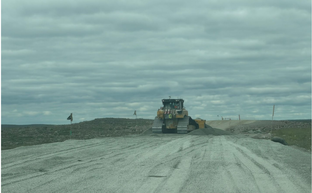
Photo 69: Road maintenance activities on the WTHR
