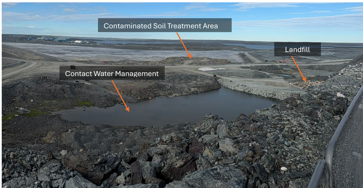
Photo 51: Waste management area, westward view from atop Portage Rock Storage Facility
