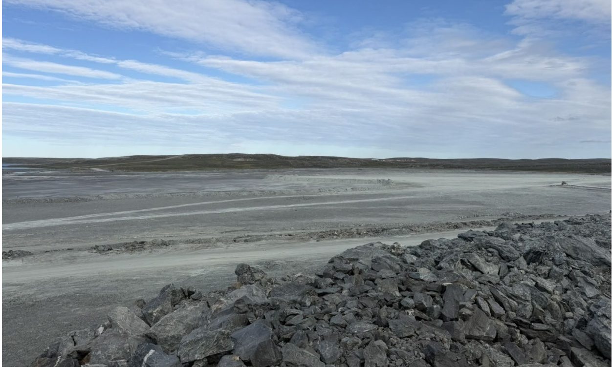
Photo 50: Tailings Storage Facility – North Cell, with active NAG capping underway as part of progressive reclamation activities
