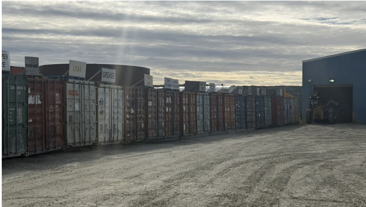
Photo 54: Composter Building and HAZMAT storage seacans 9
