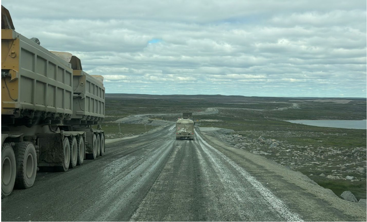
Photo 75: Active application of calcium chloride dust suppressant along the WTHR
