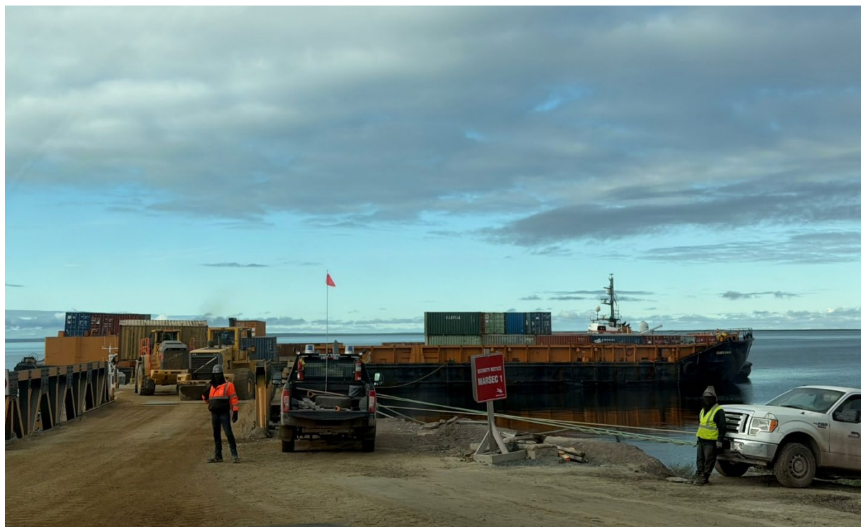
Photo 1: Dock and barge landing area
