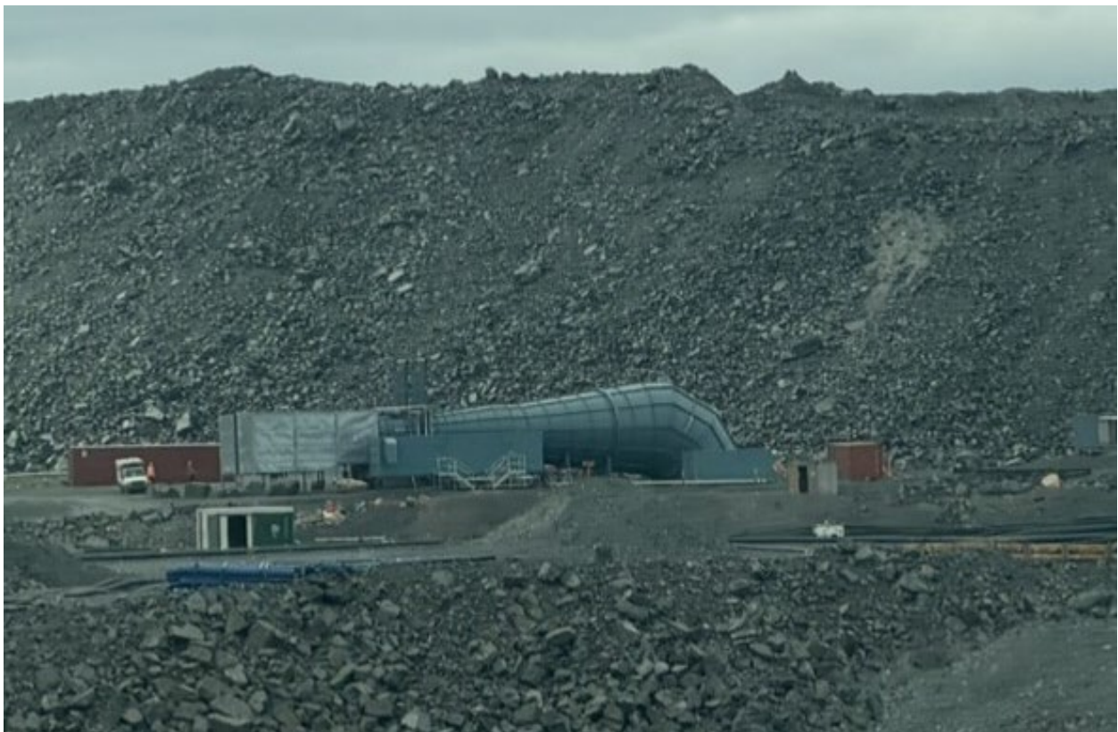
Photo 87: Vent raise to support underground mining
