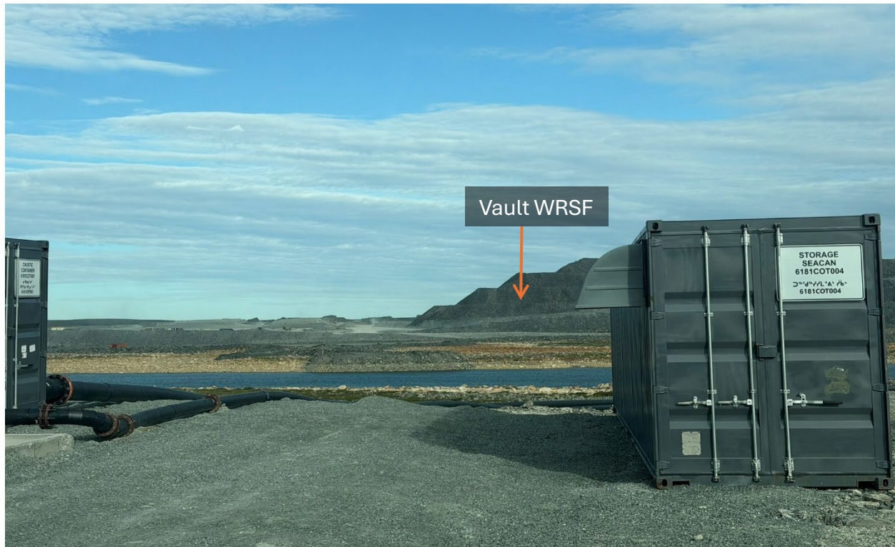
Photo 38: Vault Attenuation Pond 3
