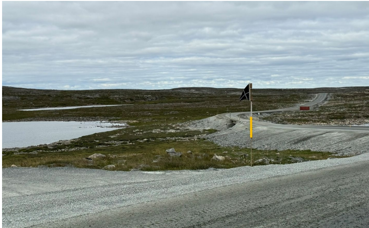
Photo 62: Bridge crossing at WTHR KM 102 and adjacent emergency response seacan
