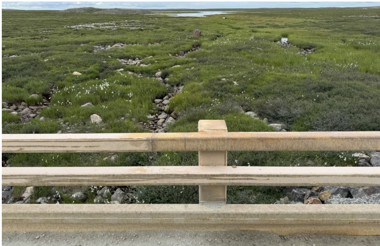
Photo 23: Close-up view of containment plates
