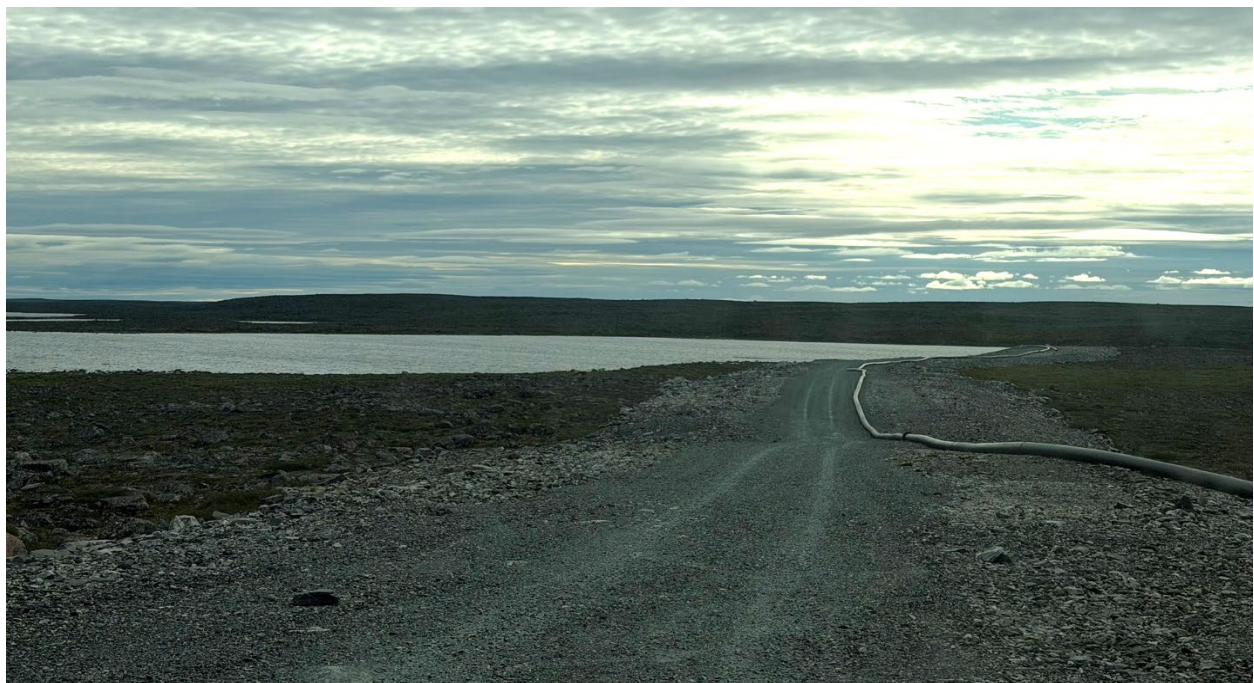
Photo 39: Wally Lake and Discharge Line
