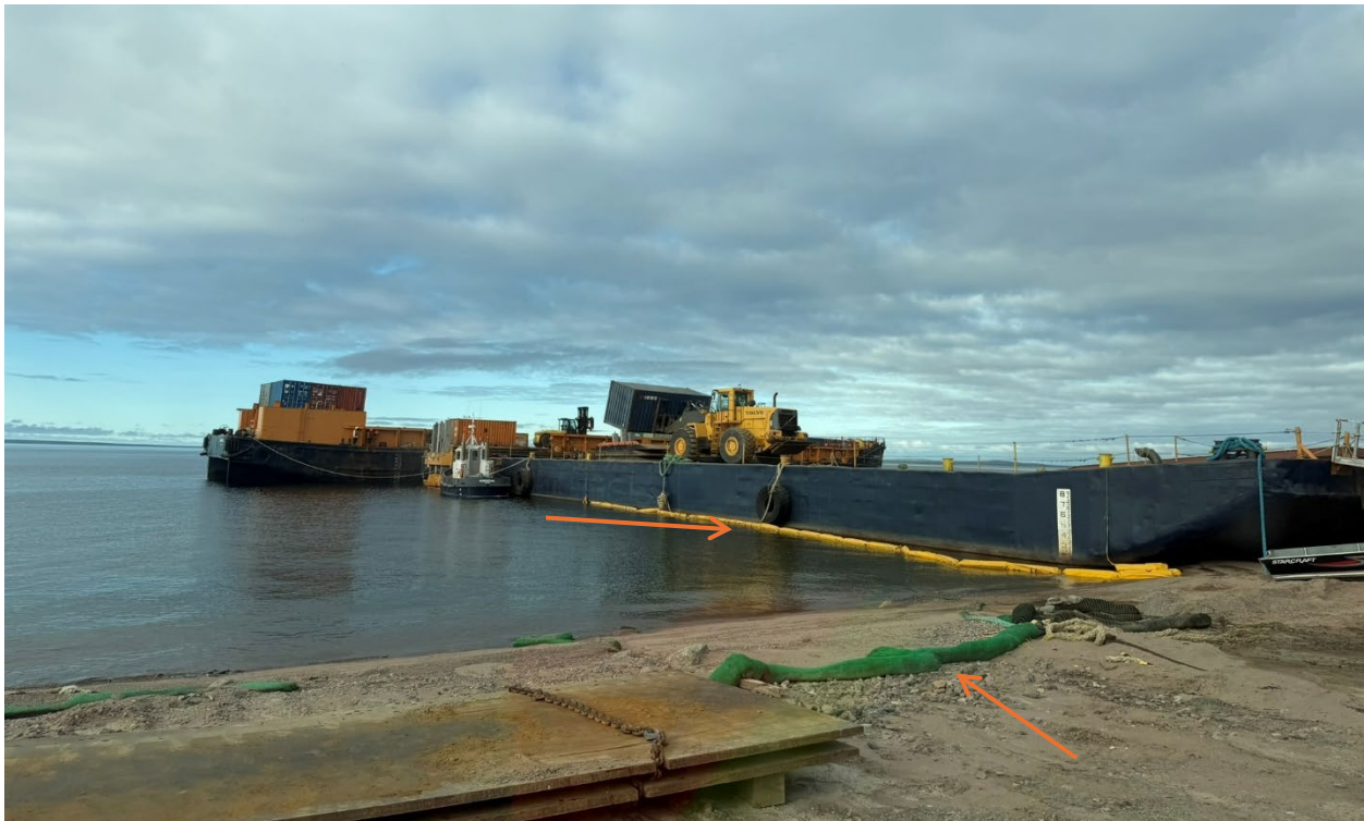
Photo 3: Erosion control and spill contingency measures at the barge landing, including silt socks along the shoreline and a floating containment boom deployed around the barge
