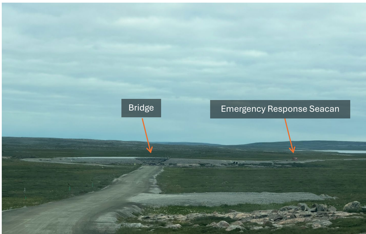
Photo 15: Distant view of the KM 8 bridge and nearby emergency response seacan
