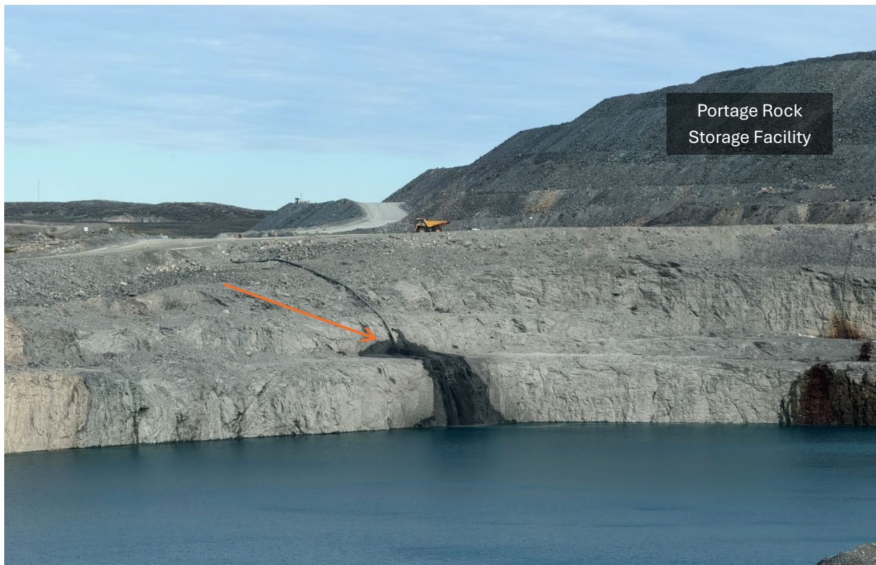
Photo 43: Active in-pit tailings deposition at Portage Pit A
