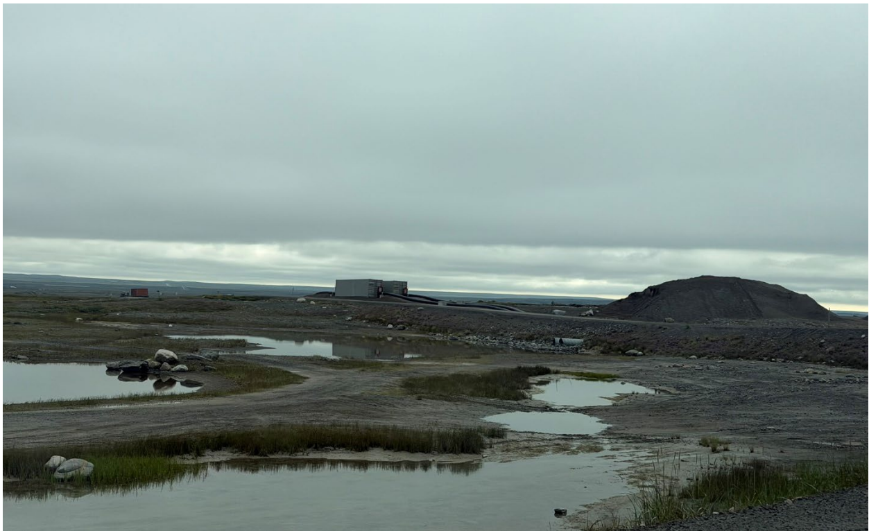
Photo 17: Distant view of air pressure relief sea cans and exposed waterlines at KM 4
