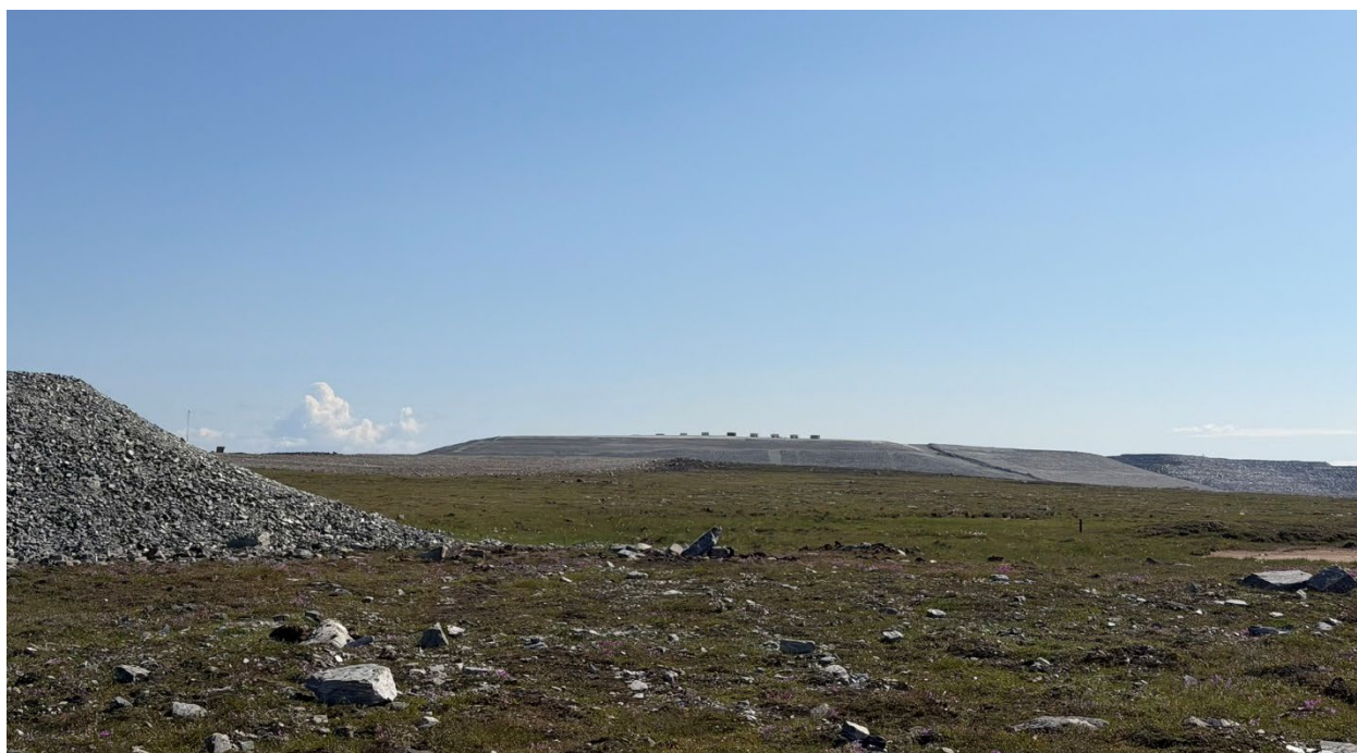
Photo 65: Distant view of Tailings Storage Facility (TSF) 5
