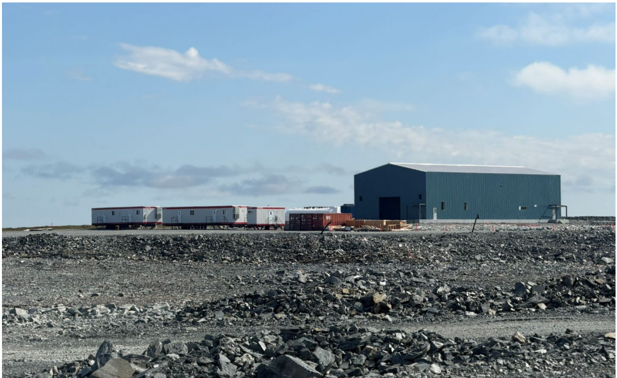
Photo 38: Pump Service Shop
