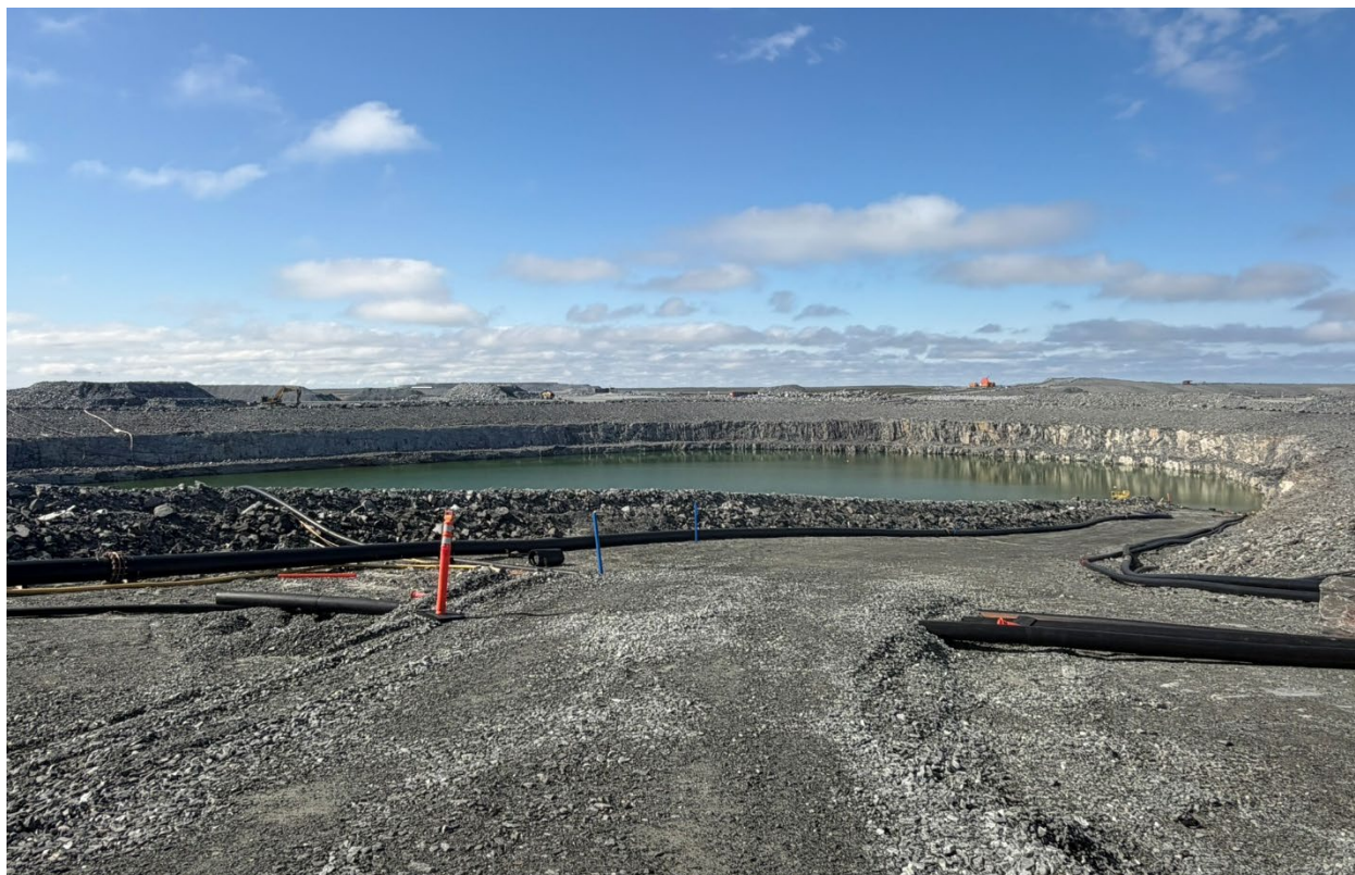
Photo 52: Tiriganiaq 02 (TIRI 02), facing south, currently used for storage of saline contact water from the underground mine
