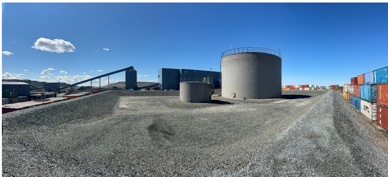
Photo 87: Fuel Tanks within secondary containment at onsite 6M Fuel Tank Farm
