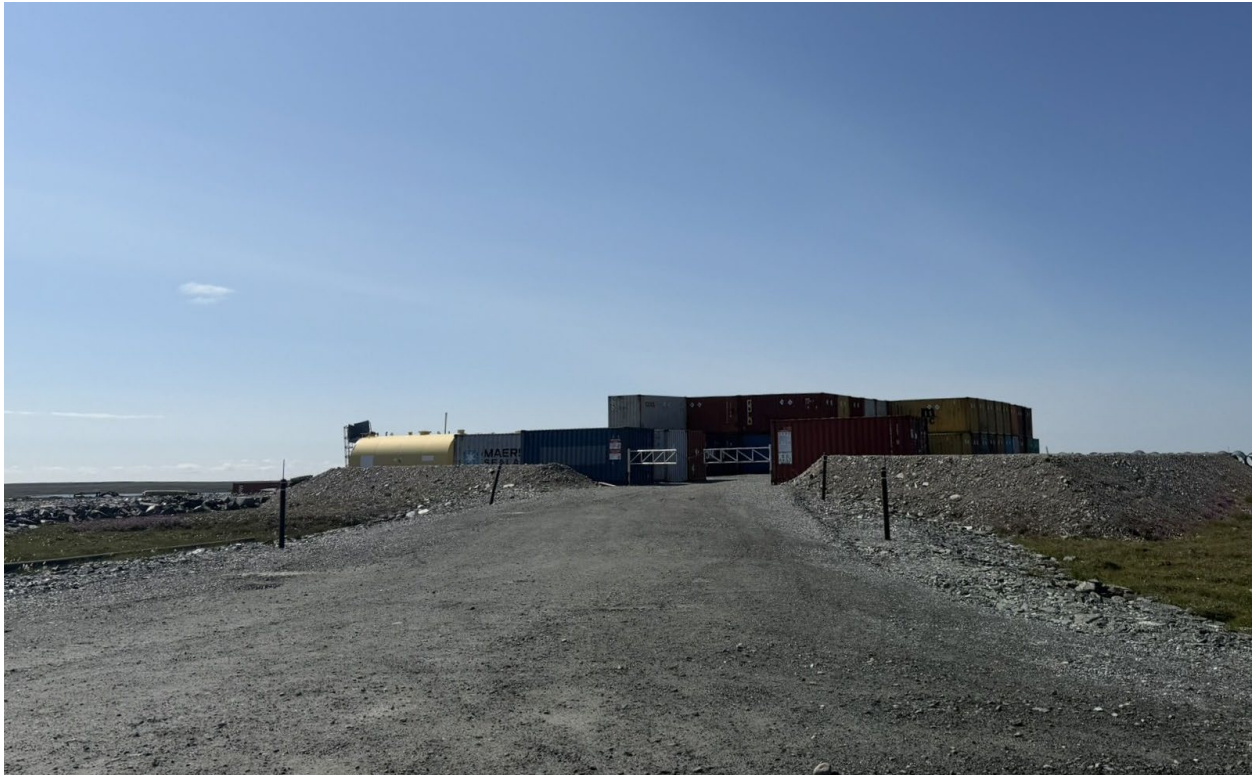
Photo 58: Cyanide Storage Tanks
