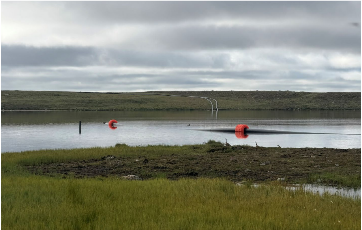
Photo 34: Dewatering infrastructure in place on Lake A6
