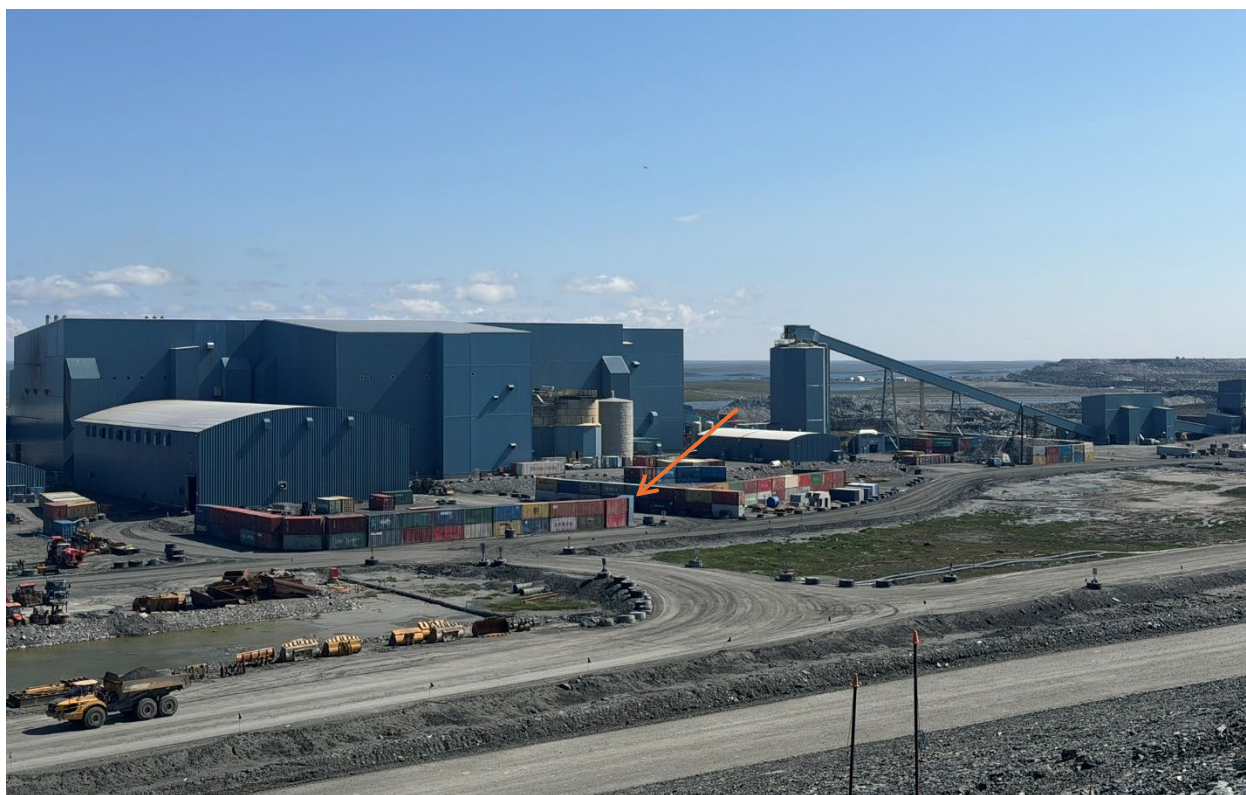
Photo 57: Processing Plant, with seacans stacked two high to form a screening wall 4
