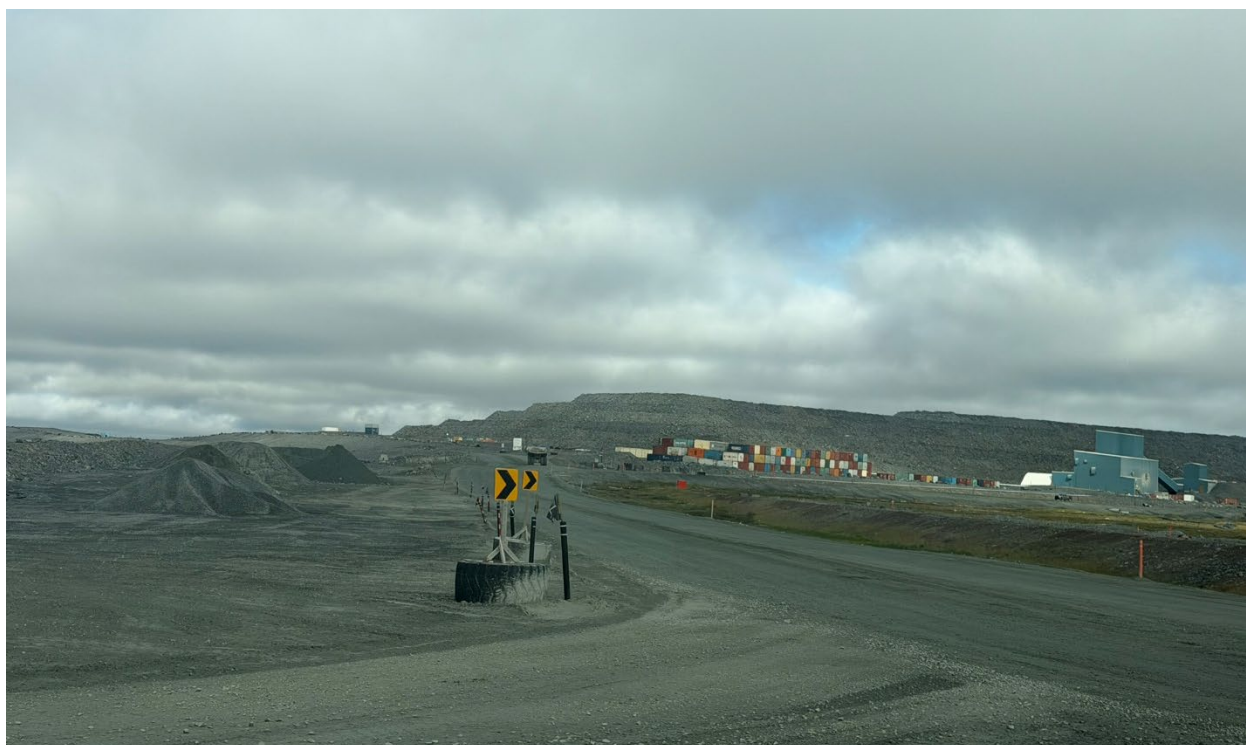
Photo 53: Distant view of WRSF 1
