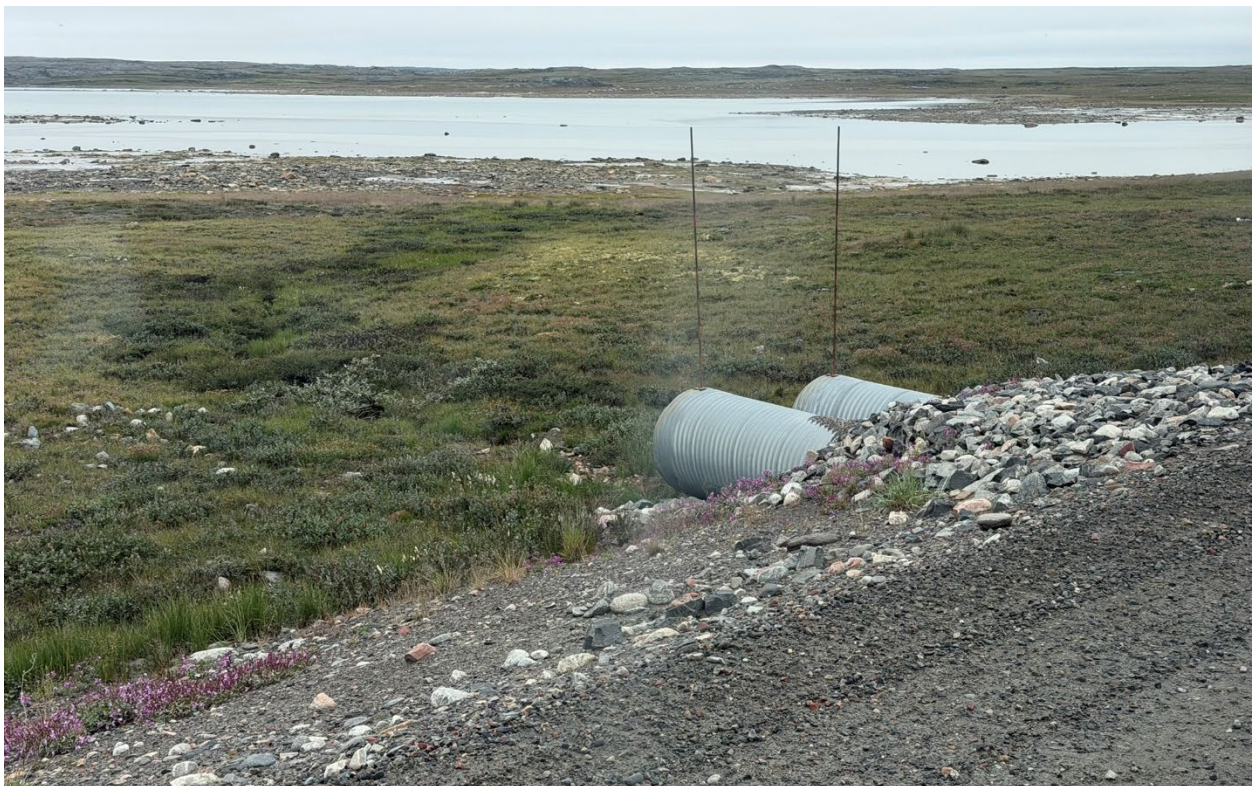
Photo 15: Twin culvert outlets at KM 2.5
