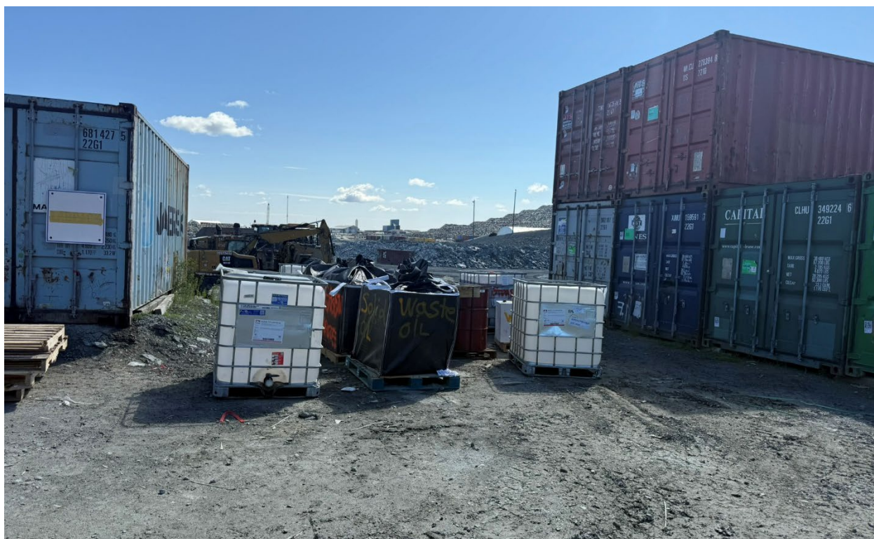
Photo 93: Hazardous material totes and bulk bags staged outside of the seacans without secondary containment
