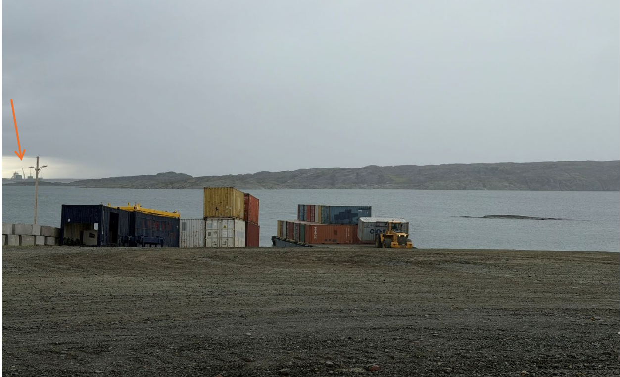
Photo 12: Loaders staging seacans on the dock, with the vessel visible in the background
