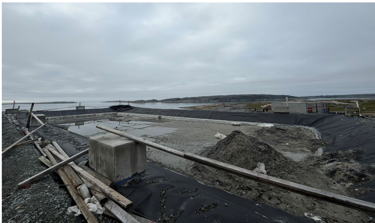
Photo 9: Temporary contact water management pond at Itivia, which is planned to be decommissioned as the works for HDD is over
