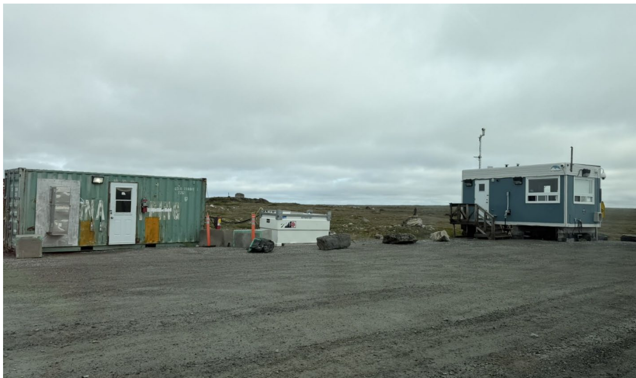
Photo 26: Access control gatehouse at KM 12, where road users are required to check-in upon entry
