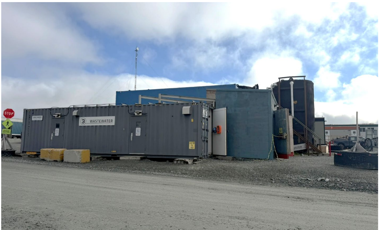
Photo 103: Sewage Treatment Plant to treat wastewater from the accommodation complex
