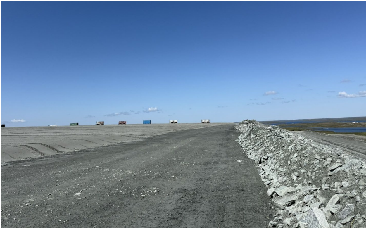
Photo 67: Seacans stacked on top of the Tailings Storage Facility to act as wind fences 6
