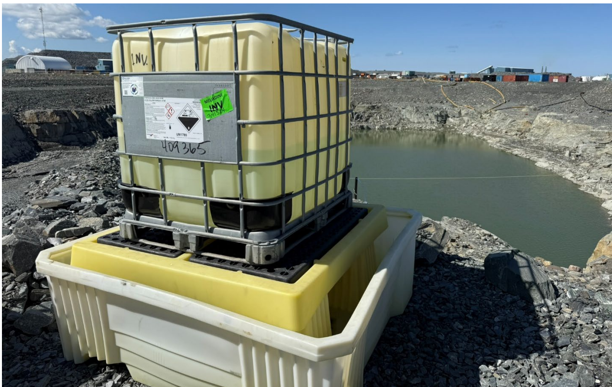
Photo 73: Hydrochloric acid tote within secondary containment near SP1 for pH adjustment ahead of RO treatment
