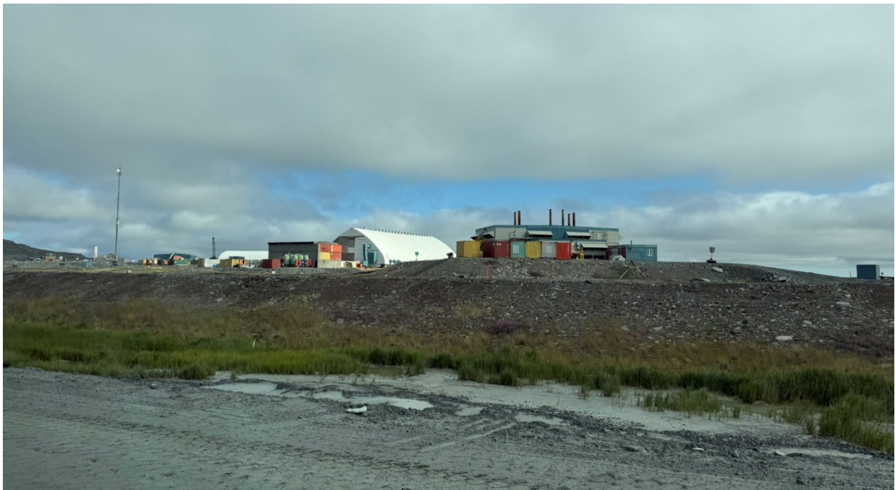
Photo 49: Vent Raise infrastructure supporting underground mine
