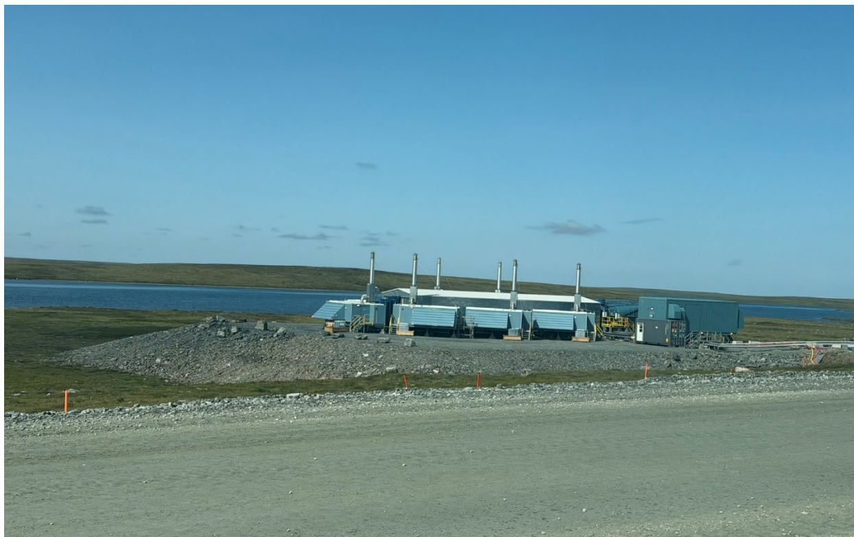
Photo 41: West Vent Raise infrastructure supporting underground mine
