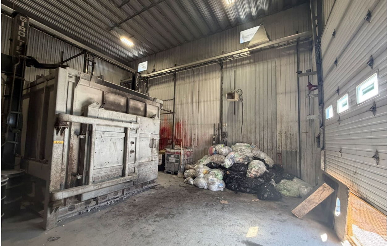
Photo 90: Bagged waste accumulated within the incinerator building
