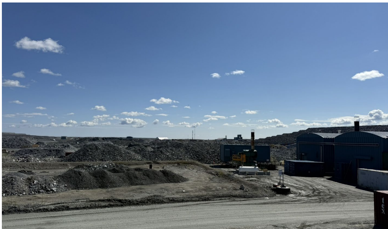
Photo 95: Landfarm cells to treat contaminated soil 12
