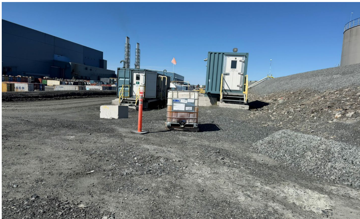
Photo 88: 6M Pumping Station, with the DEF storage tank located outside secondary containment
