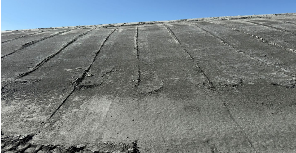
Photo 66: Eastern perimeter slope of the Tailings Storage Facility, viewed from the TSF access road
