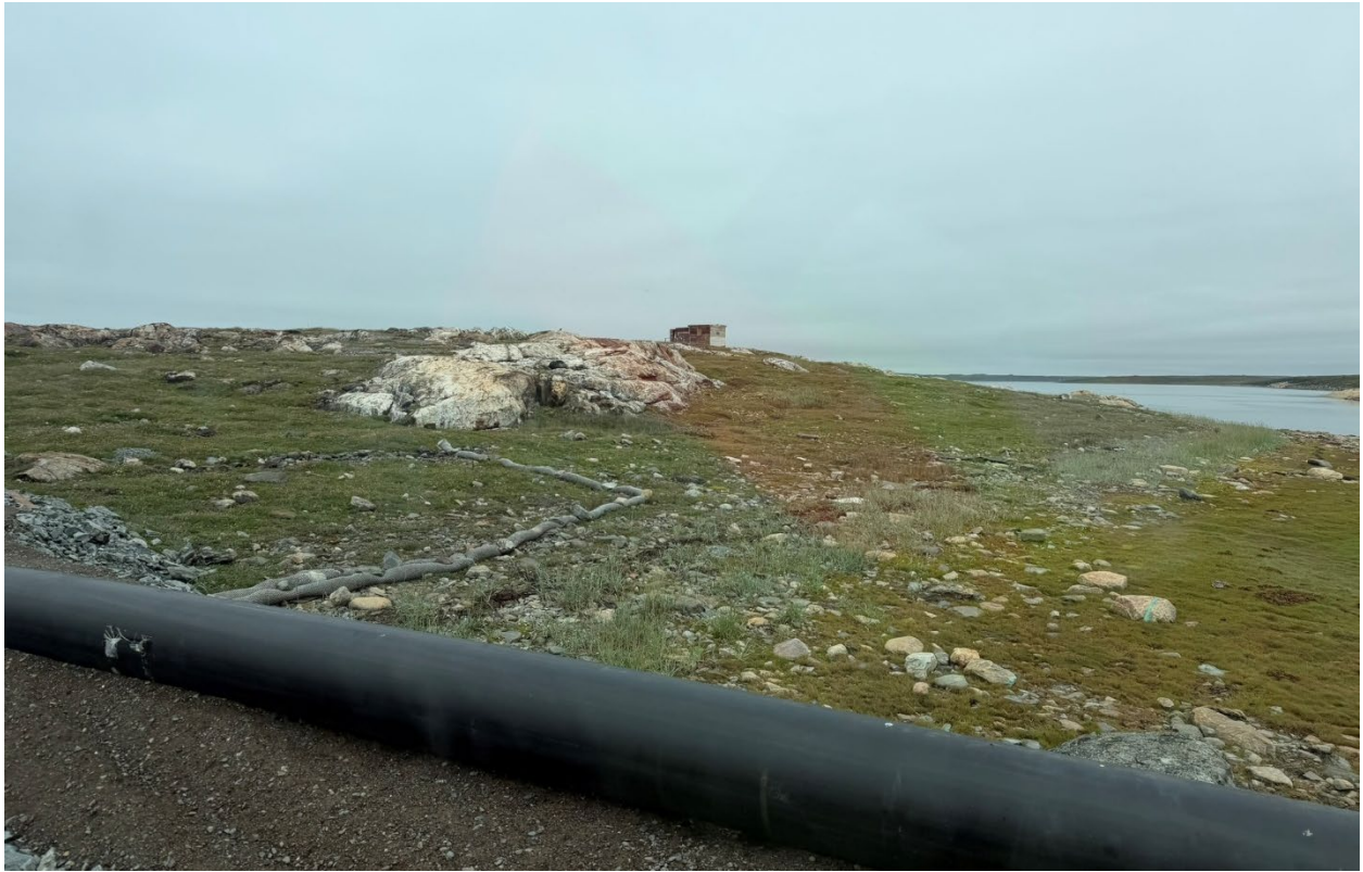
Photo 10: Erosion and sediment controls
