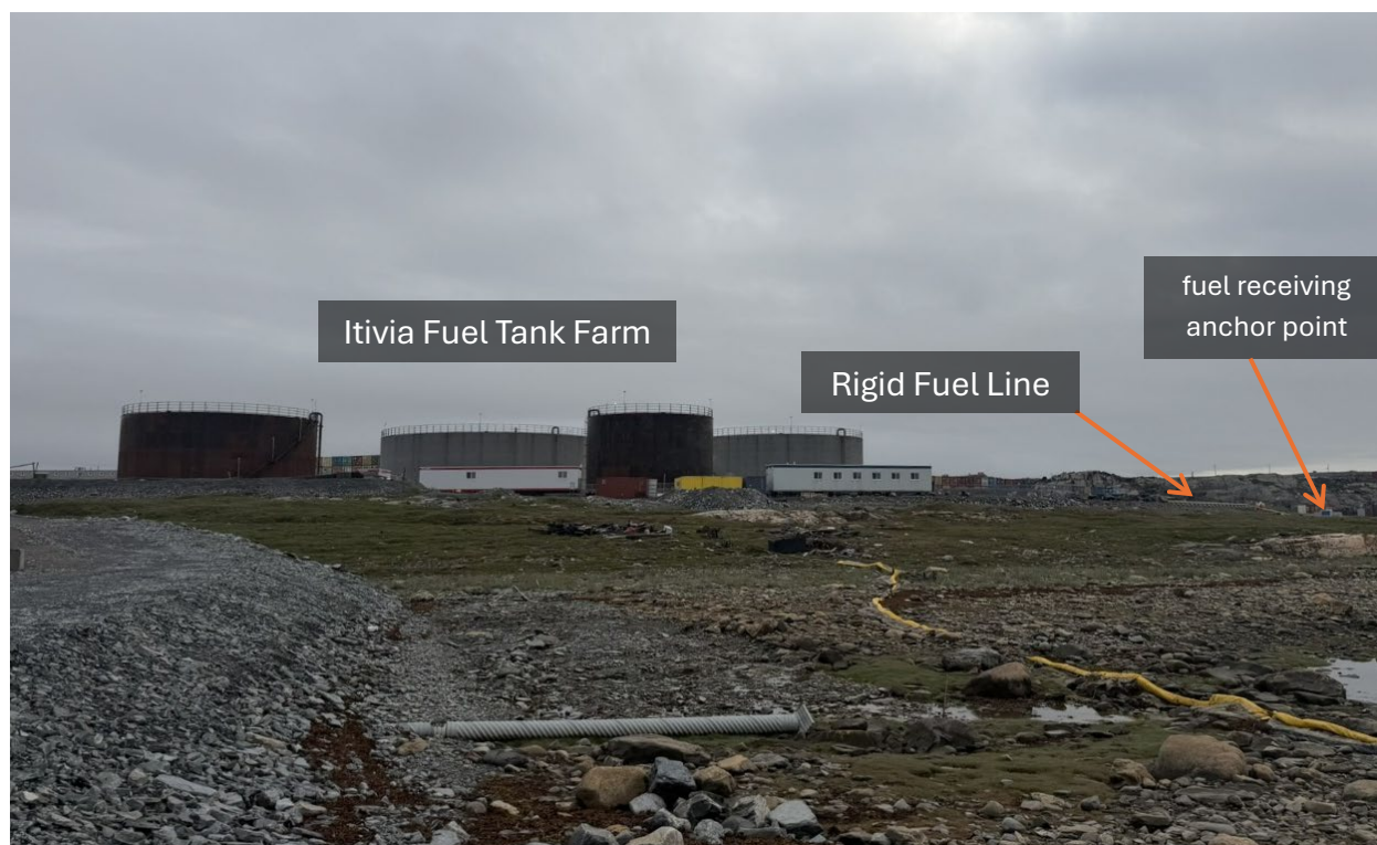
Photo 5: Distant view of the Itivia Fuel Tank Farm, rigid fuel transfer line, and anchor point
