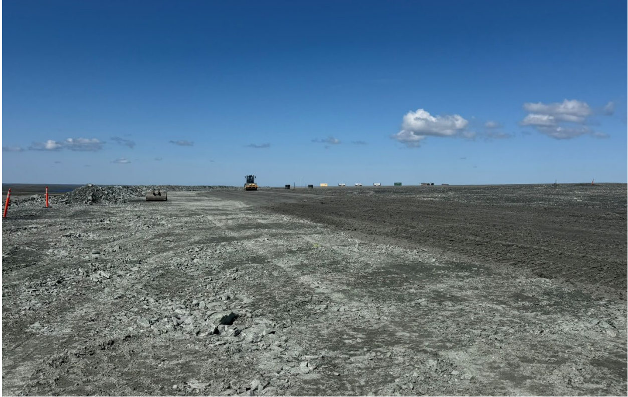
Photo 68: Roller compacting dry tailings
