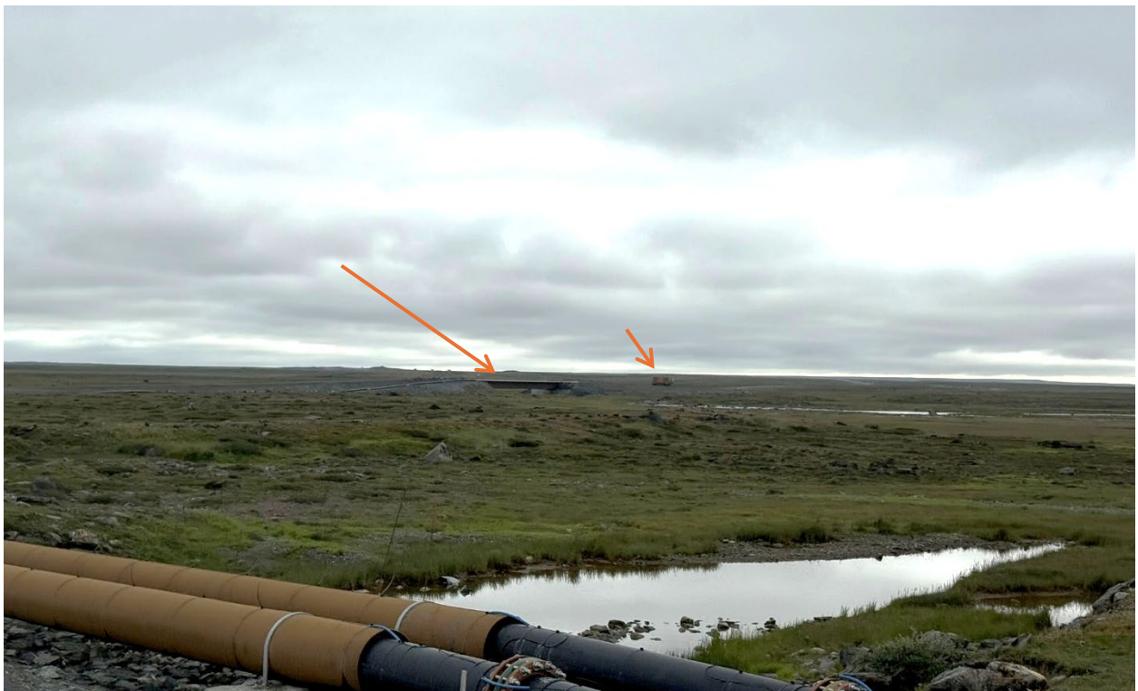
Photo 21: Meliadine River bridge with emergency response sea can located nearby
