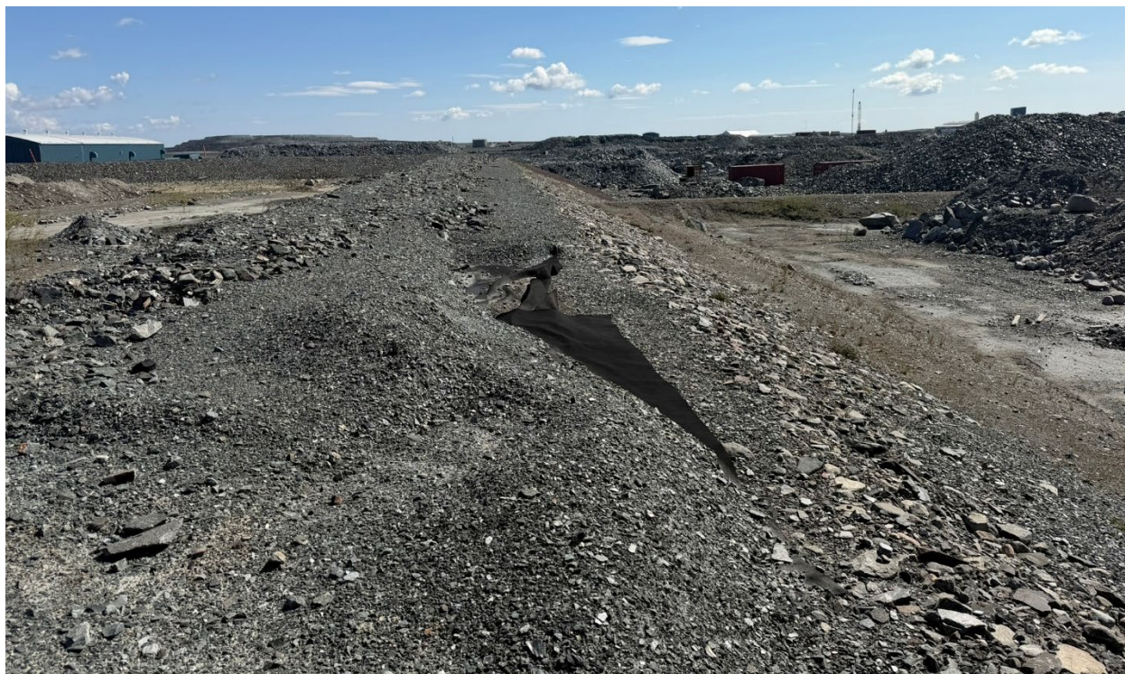
Photo 94: Landfarm cells used for contaminated soil treatment; noted exposed liner
