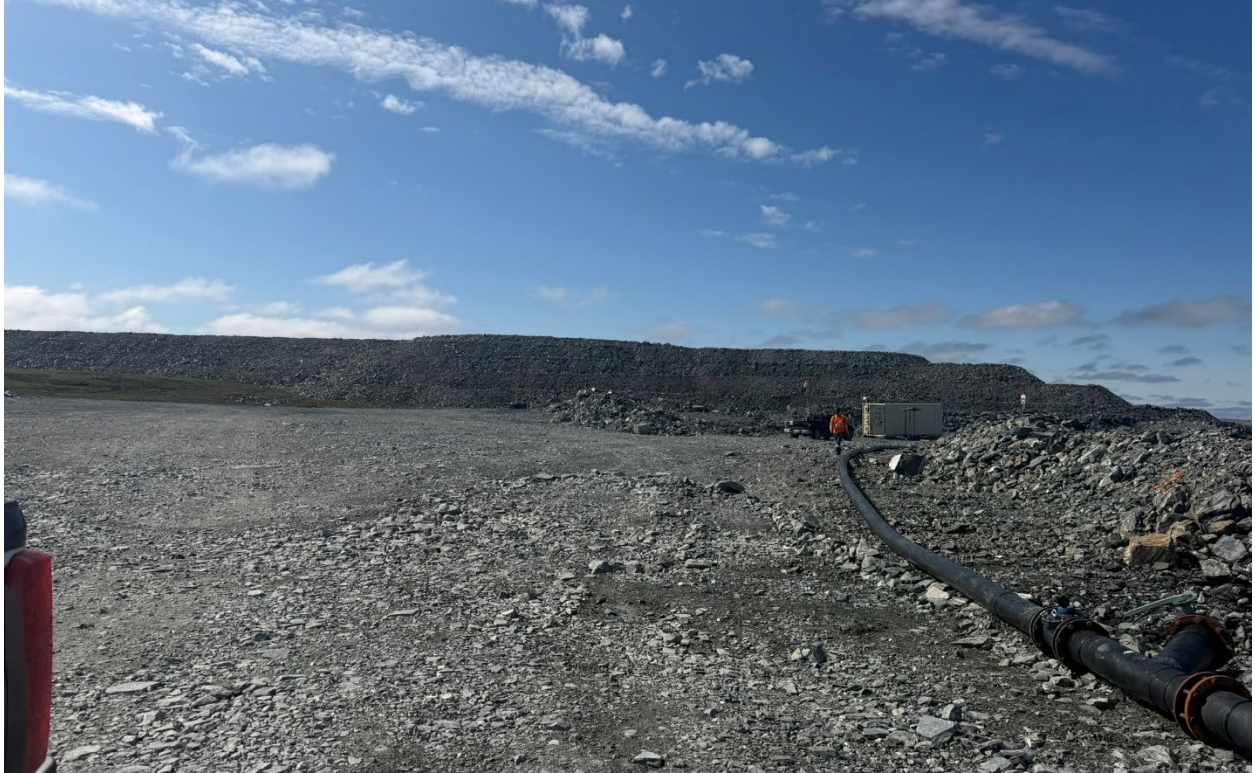
Photo 37: Waste Rock Storage Facility (WRSF) 6
