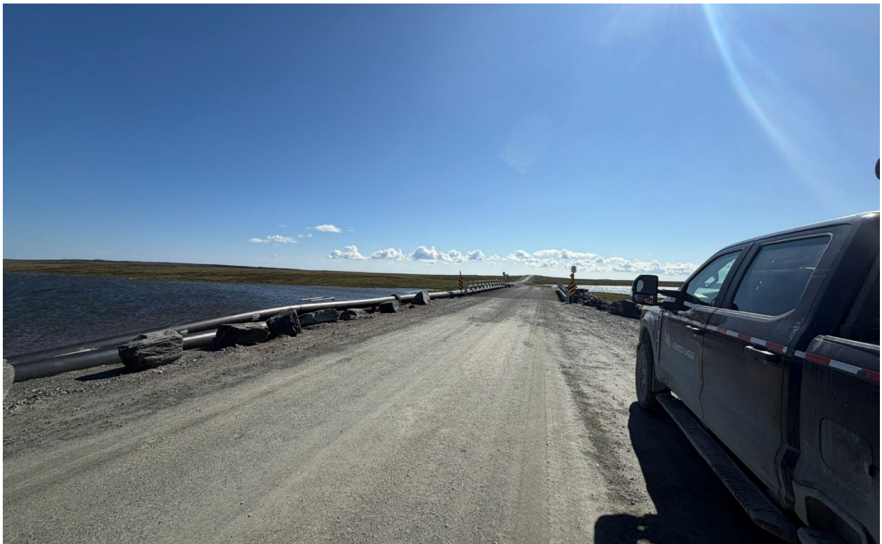
Photo 25: Bridge crossing and exposed waterlines at KM 11
