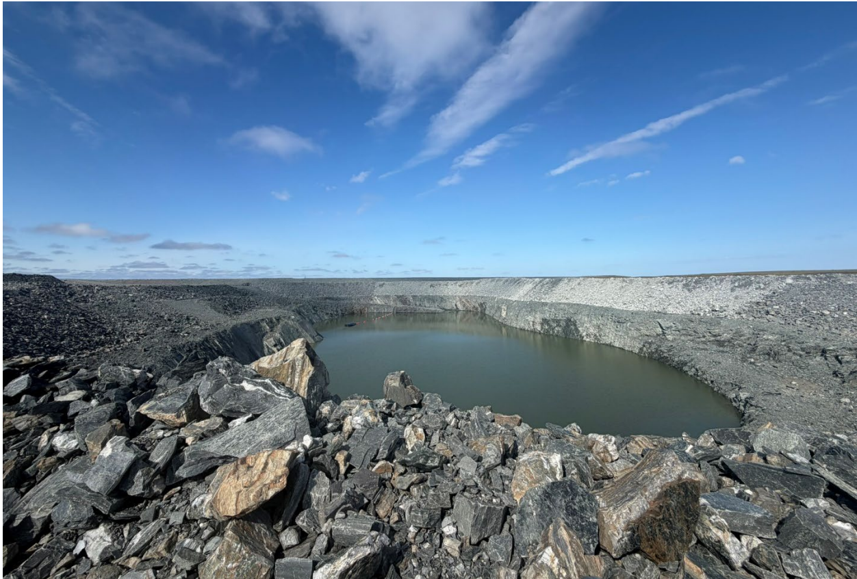
Photo 36: Open pit Pump 01 / CP 9 2
