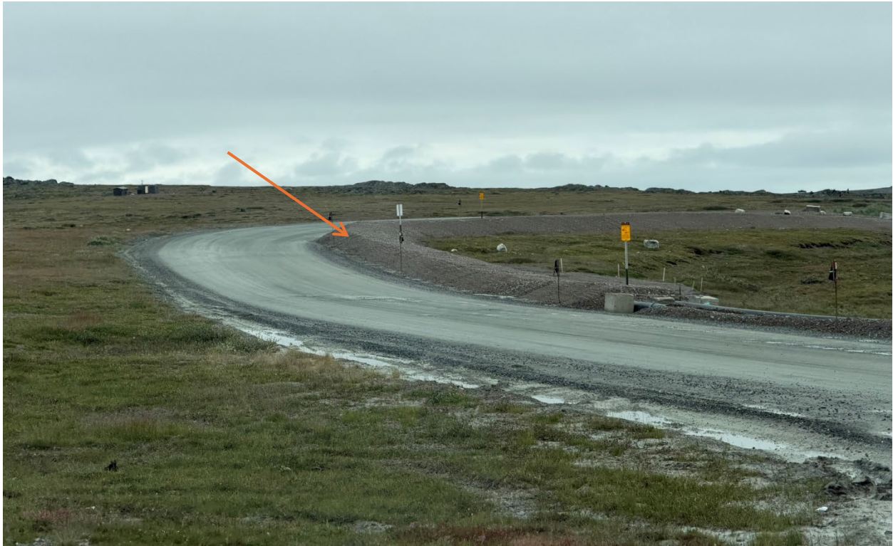
Photo 18: Covered waterline at KM 4.5 with bilingual warning signs
