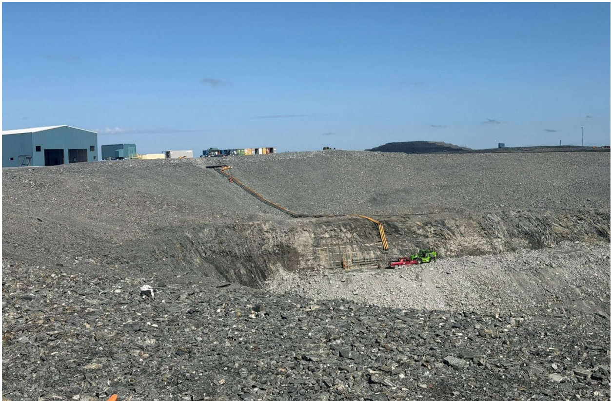
Photo 40: Portal 4, Pump underground portal under development at Pump 02
