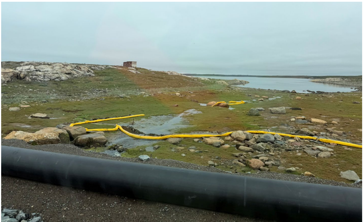
Photo 11: Erosion and sediment controls
