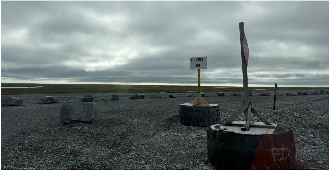
Photo 32: F-Zone Haul Road
