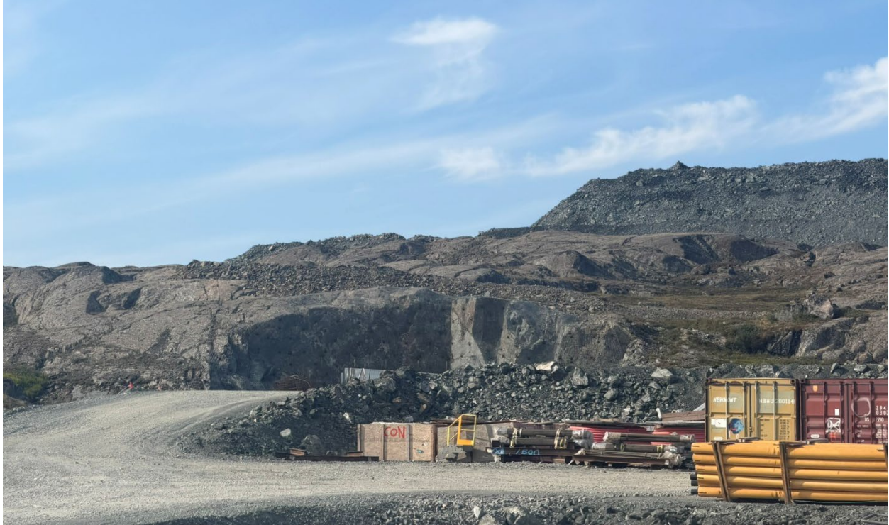
Photo 75: Former Madrid North Portal, which was backfilled in 2025
