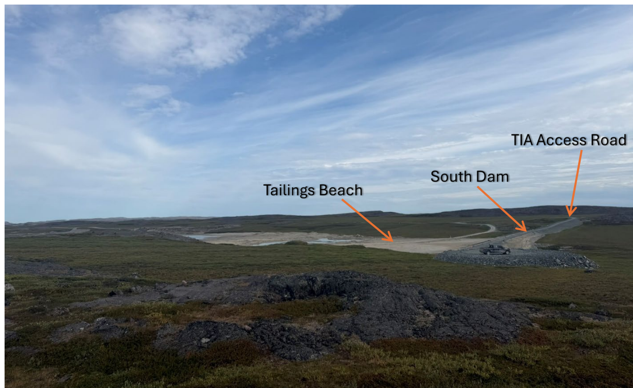
Photo 60: Tailings Impoundment Area – South Dam, distant view facing northeast
