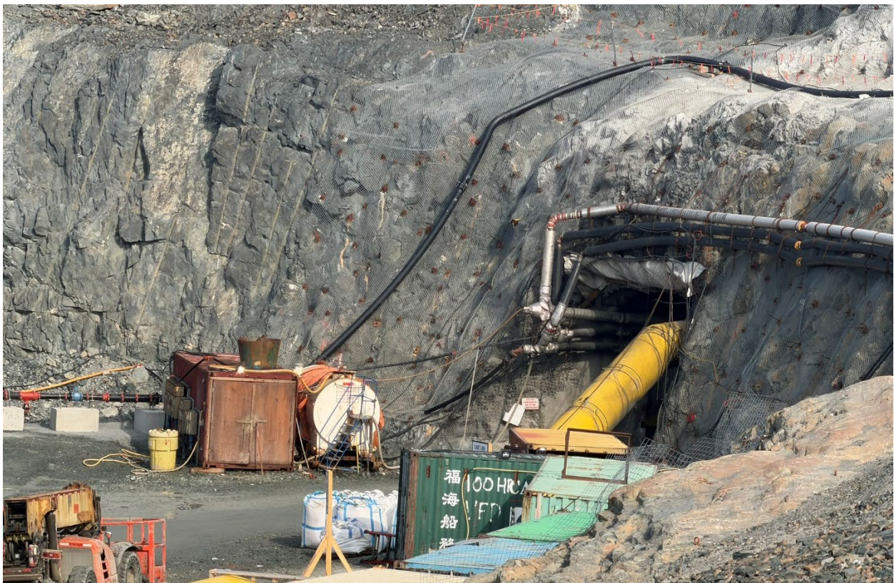
Photo 72: Close up: Underground Portal
