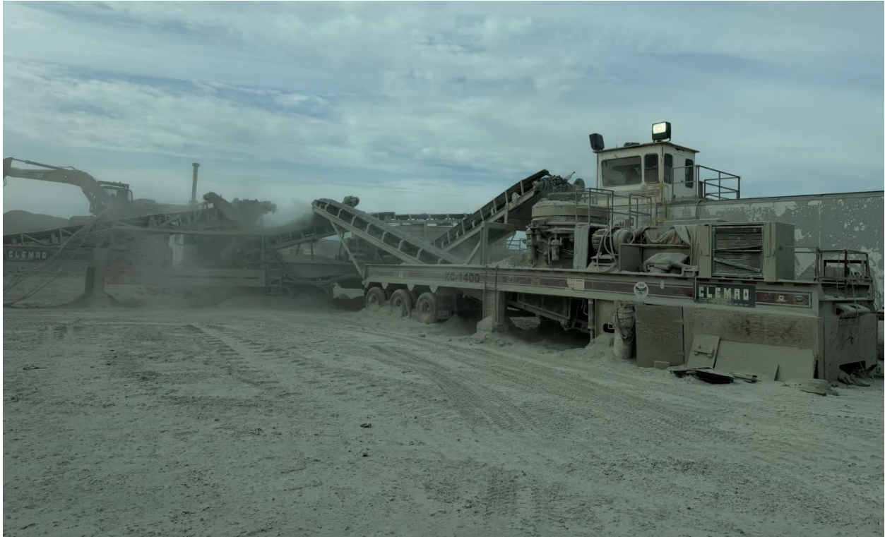
Photo 29: Crusher Pad at Quarry 2
