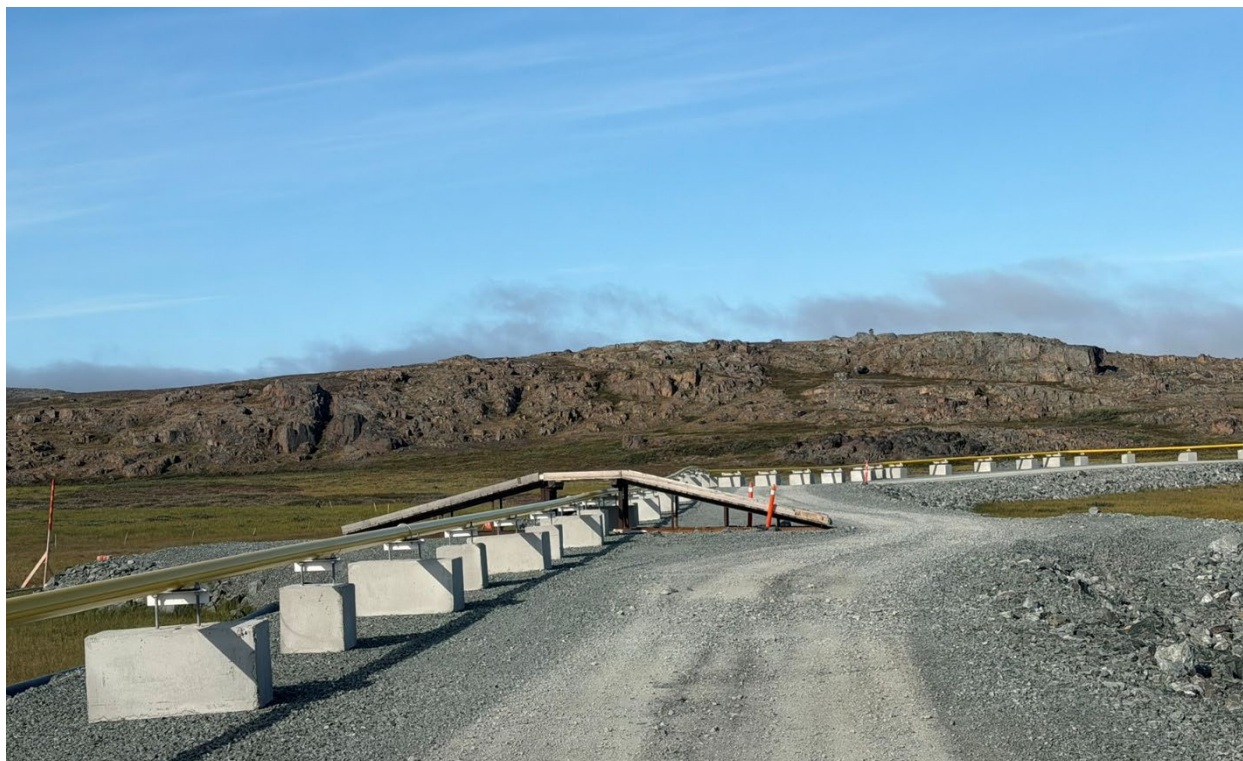
Photo 9: Designated snowmachine crossing over the rigid fuel line 1
