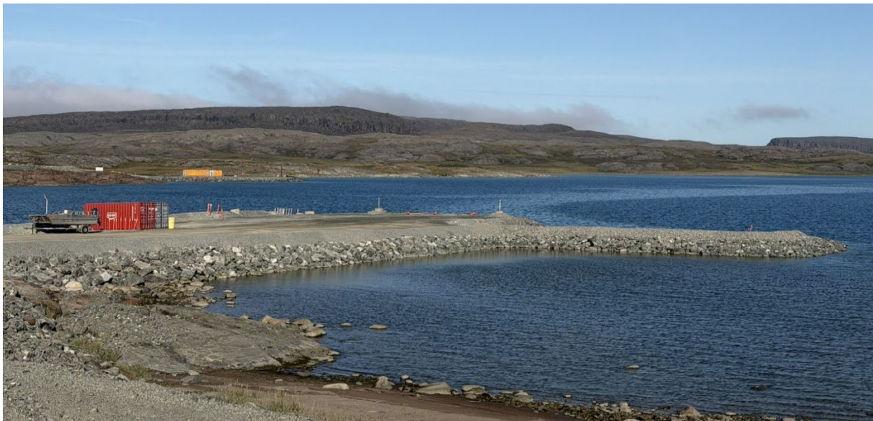
Photo 2: Roberts Bay Jetty, with spill response equipment nearby
