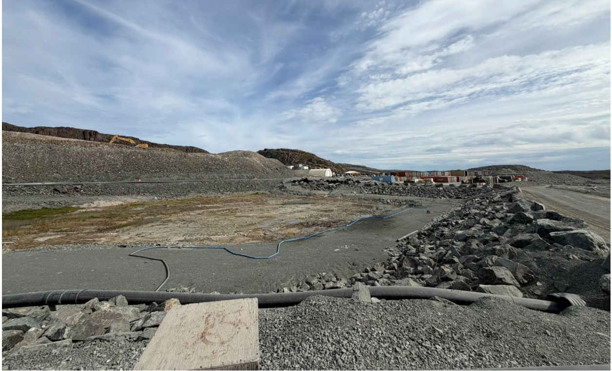
Photo 37: Contact Water Pond
