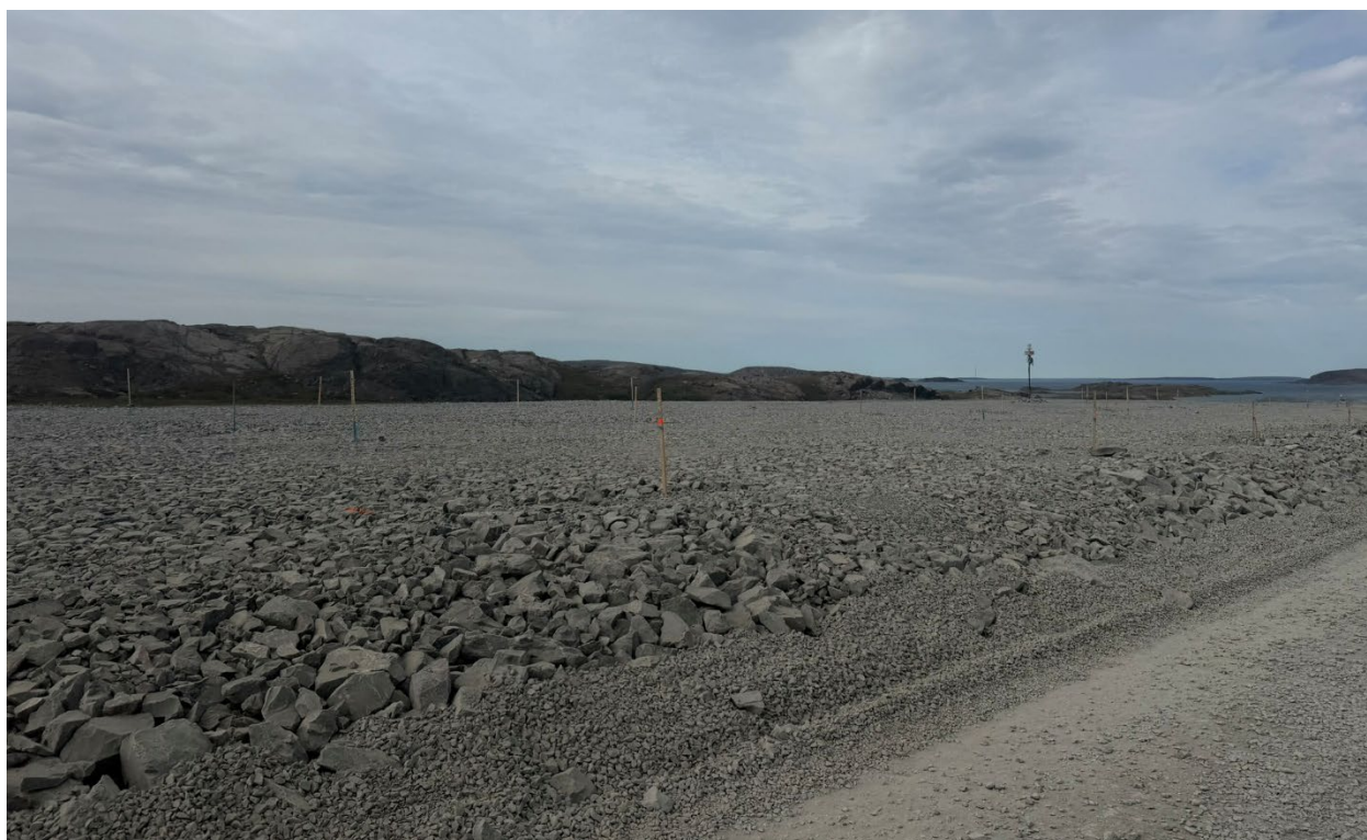
Photo 20: Ongoing construction activities associated with the airstrip extension at the southern toe
