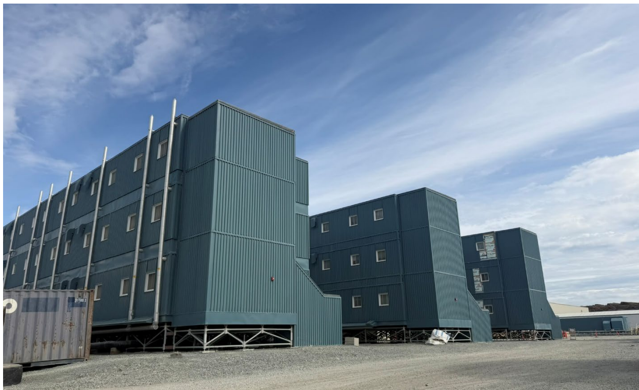
Photo 39: Newly built three-wing, three-storey accommodation complex at Doris Camp, future expansion planned
