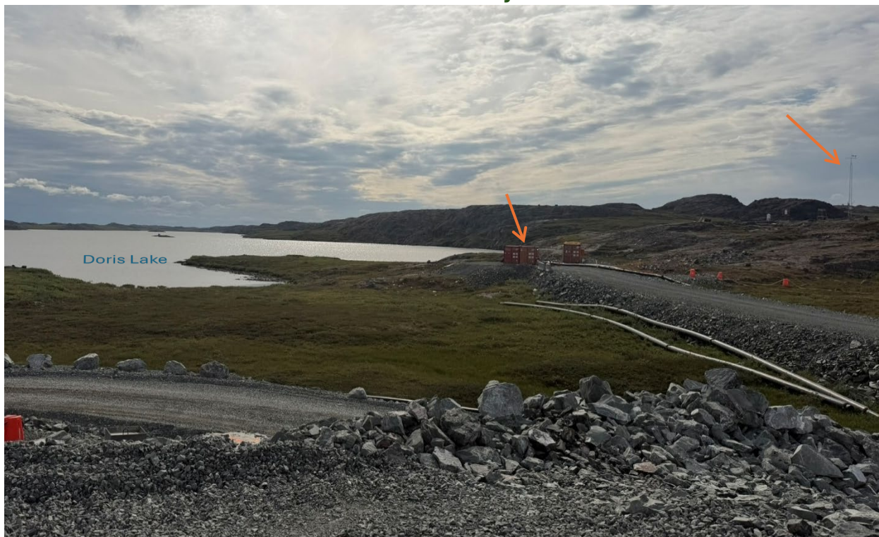
Photo 51: Doris connector vent raise and weather station
