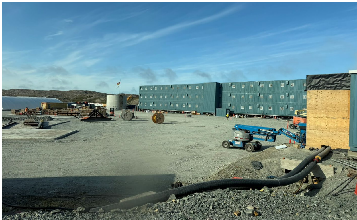
Photo 40: New accommodation complex, facing southwest
