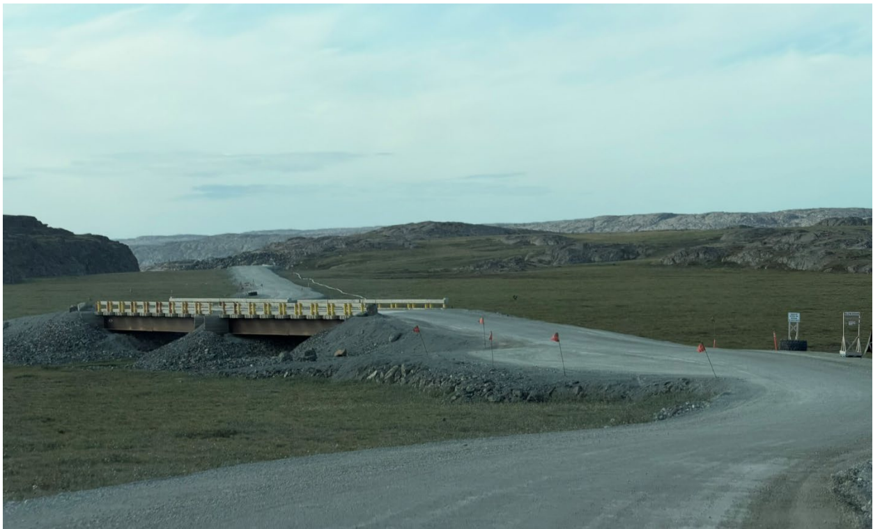
Photo 65: Bridge on Doris-Windy All-Weather Road
