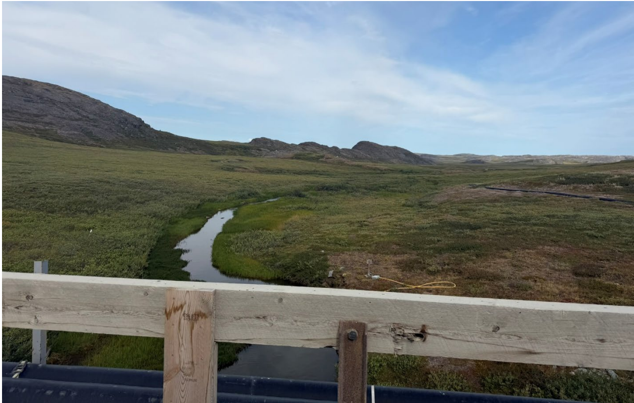
Photo 56: Doris Creek, looking north from Doris Creek Bridge
