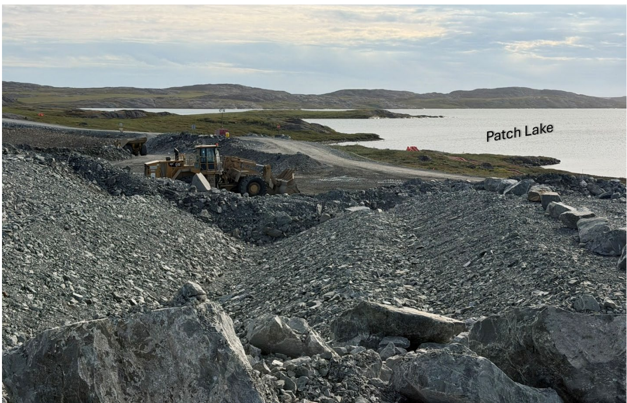
Photo 74: Crown Pillar Recovery Trench (CPRT) and sump
