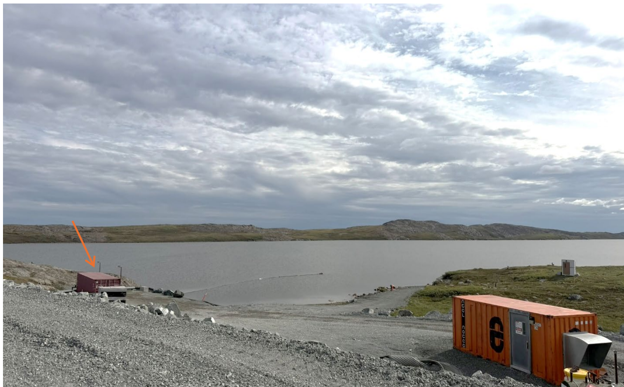
Photo 50: Doris Lake and freshwater intake facility 2
