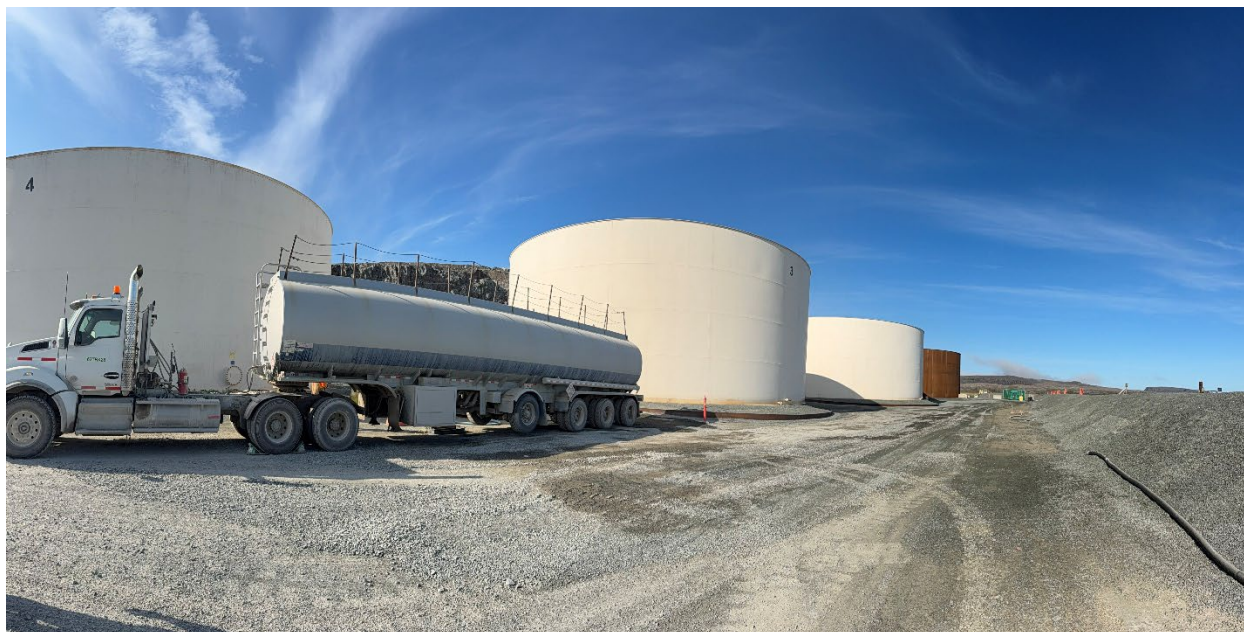
Photo 11: Roberts Bay Multi Tank Farm, within secondary containment
