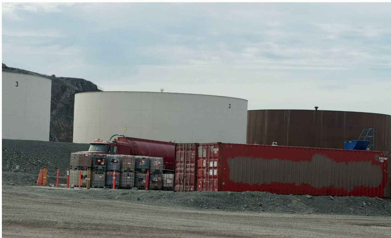
Photo 17: Hazardous-material totes stored adjacent to the Roberts Bay Tank Farm, without proper secondary containment
