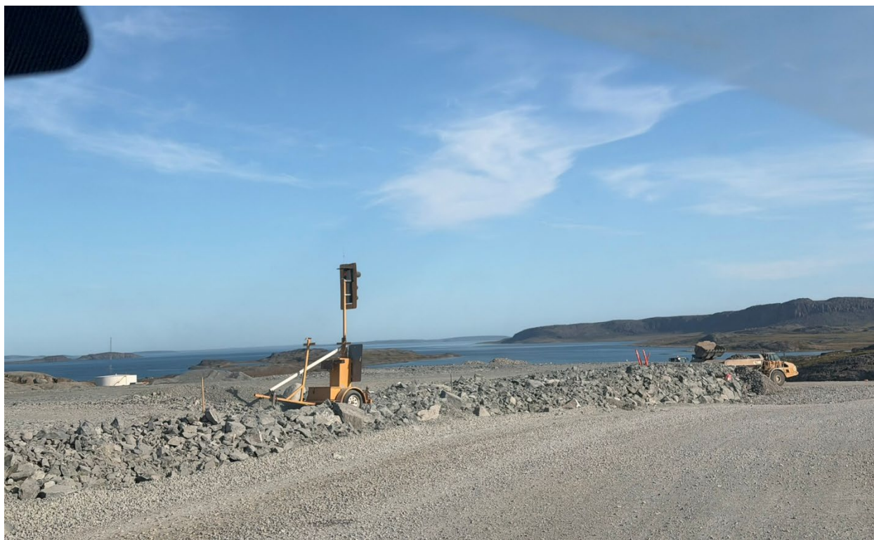
Photo 21: Ongoing construction activities associated with the airstrip extension at the southern toe
