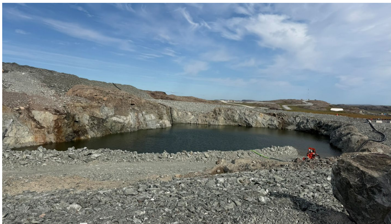
Photo 80: CWP2 Sump - used for collecting leakage from Contact Water Pond 2
