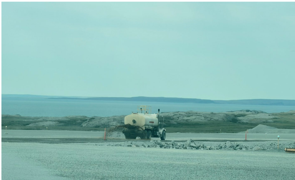
Photo 23: Active dust suppressant being applied on the Primary Road and airstrip
