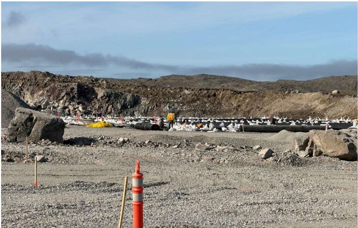
Photo 14: Liner installation at Quarry AF
