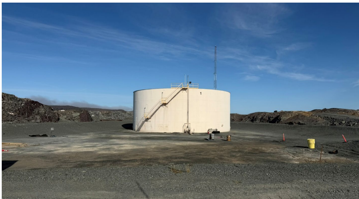
Photo 10: Quarry 1 tank farm, within secondary containment
