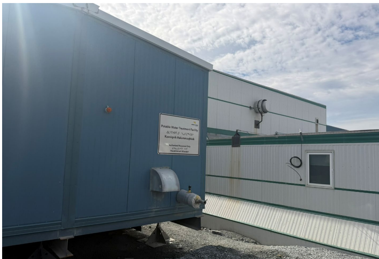
Photo 49: Potable Water Treatment Facility
