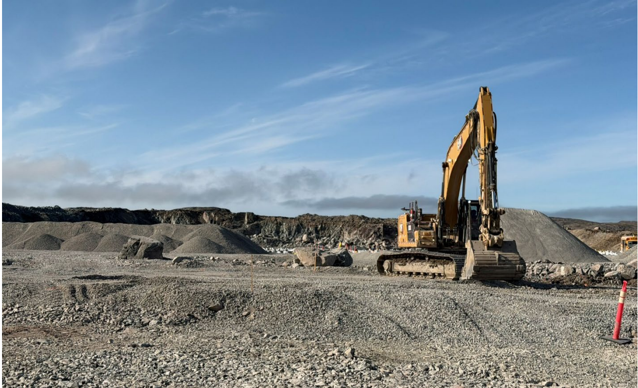
Photo 13: Ongoing earthworks for future tank farm at Quarry AF
